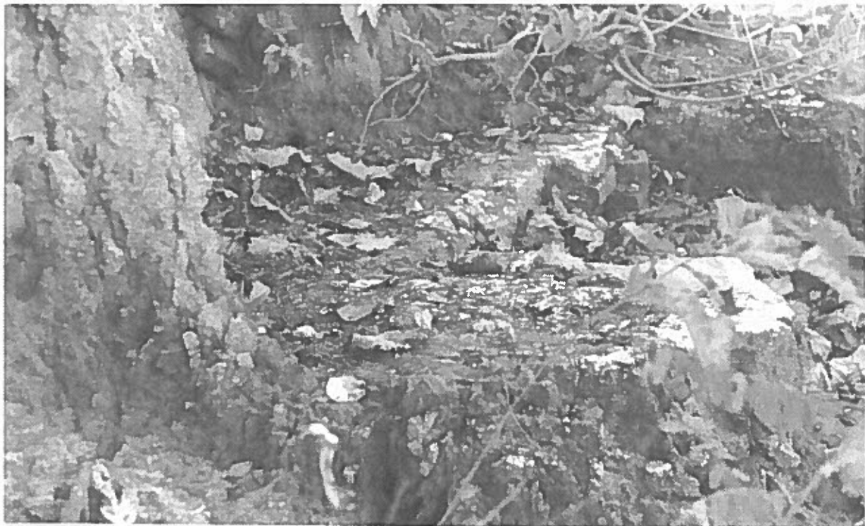
Figure 8. Photograph of the Back Wall and the Rear of the Fire Box at the Lower Rudd Lime Kiln on October 29, 1998 After Several Years of Erosion. Photograph is facing southwest.
