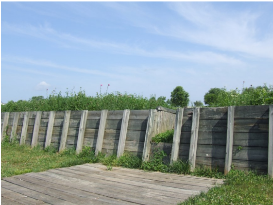
Earthworks at Camp Nelson, Jessamine County, KY
