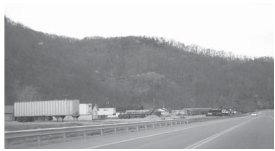
Highway 15 in Perry County is an example of a WPA era road that has lost its integrity of design, and is no longer eligible for the National Register. The original alignment, an important element of design, no longer exists. As a result, the road does not read as a New Deal resource. Photo taken in 2004.
