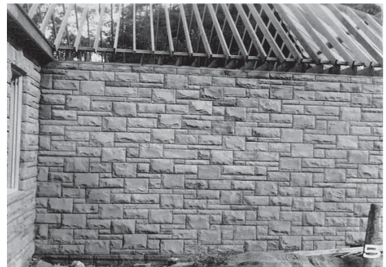
Representative stone work on WPA schools in Greenup County. Fullerton School, circa 1939. (GP Collection).
