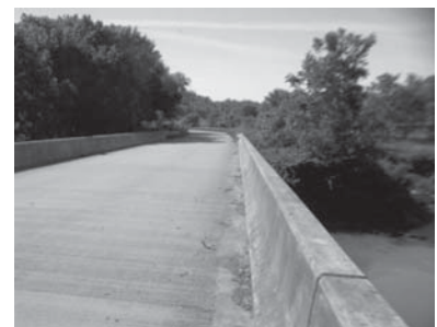
Kehoe Road Bridge (Boyd Co.), 2004.
