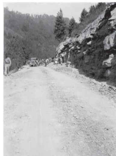
“Constructing Blackey Road.” Photo date unknown. (GP Collection).
