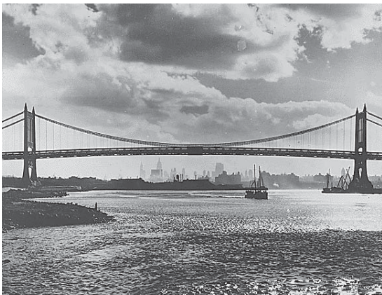
The Tri-borough Bridge in New York City was a PWA project. Photo date unknown. (FDR Library).
