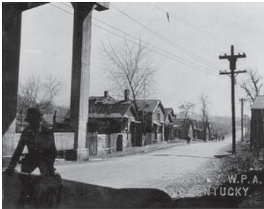
Example of “substandard” housing in Lexington, KY. Photo date unknown. (GP Collection).
