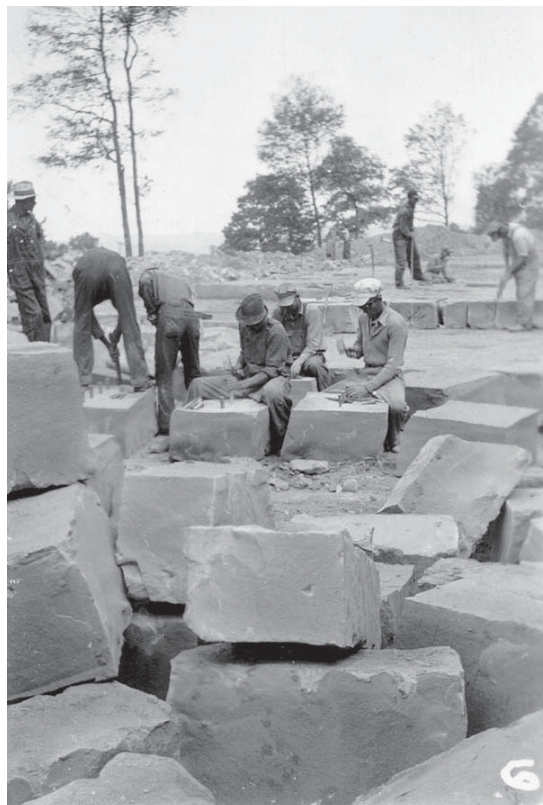
"Shaping stones for Greenup Courthouse." Photo taken circa 1938. (GP Collection).
