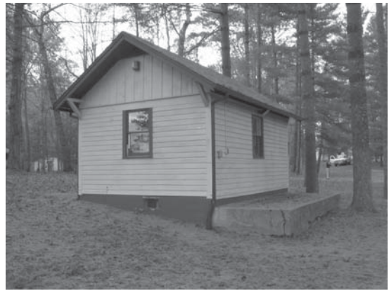
Bald Rock CCC building, known as the “Sheet Shack.” Photo taken in 2004.
