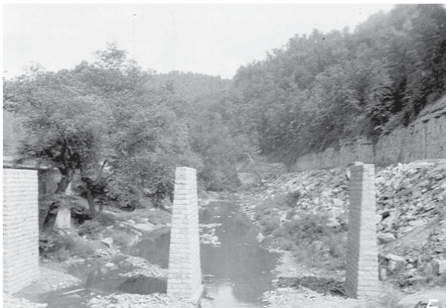
Ulvah Bridge stone piers. Photo date unknown. (GP Collection).
