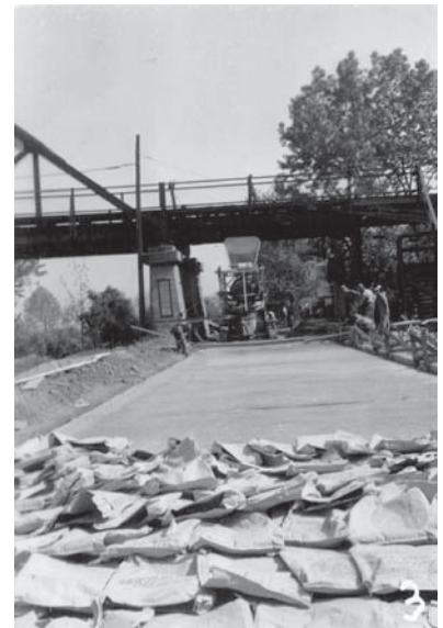
Concrete Street Construction in Russell (Greenup Co.). Photo date unknown. (GP Collection).
