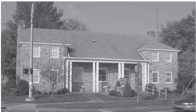
J. Albert Bagby Memorial Park Community Building, Grayson (Carter Co.). Constructed by the NYA in 1941. Photo taken in 2004.
