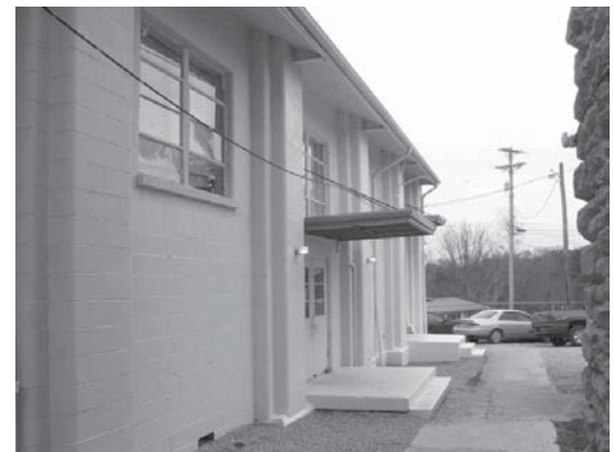
Whitley City School. Structure believed to be the NYA Cannery building. Photo taken in 2004.
