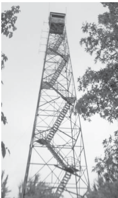
Stearns Fire Tower (McCreary Co.), 2004.
