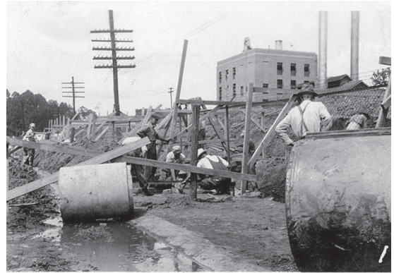
“Corbin sewers under construction by the WPA, 1940.” (GP Collection).
