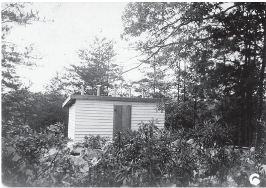
An example of a sanitary privy constructed by WPA labor in McCreary County (KY). Photo date unknown. (GP Collection).
