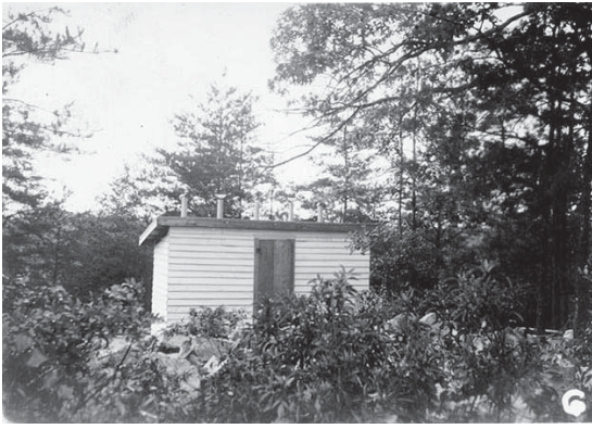
Wooden privy constructed by the WPA county sanitation project. Photo date unknown. (GP Collection).
