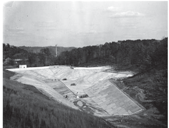
Boyd County Sediment Basin, 1939. (GP Collection).
