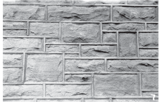
WPA stonework. Date and location unknown. (GP Collection).
