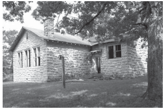
Hollyhill School building, 2004.
