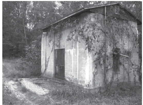
Sediment Basin Pump House, 2004.
