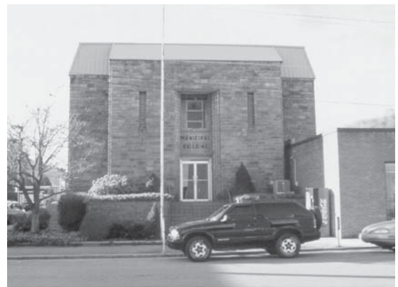
Pineville City Hall, constructed by the NYA in 1941. Photo taken in 2004.
