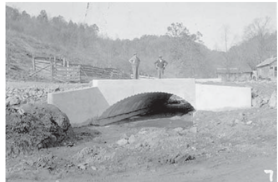
"Steel arch on Garner Road built by the WPA." (Boyd Co.). Photo date unknown. (GP Collection).
