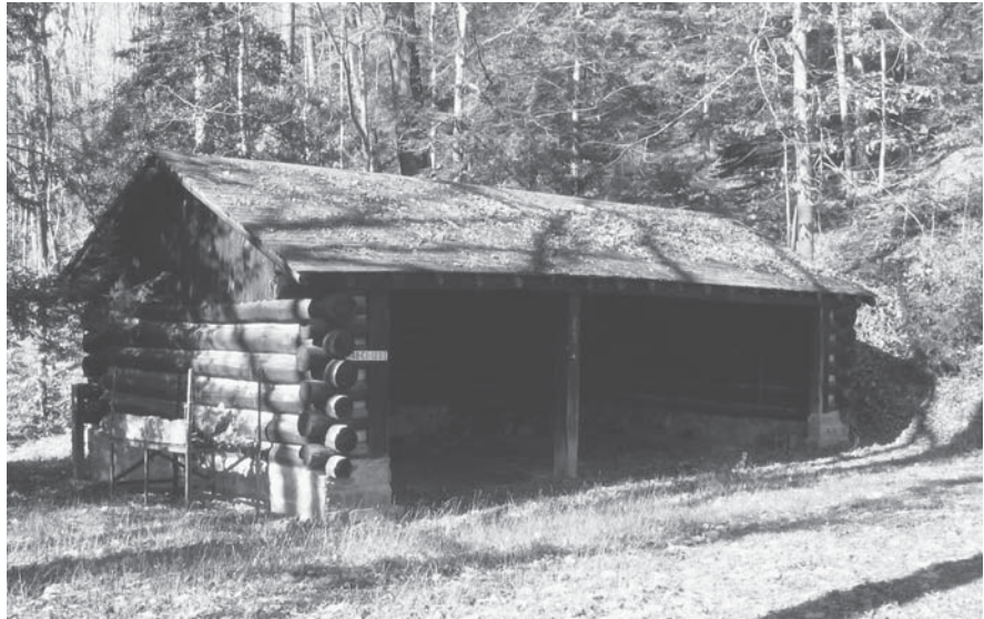
Putney double bay garage, Building C. Photo taken in 2004
