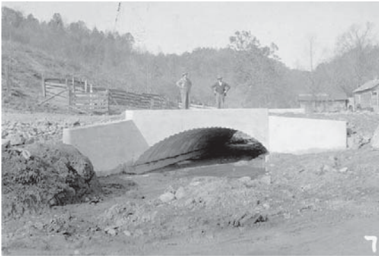
WPA Culvert in Boyd County. Photo date unknown. (GP Collection).
