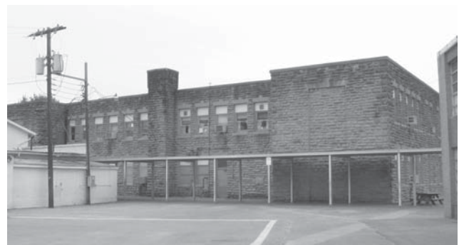
Whitley City School, rear façade. Photo taken in 2004.
