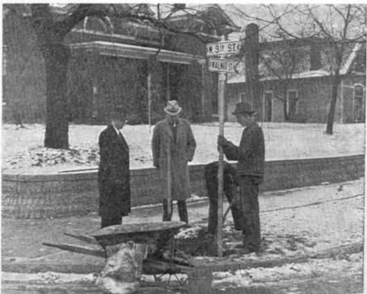
Mayor Fred Weir of Owensboro and NYA Supervisor Terry Coleman look on as NYA workers place street markers. The markers are being set in concrete.
