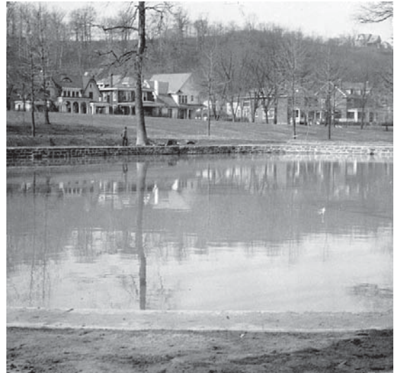
"This view shows the Central Park Pool, constructed with native sandstone and finished with a cement cap. Photographed March 25, 1936." (Boyd Co.). (GP Collection).
