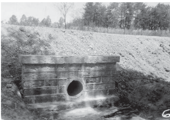
"Culvert constructed by the WPA." Photo date unknown. (GP Collection).
