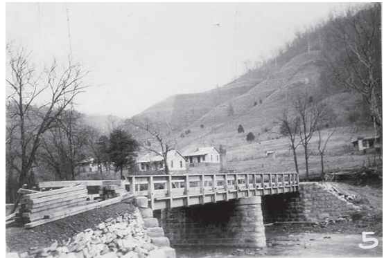
Roxana Road Bridge. Photo date unknown. (GP Collection).
