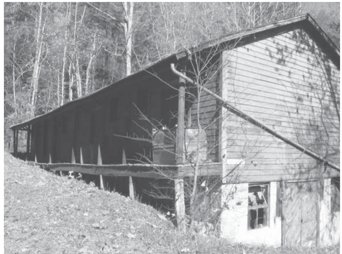
Putney "Tool Warehouse," Building E. Photo taken in 2004.
