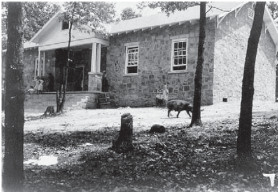
“Silerville School constructed by the WPA under a blanket project.” Photo date unknown. (GP Collection).
