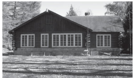
Putney Ranger Station, west façade, 2004.
