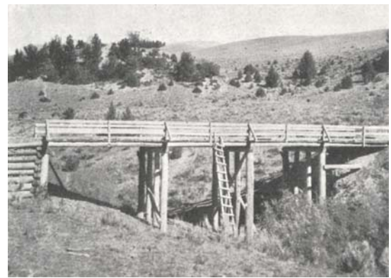
CCC truck trail bridge. Photo date unknown. (Kylie 1937, CCC Forestry).
