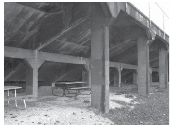
Superstructure of Putnam Stadium, 2004.
