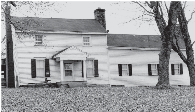
Figure 4: Hall/Parlor Log House, Collom/Owen House, Near Winchester, Clark County. The original house is the two story section to the left, constructed by 1812, with a hall/parlor plan. The single story log wing to the right was added sometime later. The weatherboards and front porch may also be later renovations
