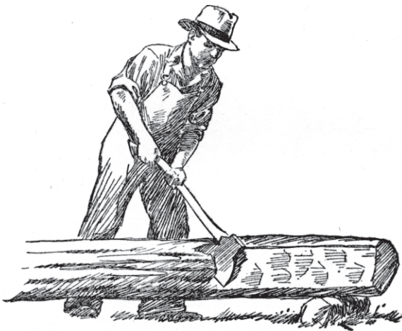
Worker hewing a log for a “modern” cabin. Illustration from Popular Science’s, How to Build Cabins, Lodges, & Bungalows, 1946.
