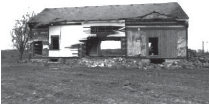
Figure 7: Dogtrot House Type, Sullivan House, Franklin County. This house was constructed Circa 1810, and had an exposed log exterior. The central passage, or “dogtrot” was not open as seen here, but had doors framed in and was enclosed with siding. The south facade, shown here, was originally the front of the house. Around 1830, the house was extensively remodeled - the interior was plastered, new trim was added in the hall, an addition was added to the south facade, the exterior was sided, and the old front of the house became the back of the house. Some of this renovation was apparently planned in the original construction, as some of the interior spaces seem to have been left unfinished until the 1830’s period
