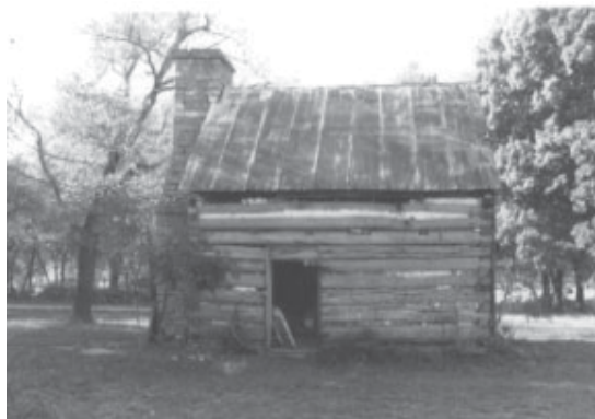
Figure 3: Cook's Cabin, Early 19th century, Franklin County. Cook's Cabin would most likely have been considered a "house" when it was built, although from today's perspective it looks like a cabin. It is an unusual survival of a relatively unaltered single pen log structure that may have originally been a kitchen
