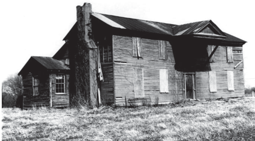
Figure 8: Watwood House, Log Center-passage I-House, Ballard County, Circa 1850. By the middle of the nineteenth century, log building had evolved to the point where the construction method could be almost entirely hidden. This log house has much the same appearance as frame houses of the same era. The exterior was weatherboarded, and inside walls were plastered downstairs and covered with beaded boards upstairs so that all evidence of log construction was entirely hidden from view. The logs and furring strips are exposed where the siding has come off to the right of the chimney.
