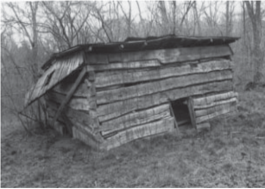
Figure 2: Single-Pen Log Cabin, Bullitt County, Circa 1830-1850. This single pen cabin was one and a half-stories tall with a loft room and a large fireplace at one end. It has three doors, but no windows. At one time there were lean-to shed additions to the left and at the back. The foundation and two or three logs have rotted into the ground. The cabin was still
