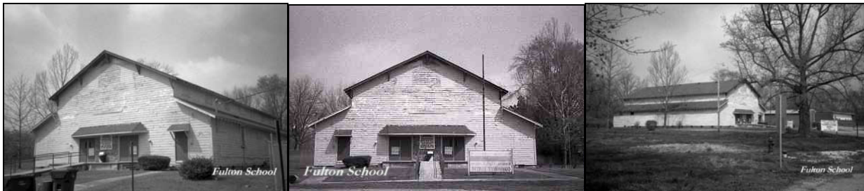
Fulton School Auditorium/Gymnasium
