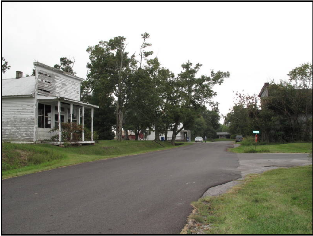
Figure 2. 13 Looking southwest down Main Street in Hampton, LV-91 on left.
