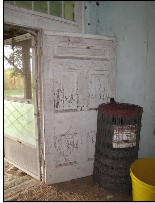
Figure 6. 13 Detail of five-panel door, LV-81.
