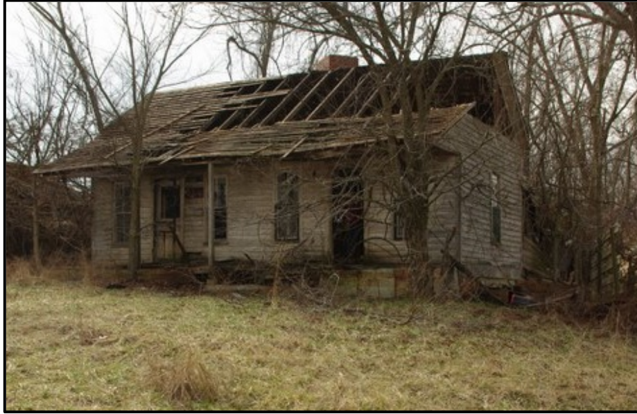
Figure 6. 27 Façade of CN-30, a two-room house with diagonal brick stack.
