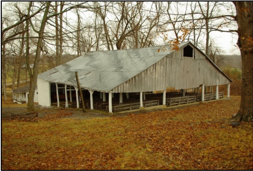
Figure 5. 39 Circa 1920 open –air shed at Hurricane Camp (CN-25).
