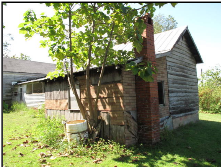
Figure 4. 9 Rear of the meathouse at CN-77, showing brick flue on addition.
