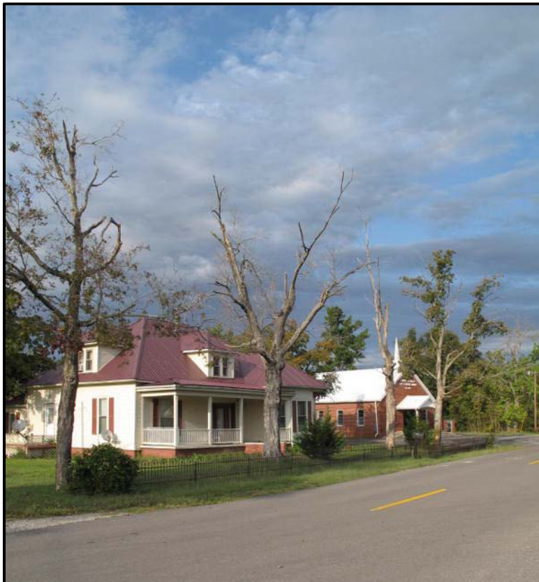
Figure 2. 20 Looking northeast on State Route70 in Tiline, LV-95 and LV-94 on left.
