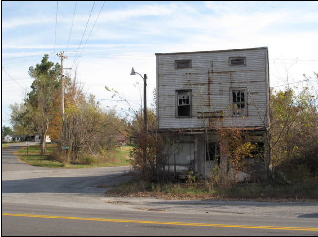
Figure 5. 14 Tribble Store (LV-103) in Burna
