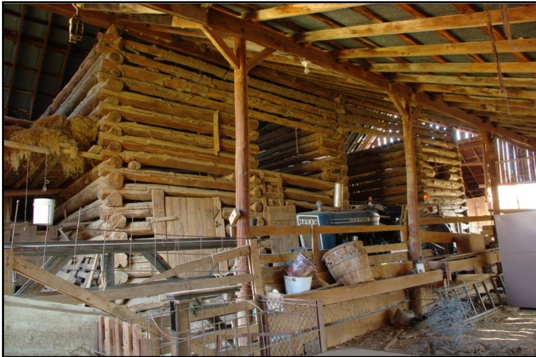
Figure 3. 6 Interior of barn, showing the two cribs (LV-42), facing northeast.
