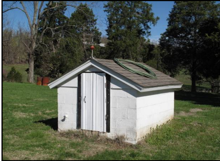
Figure 4. 34 Concrete block pump house at LV-51.
