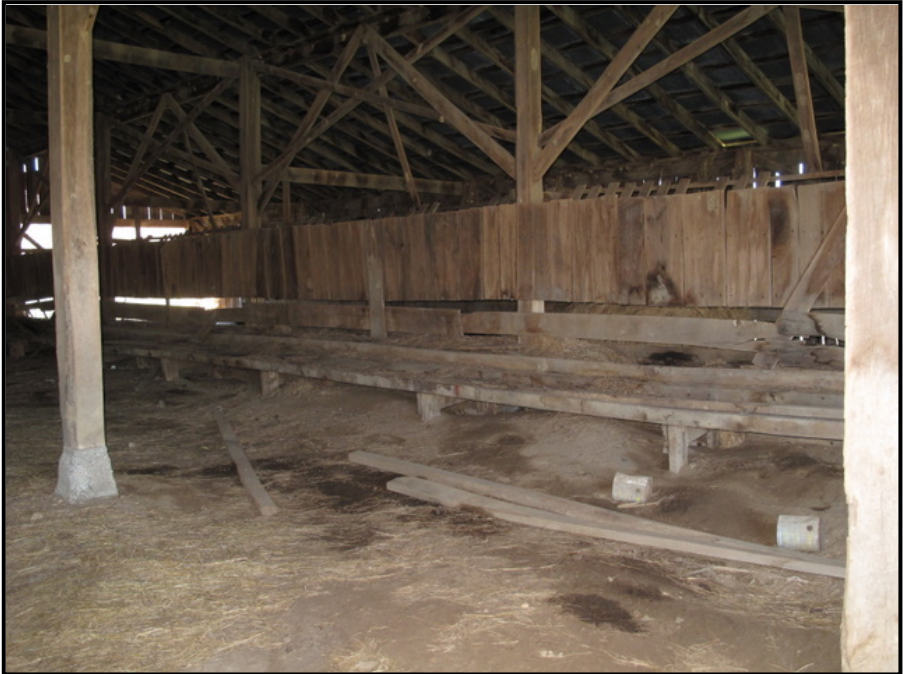
Figure 3. 40 The silage track at CN-31 ran around the barn to this trough, which has hay racks mounted on the other side.
