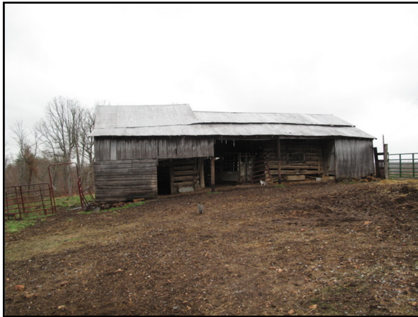
Figure 3. 19 Log barn (CN-67) at the Underdown Farm in Crittenden County.
