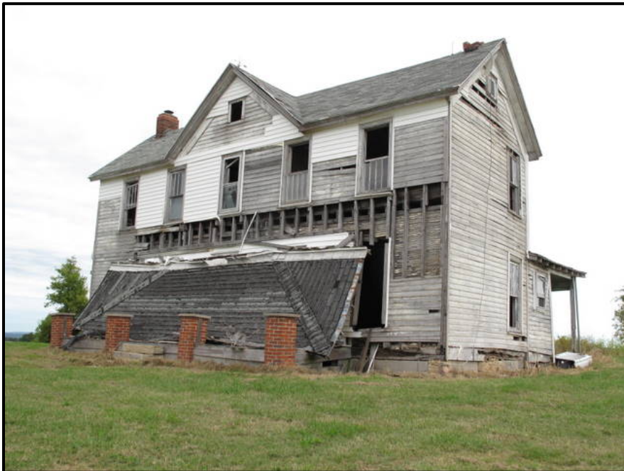
Figure 6. 39 Ray House, LV-79, a two-story central cross gable Gothic Revival.
