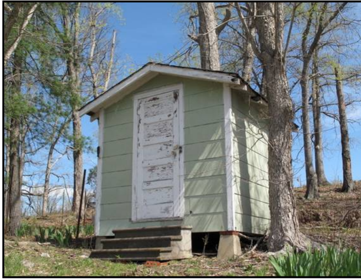
Figure 4. 4 Meathouse on concrete piers, LV-54.
