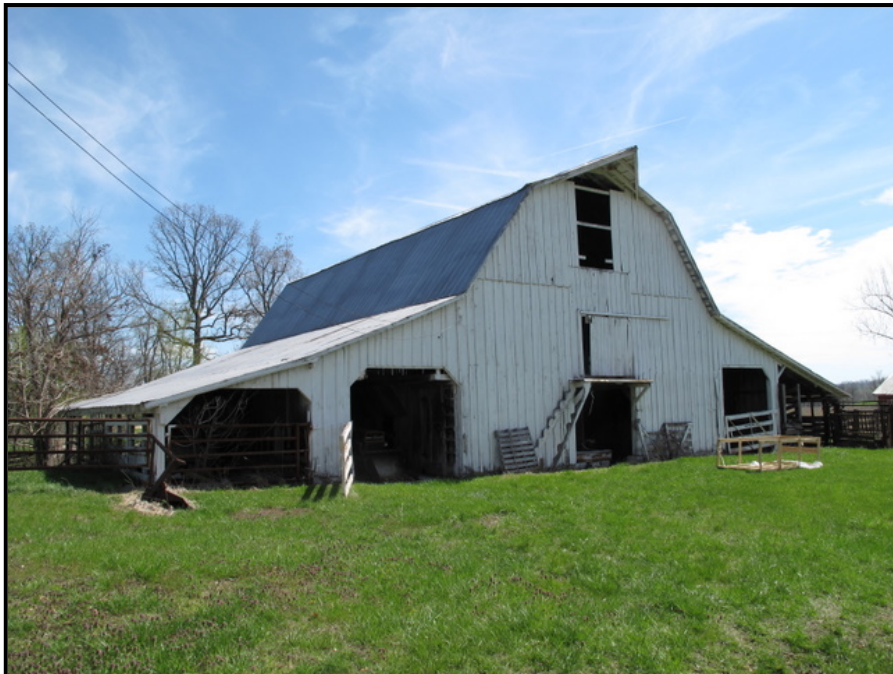
Figure 3. 28 LV-54, multi-purpose barn outside of Lola, Livingston County.
