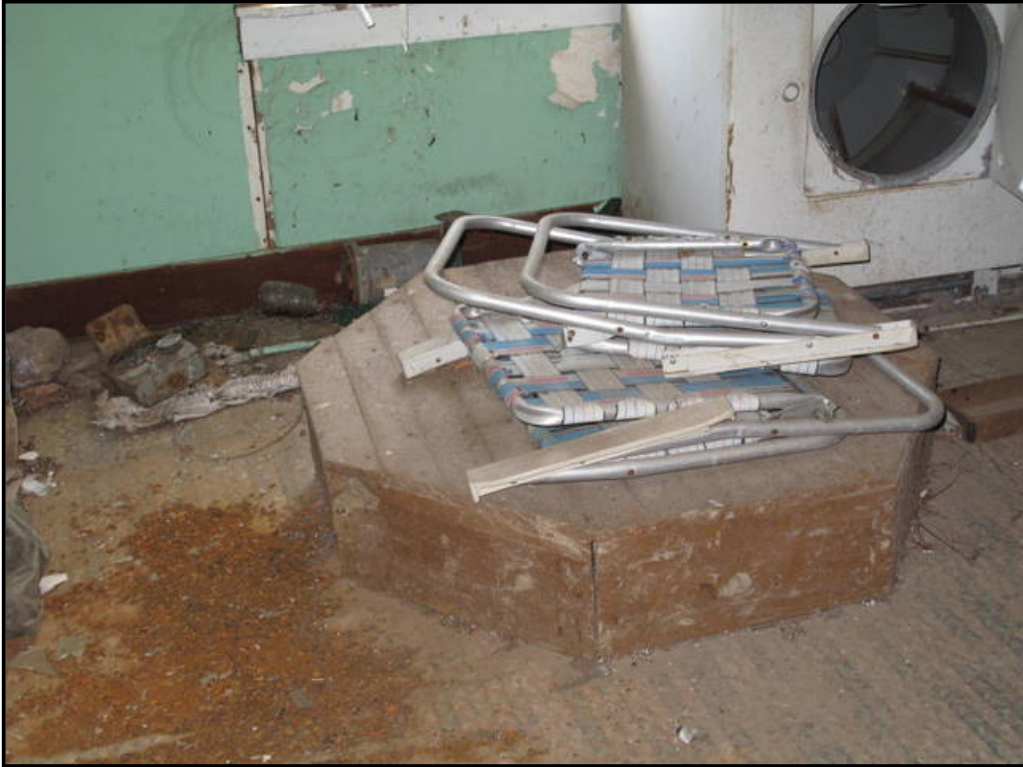
Figure 4. 32 Cistern on enclosed porch at LV-62.
