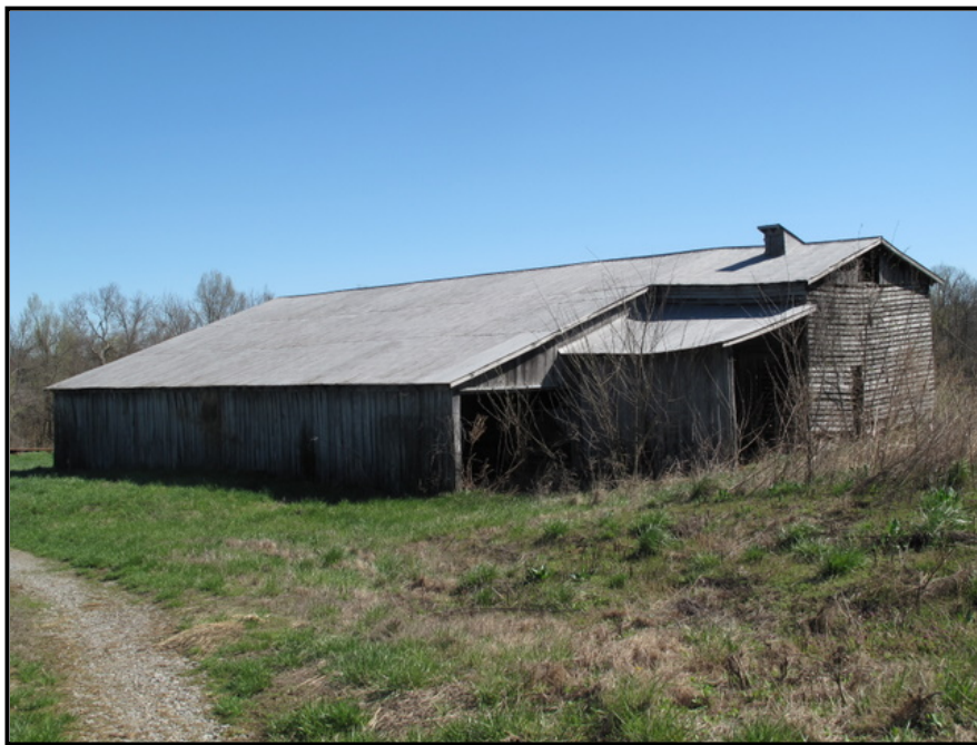
Figure 3. 35 Silage/stock barn, showing exterior corn crib, CN-31, Crittenden County.
