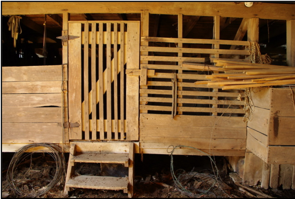
Figure 3. 66 Tack room at CN-41. Steps in tack room lead to loft.
