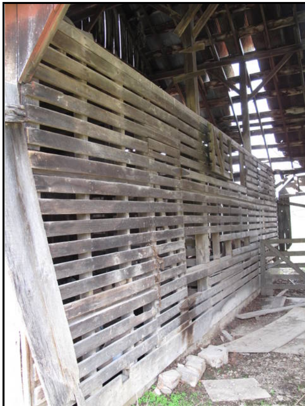
Figure 3. 44 View of the interior corner crib at LV-68.
