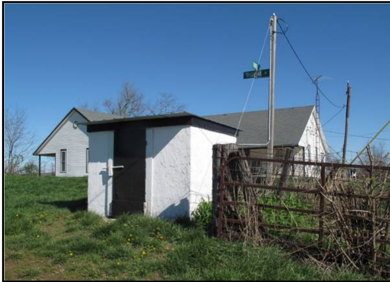
Figure 4. 35 Concrete pump house at CN-31.
