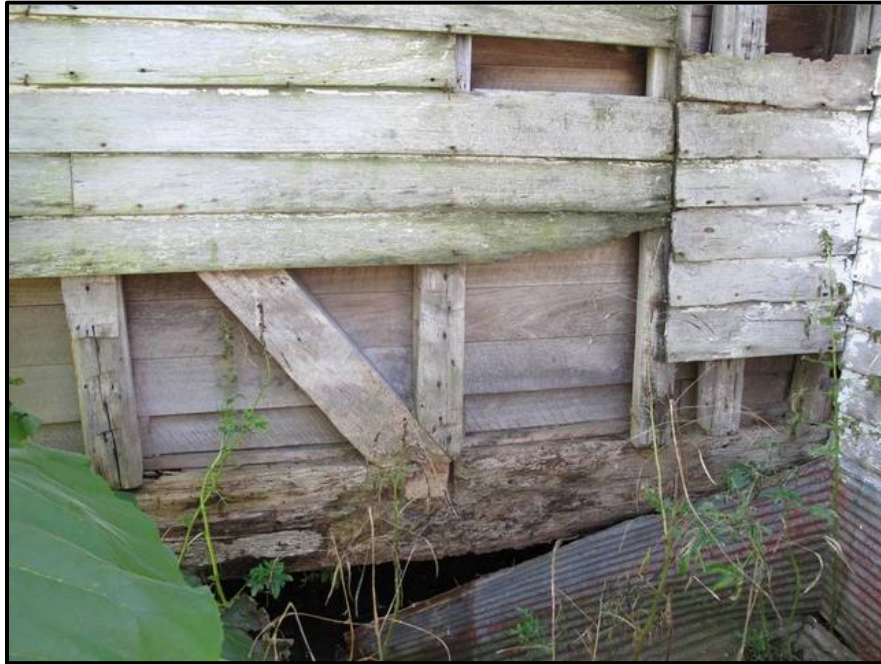
Figure 6. 26 Detail of framing of CN-77 on rear elevation.
