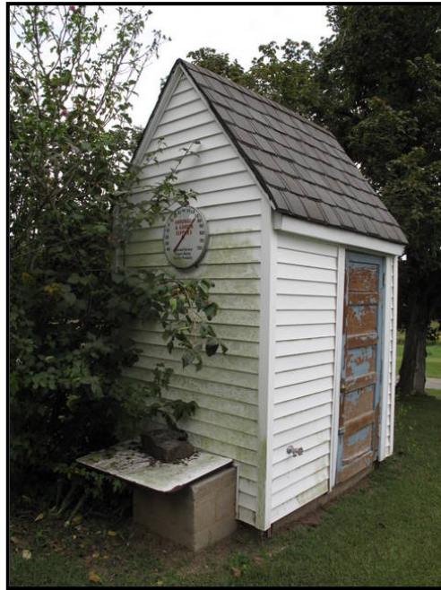
Figure 4. 36 Frame pump house at LV-87.
