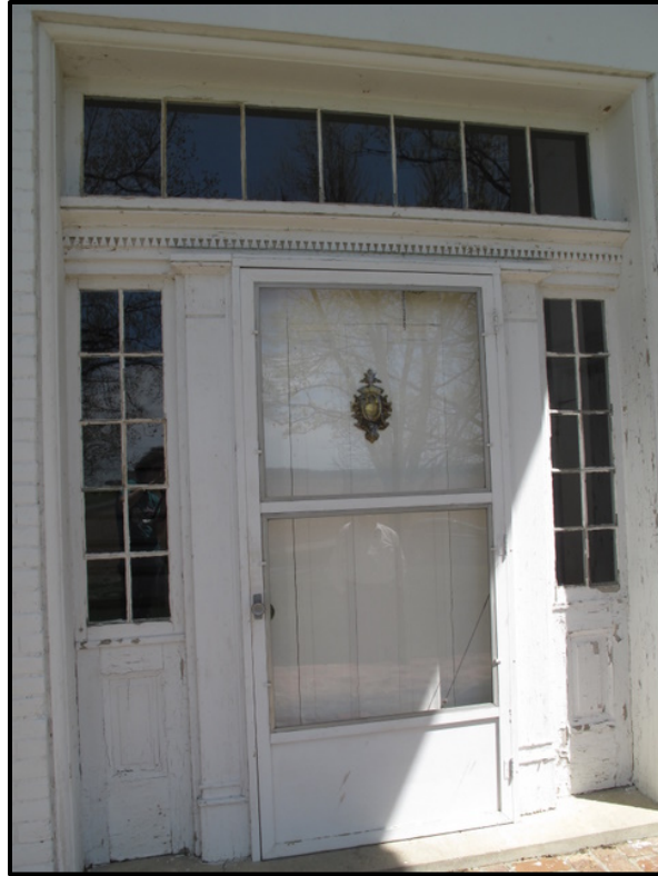
Figure 6. 23 Central entryway, LV-56. The use of transom, sidelights, inset panels and denticulation is common of the vernacular Greek Revival expression in Livingston County.
