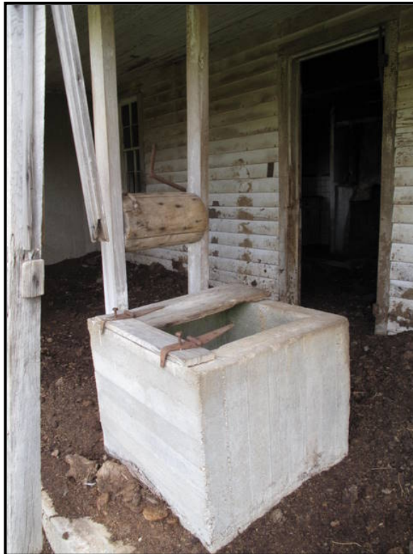
Figure 4. 33 Cistern/well on back porch at LV-74.
