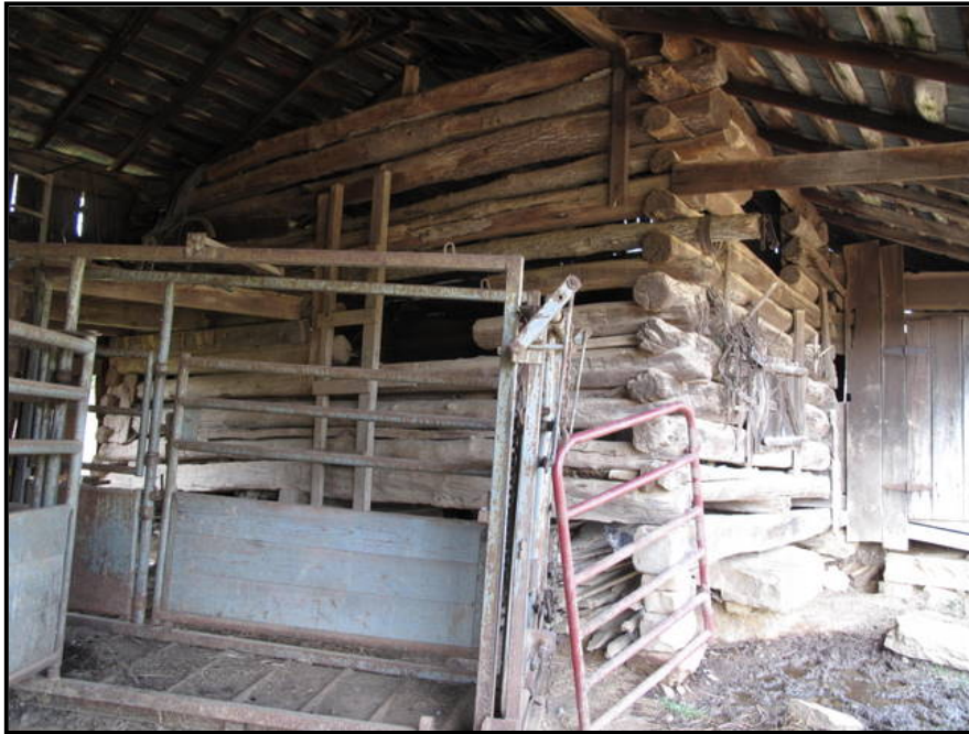
Figure 3. 20 Detail of the right hand side crib at CN-67.
