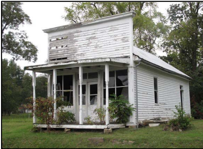
Figure 5. 18 Dr. Davenport's office, LV-91, in Hampton, Livingston County.
