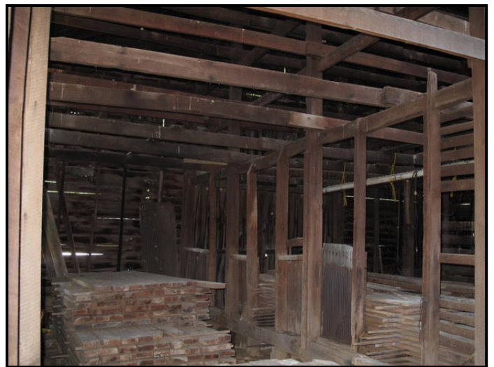
Figure 3. 57 Interior of CN-45.
