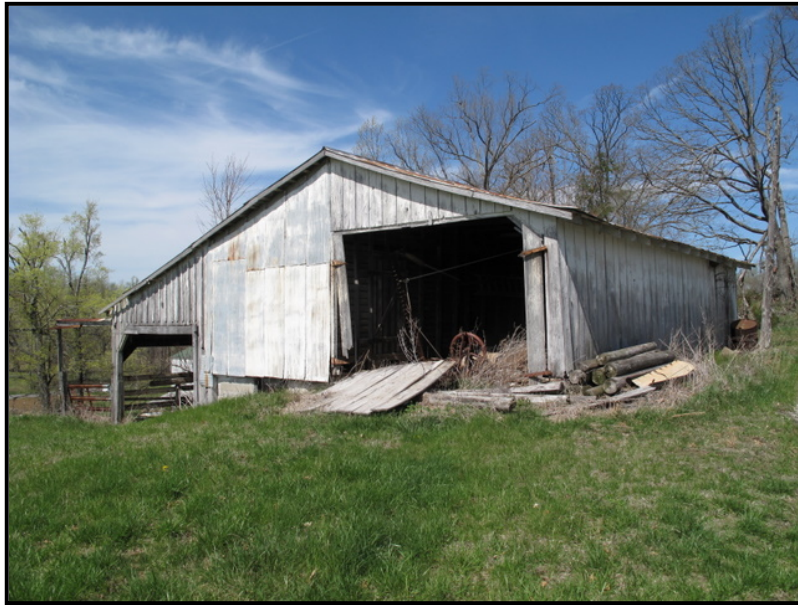
Figure 3. 78 Corncrib at the Old Smith Farm, LV-54.
