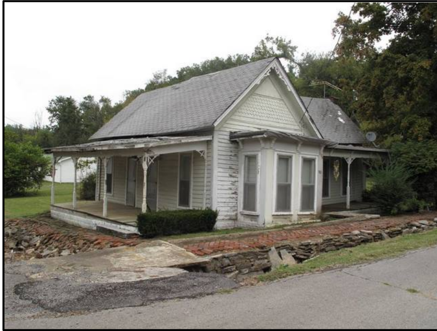
Figure 6. 42 Late-nineteenth century Cumberland in Dycusburg (CN-74). The dwelling has Italianate and Queen Anne stylistic details.
