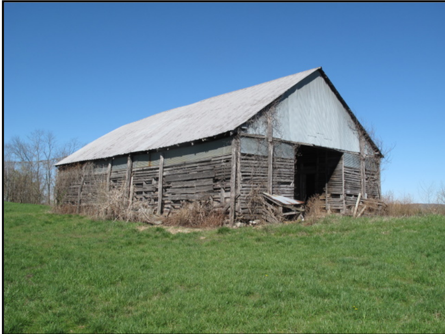
Figure 3. 76 Corncrib at CN-31, south and east elevations.
