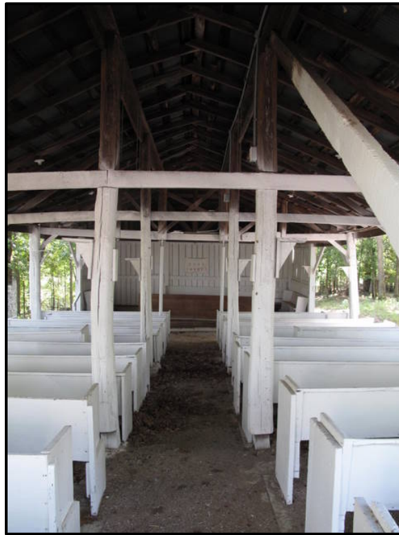
Figure 5. 37 Interior of shed at CN-68.
