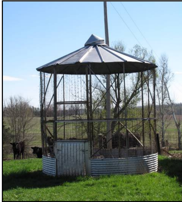
Figure 3. 81 Circa 1950s wire mesh corncrib at LV-51.
