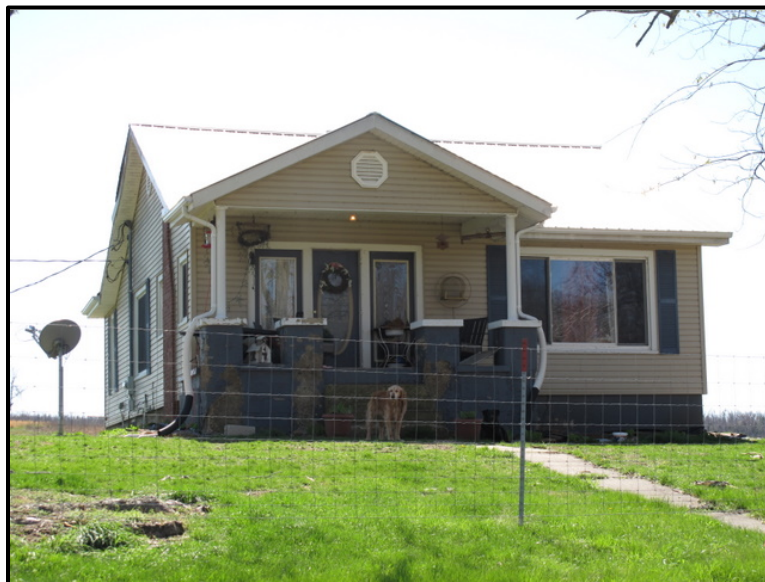
Figure 6. 47 CN-35, a possible Wigginton-built bungalow in Crittenden County.
