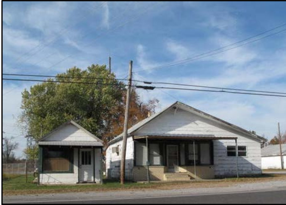
Figure 5. 8 LV-101 and LV-102 in Burna.
