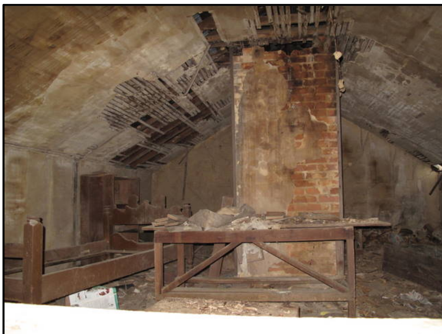
Figure 6. 33 Interior stack on upper story of LV-83, east side of house.
