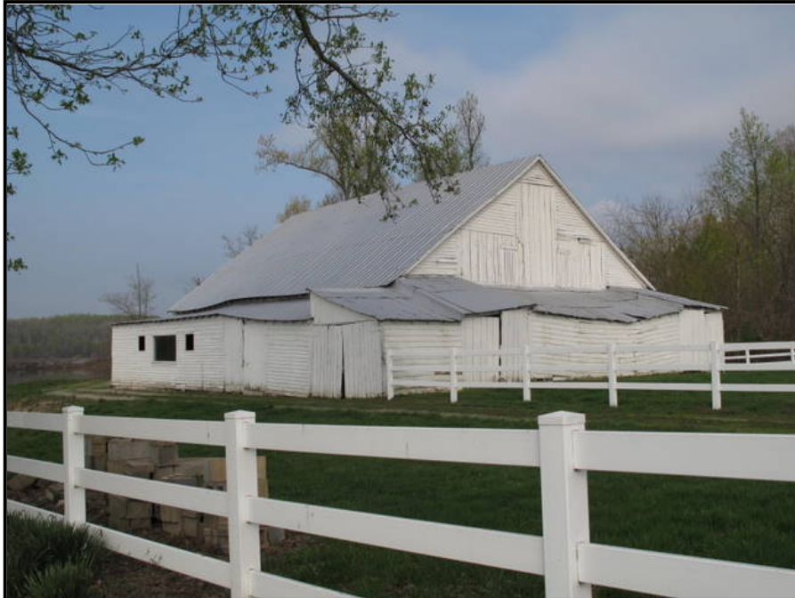
Figure 3. 27 Barn with multiple shed additions, LV-69, Kathleen Chipps Farm in Bayou, Livingston County.
