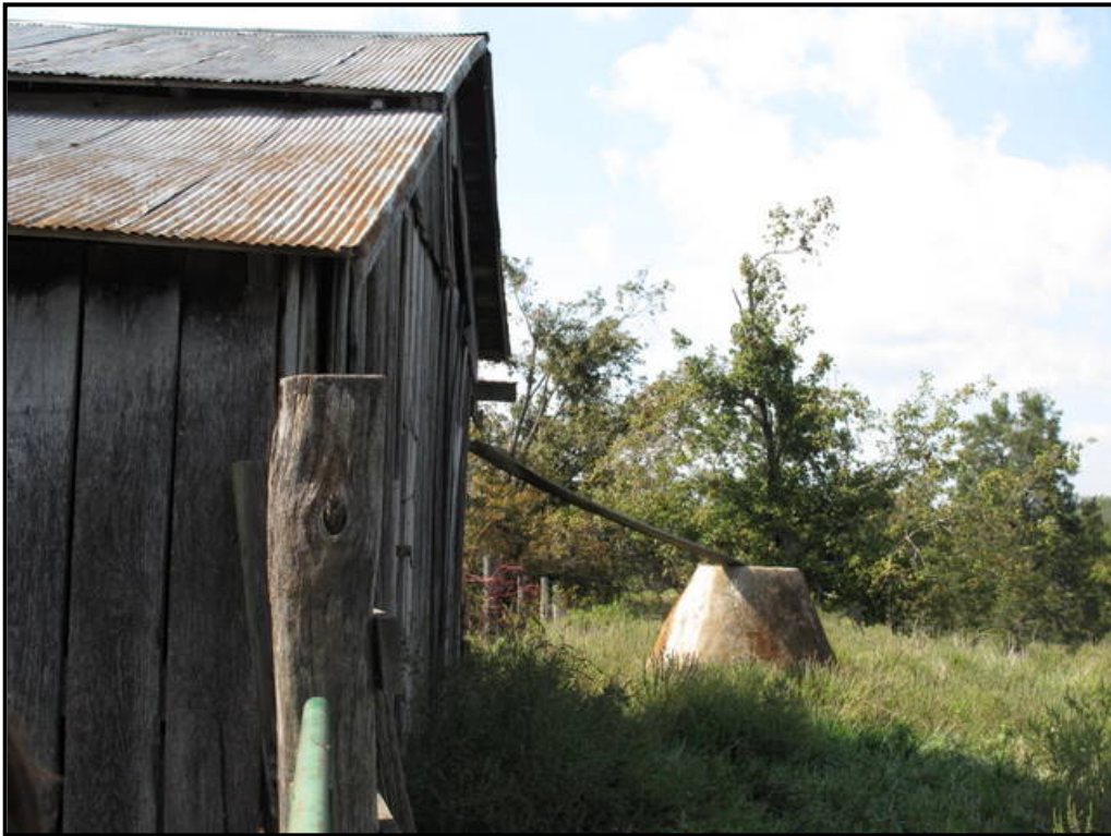
Figure 4. 30 Raised cistern in barn lot at CN-67.
