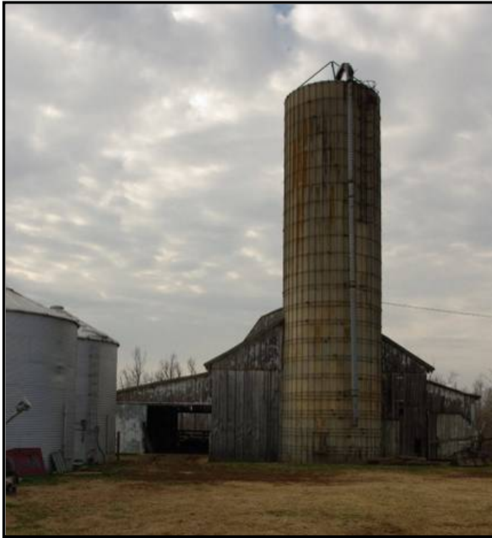
Figure 3. 85 Cement stave silo, with grain bins to the left at the Robert and Ada White Farm, CN-29.
