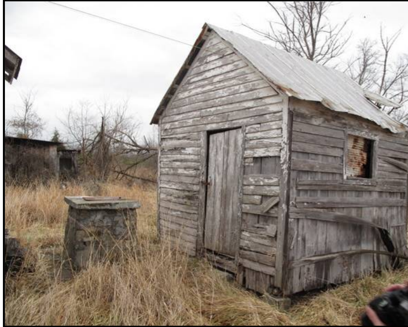
Figure 4. 2 Meathouse at CN-24. Note the horizontal weatherboards over the vertical board boxing. A raised cistern is located at left in photo.
