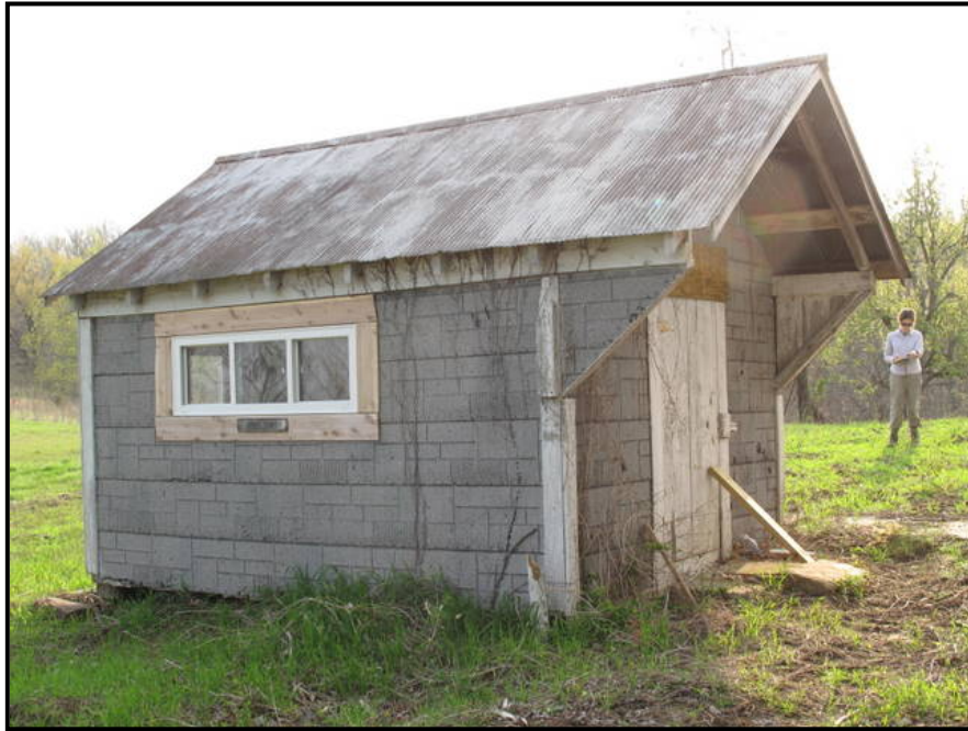
Figure 4. 6 Cantilevered front-gable meathouse at the Rudell Ford Farm, LV-62. The window on the side is a later addition.
