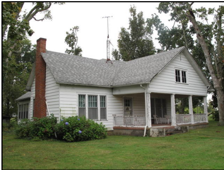
Figure 6. 51 Edward Davenport House (LV-90) in Hampton.
