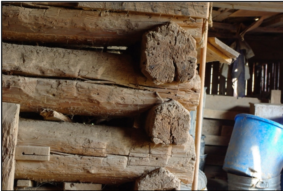
Figure 3. 8 Detail of log notching in barn at LV-42.
