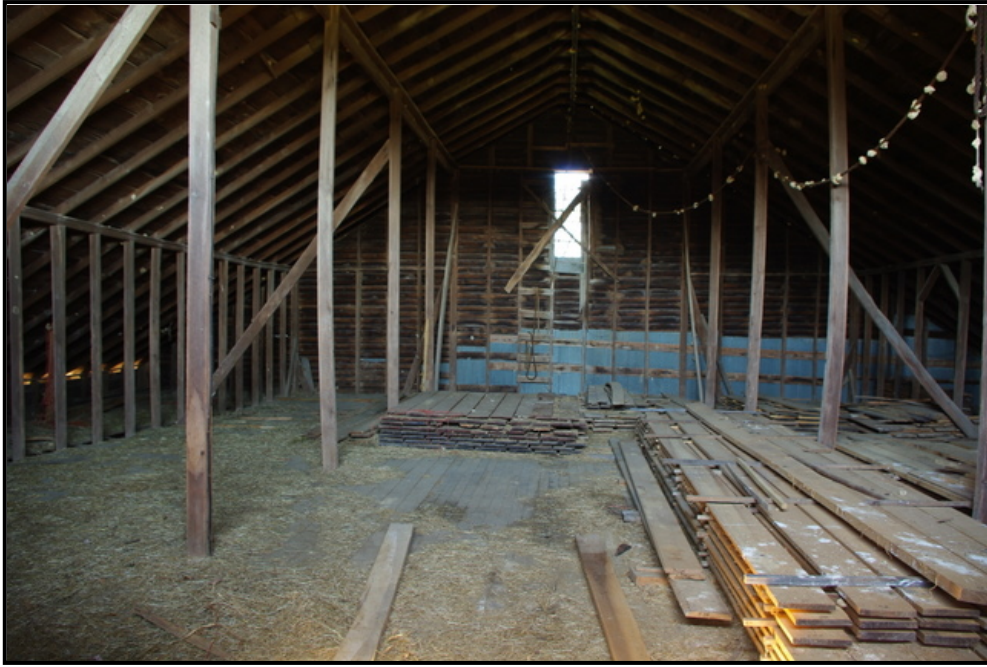
Figure 3. 65 Interior of loft at CN-41.
