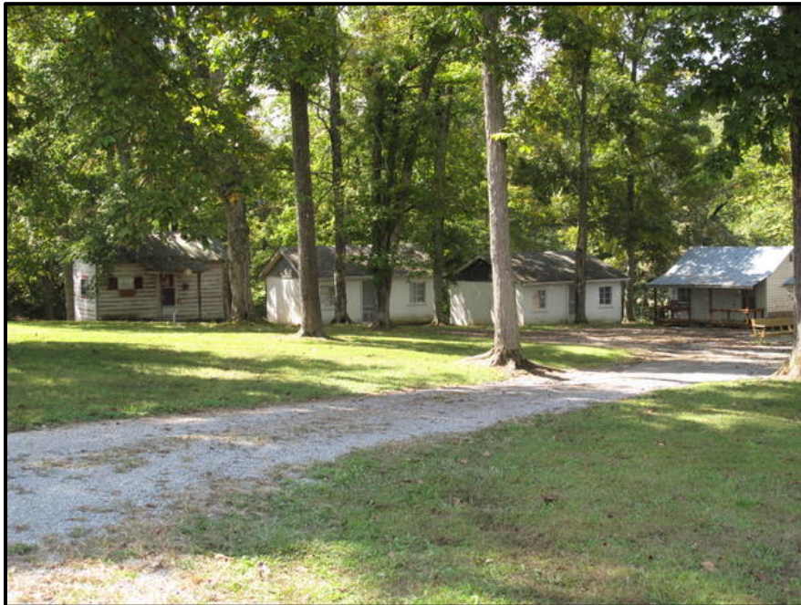
Figure 5. 42 View of lower cabins at Hurricane Camp near the dining hall.
