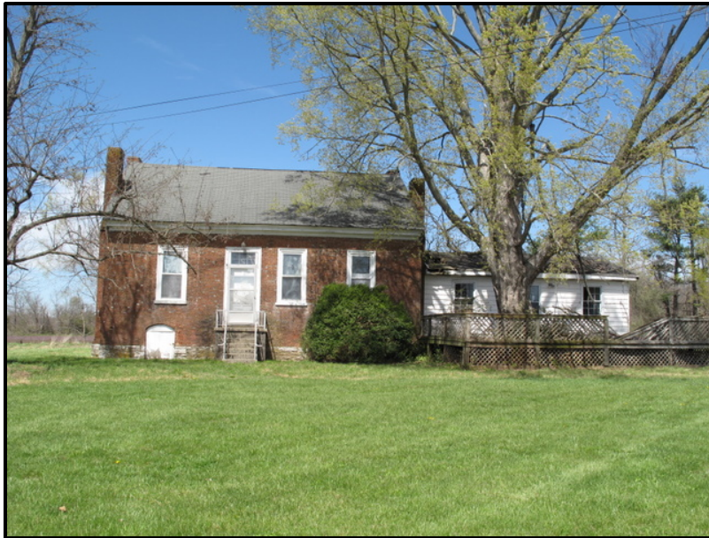
Figure 6. 20 Alvis House (LV-55), original rear elevation, facing northwest.
