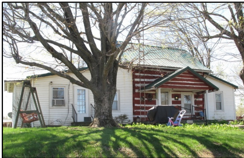
Figure 6. 1 CN-33, a single pen log house with side frame additions.
