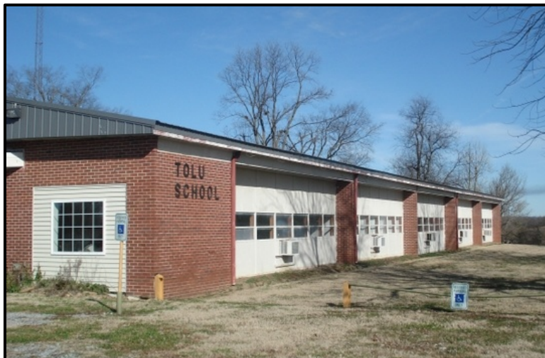
Figure 5. 29 Part of the façade and south elevation of Tolu School (CN-88). Photo by Kathleen Guess.
