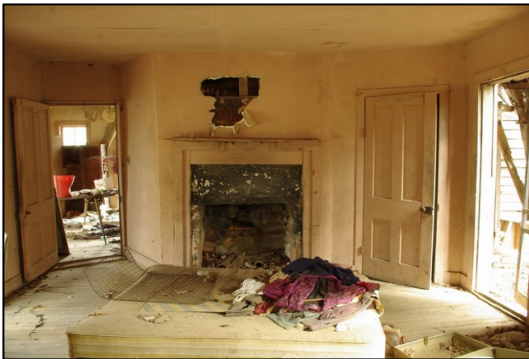
Figure 6. 28 Interior of CN-30, right-hand side room, showing diagonal firebox.
