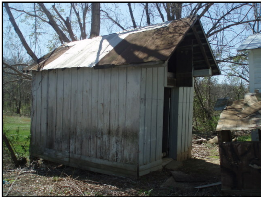
Figure 4. 7 Meathouse at the Trimble Farm on River Road, LV-25.
