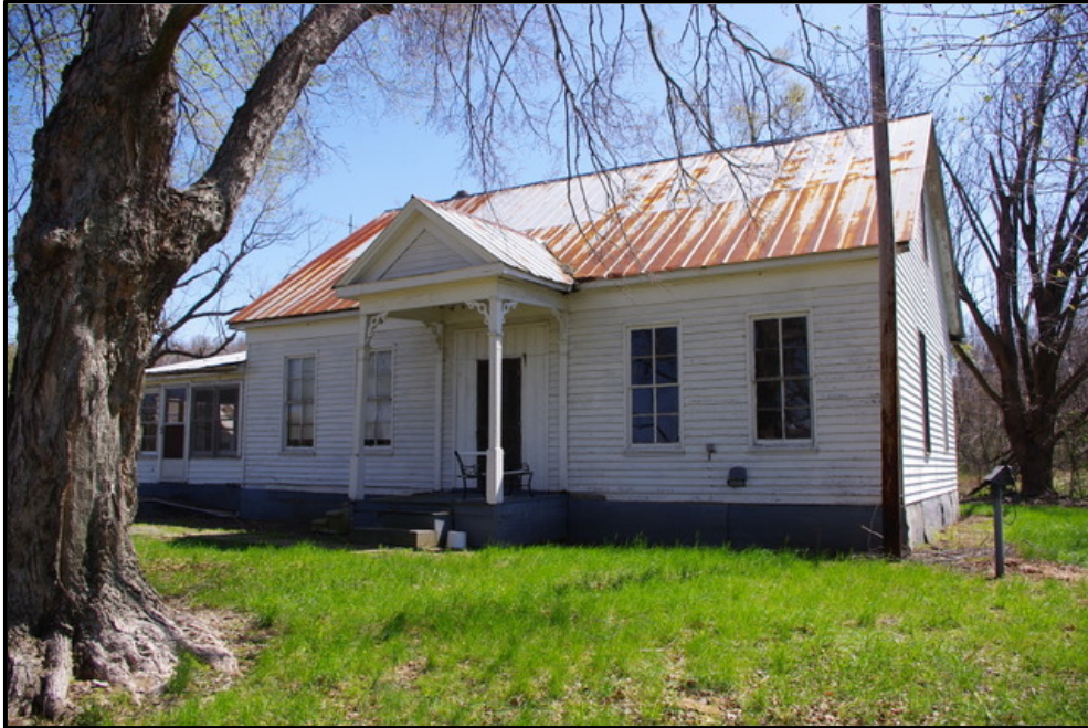
Figure 6. 29 Trimble House on River Road (LV-25).
