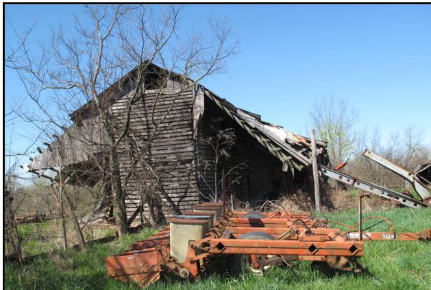
Figure 3. 69 East gable end of CN-32 corncrib, showing open north shed.
