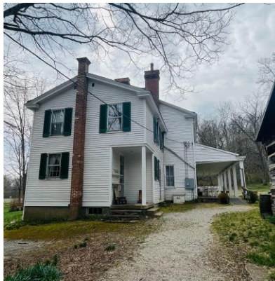
Photo 9: Main House Right Facade
