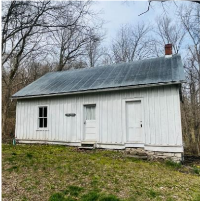
Photo 11: Wine House Front Facade
