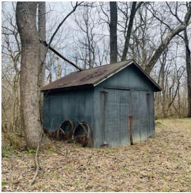
Photo 30: Corrugated Metal Shed
