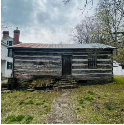
Photo 16: Slave Cabin /Cook House Front Facade
