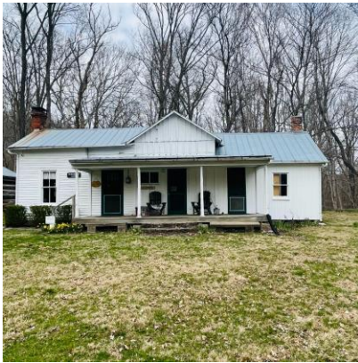
Photo 24: Roseberry House Front Facade
