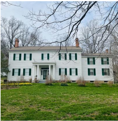
Photo 8: Main House Front Facade
