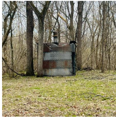
Photo 31: Corrugated Metal Silo
