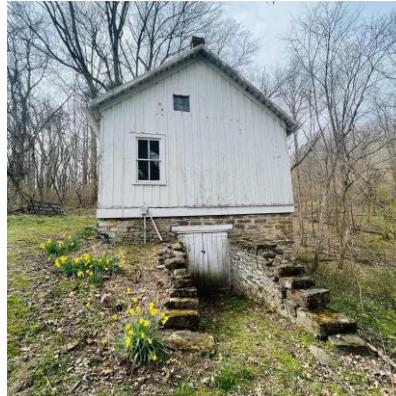
Photo 12: Wine House Side Facade
