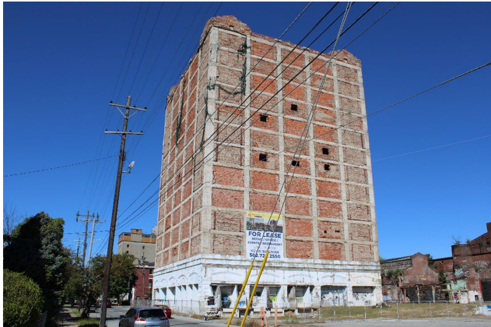
Figure 17. View of Property 5, south and west facades.
