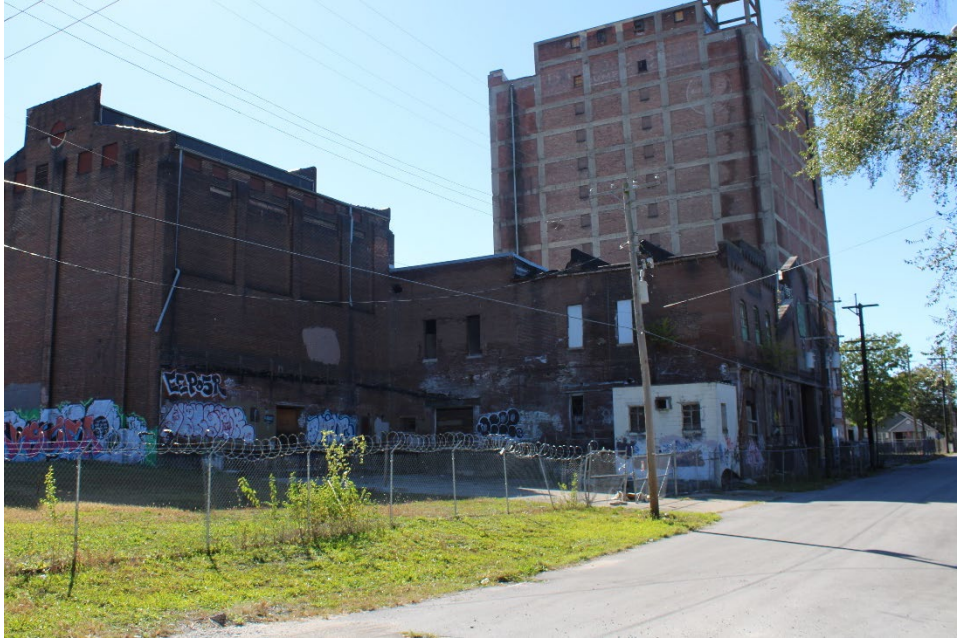
Figure 15. View of Property 4, east facade.
