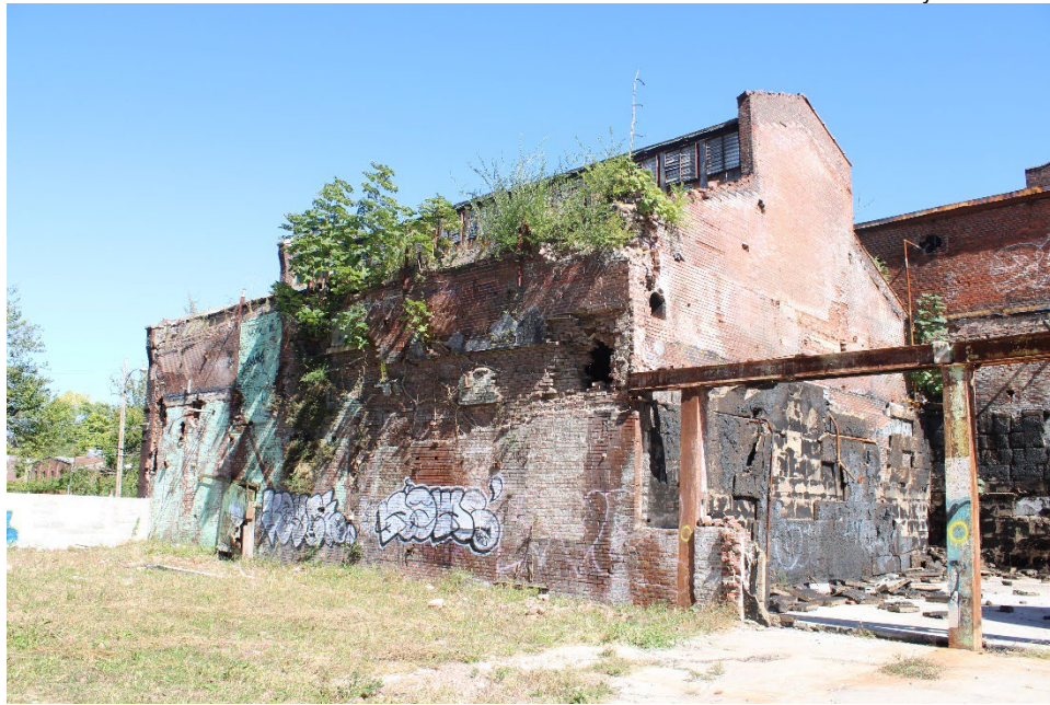
Figure 14. View of Property 3, south and west facades.
