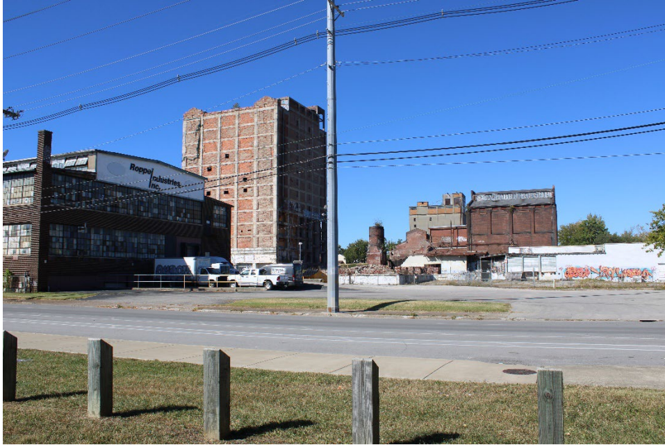
Figure 11. Overview of Properties 3-8 (the complex), facing northwest..
