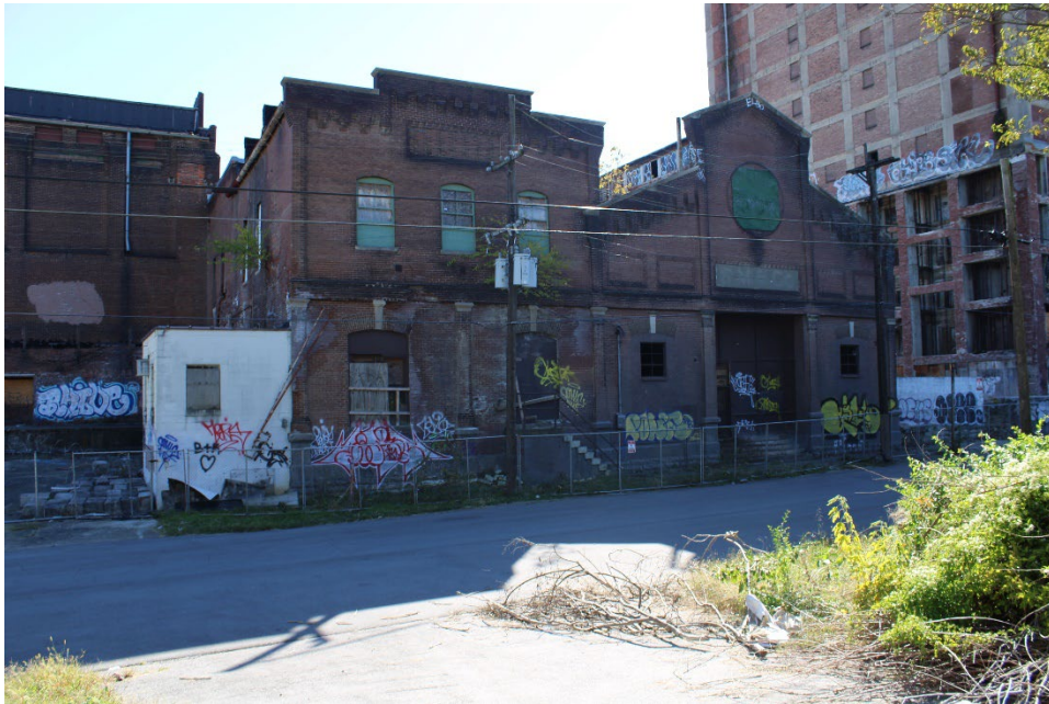
Figure 16. View of Property 4, north facade.
