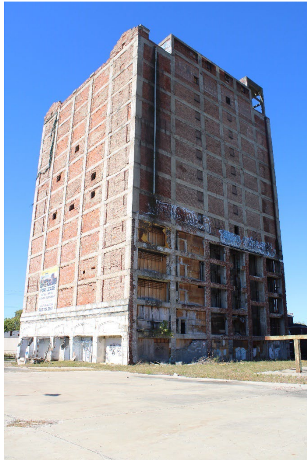
Figure 18. View of Property 5, south and east facades.
