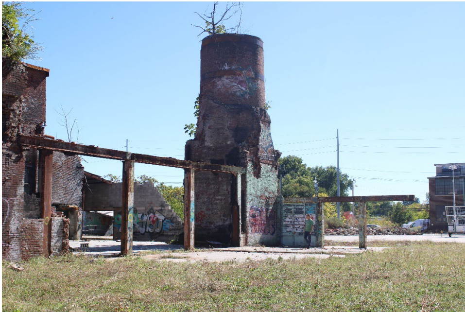
Figure 20. View of Property 6, looking southeast.
