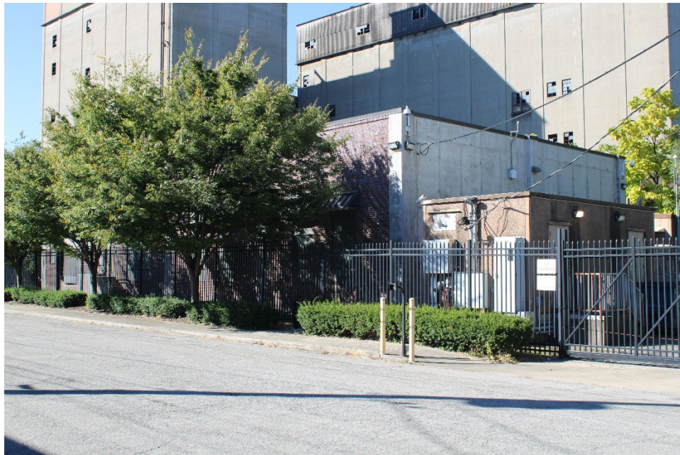
Figure 34. View of Property 13, south and east facades.
