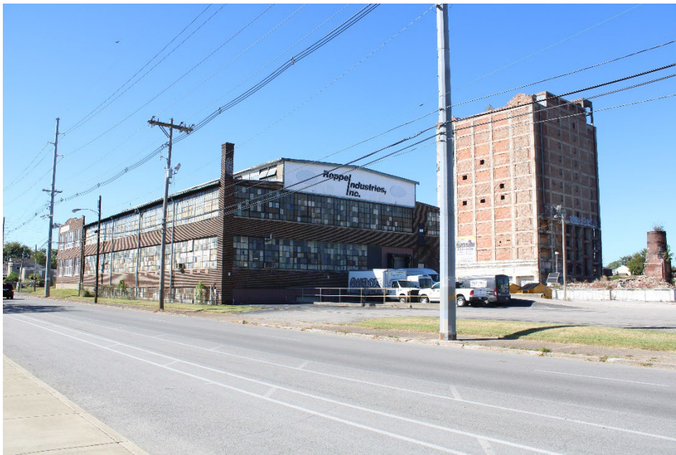
Figure 27. View of Property 9, south and east facades.
