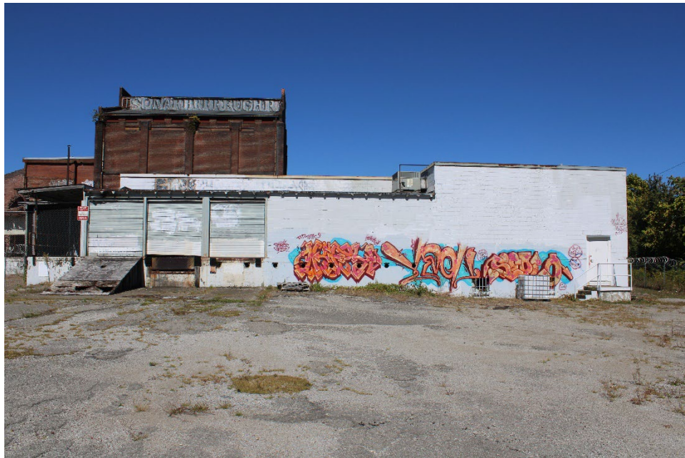
Figure 24. Property 8, south facade.
