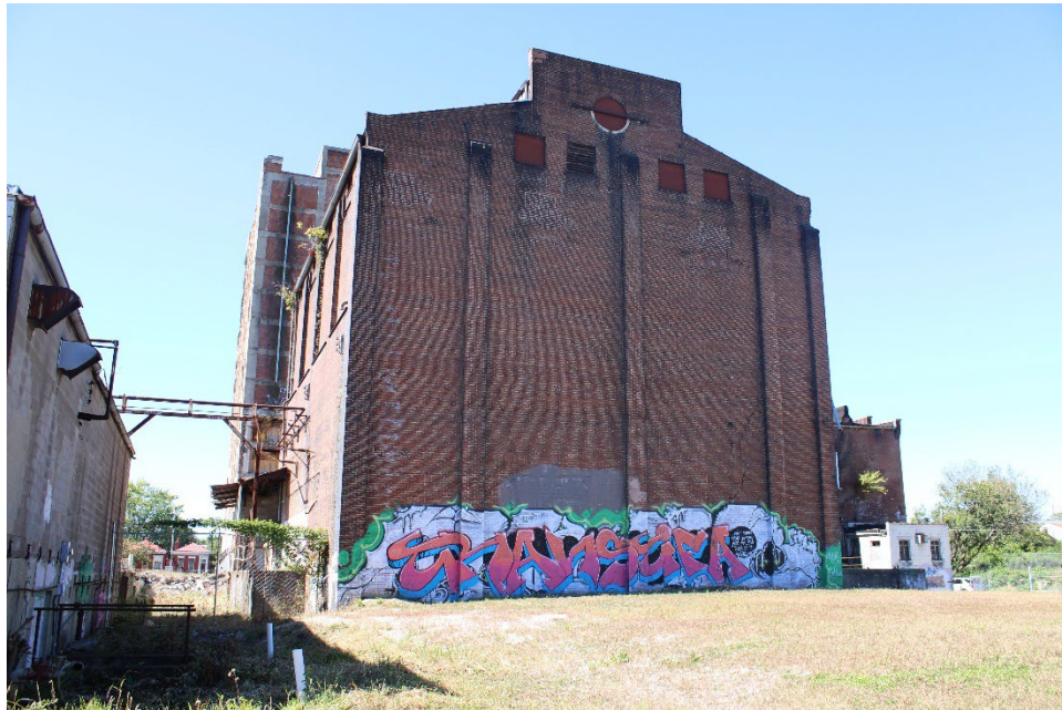
Figure 21. View of Property 7, east facade.
