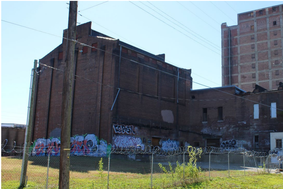
Figure 23. View of Property 7, south and east facades.
