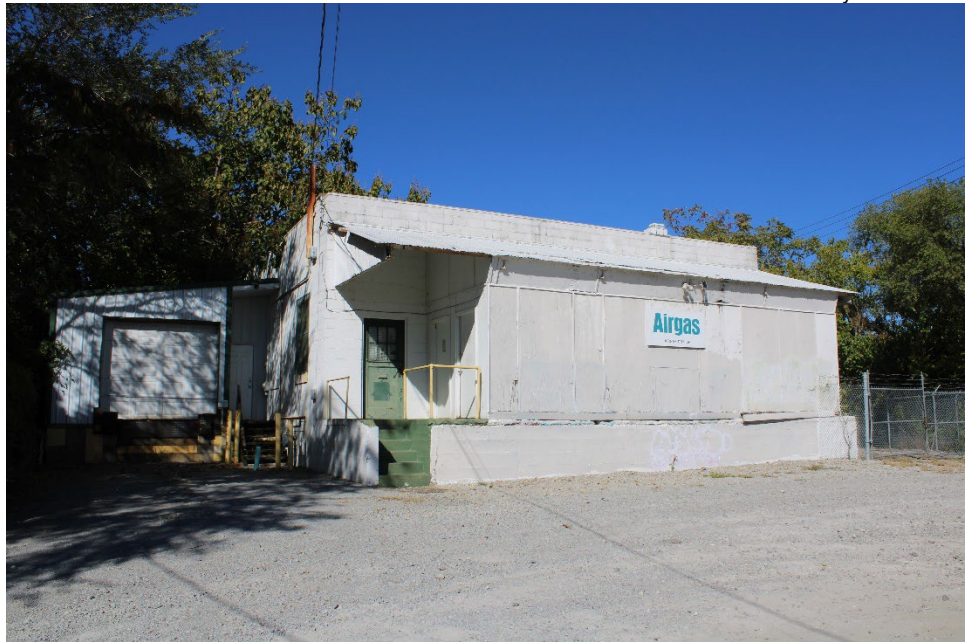
Figure 29. View of Property 10, south and west facades.
