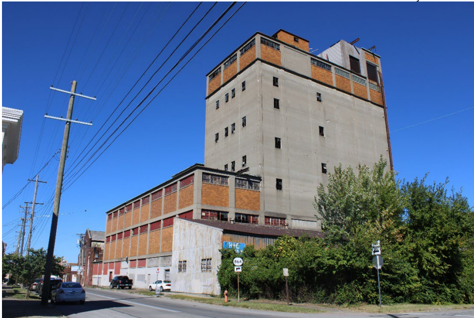
Figure 4. View of Property 1, south and east facades.
