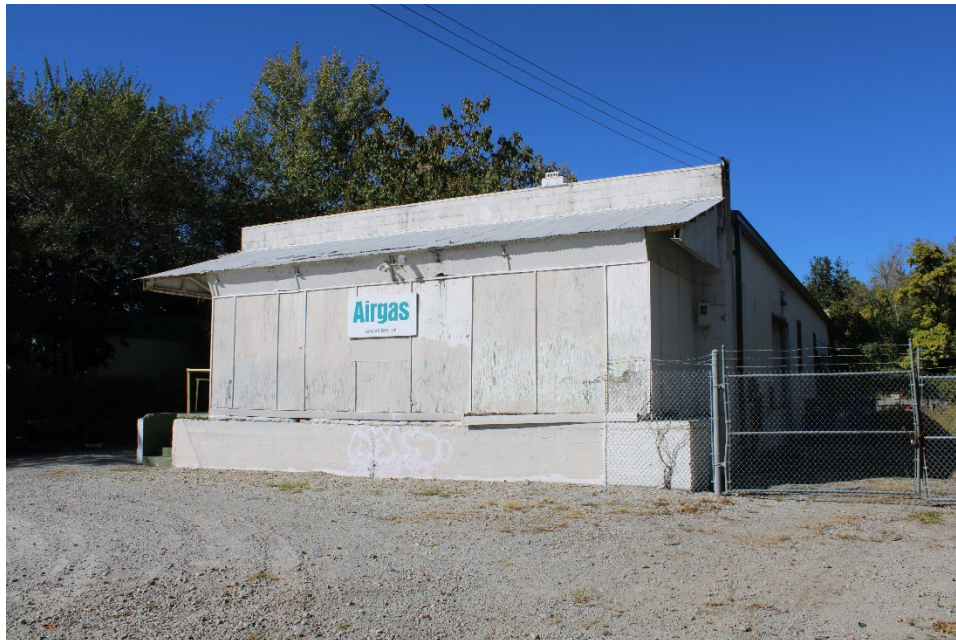
Figure 28. View of Property 10, south and east facades.
