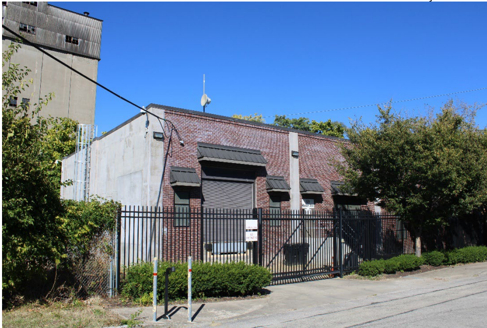
Figure 35. View of Property 13, south and west facades.
