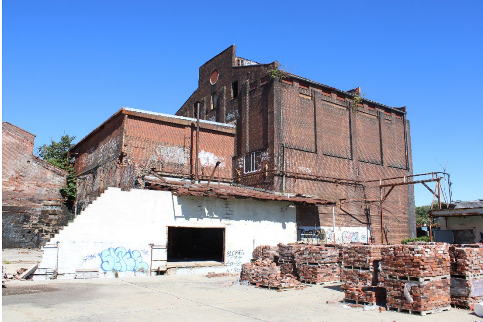
Figure 22. View of Property 7, south and west facades.
