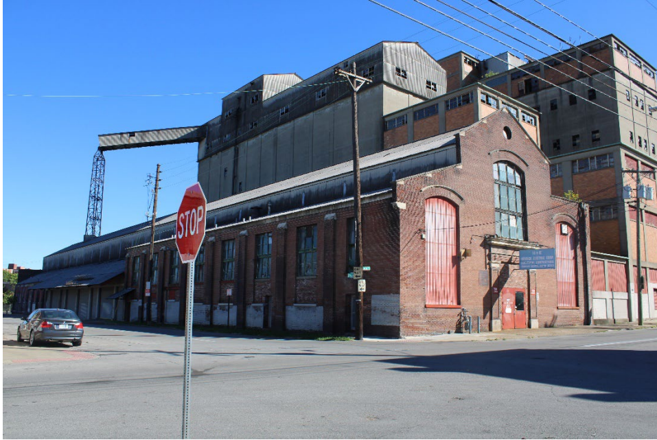
Figure 6. View of Property 1, north and east facades.
