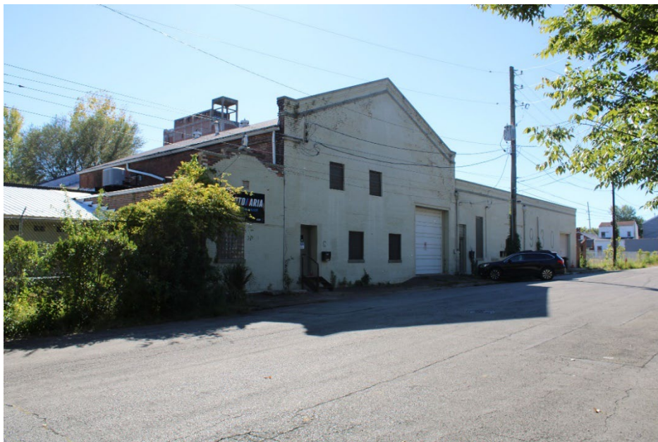
Figure 33. View of Property 12, north and east facades.
