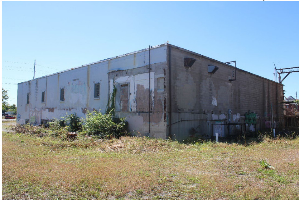
Figure 25. View of Property 8, south and east facades.
