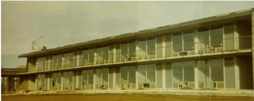
Figure 05: Construction photo ca. 1970
