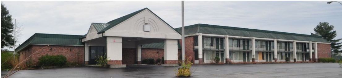
Figure 06: Photo of the property showing 1980s non-historic materials, Aug. 2022
