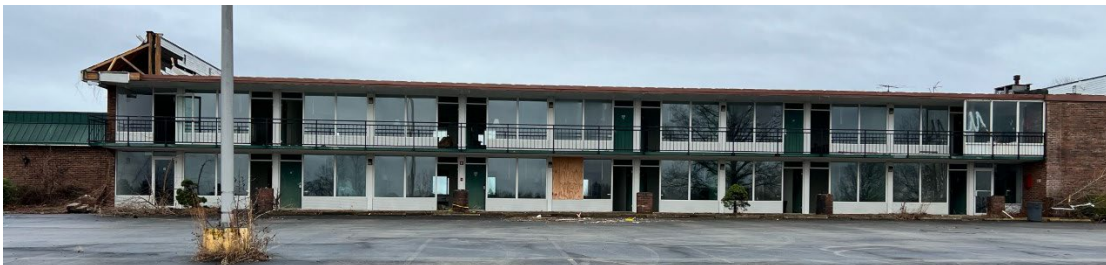
Figure 07: Selective demolition of the non-historic materials in progress, fall 2022
