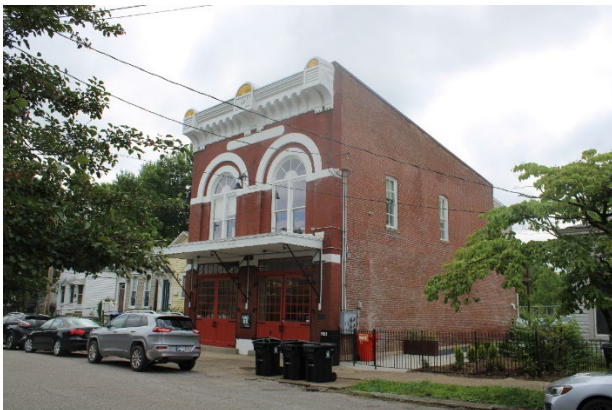
NRHP-Listed Firehouse at 1122 Rogers St.
