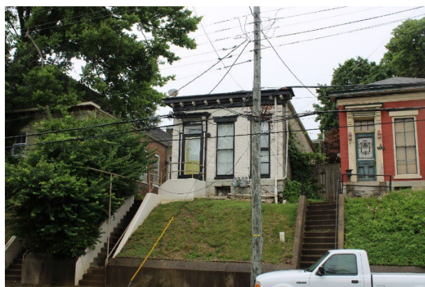
Shotgun House, 111 Spring Street
