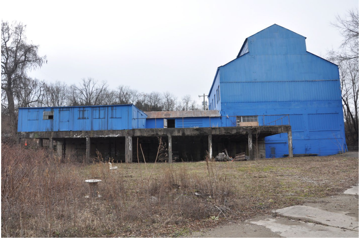
Figure 10: Northeast (rear) elevation of the Magnus Metal Company Building, looking south-southwest.
