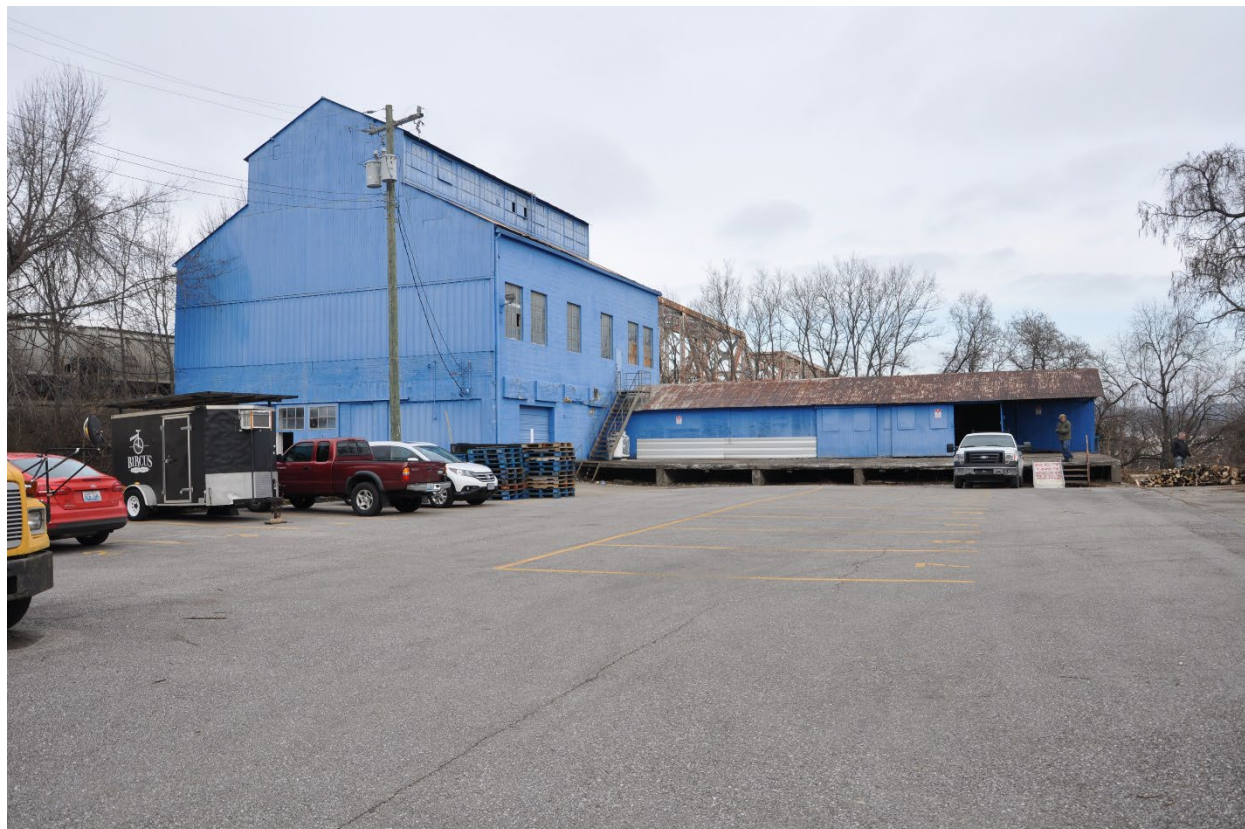
Figure 2: Façade (southwest) elevation of the Magnus Metal Company Building, looking north-northeast.
