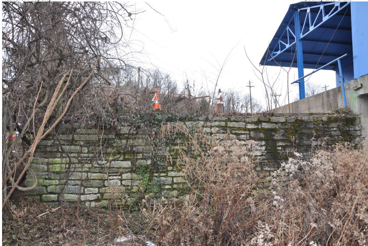
Figure 9: View of the quarried stone and mortar retaining wall, looking south-southwest.
