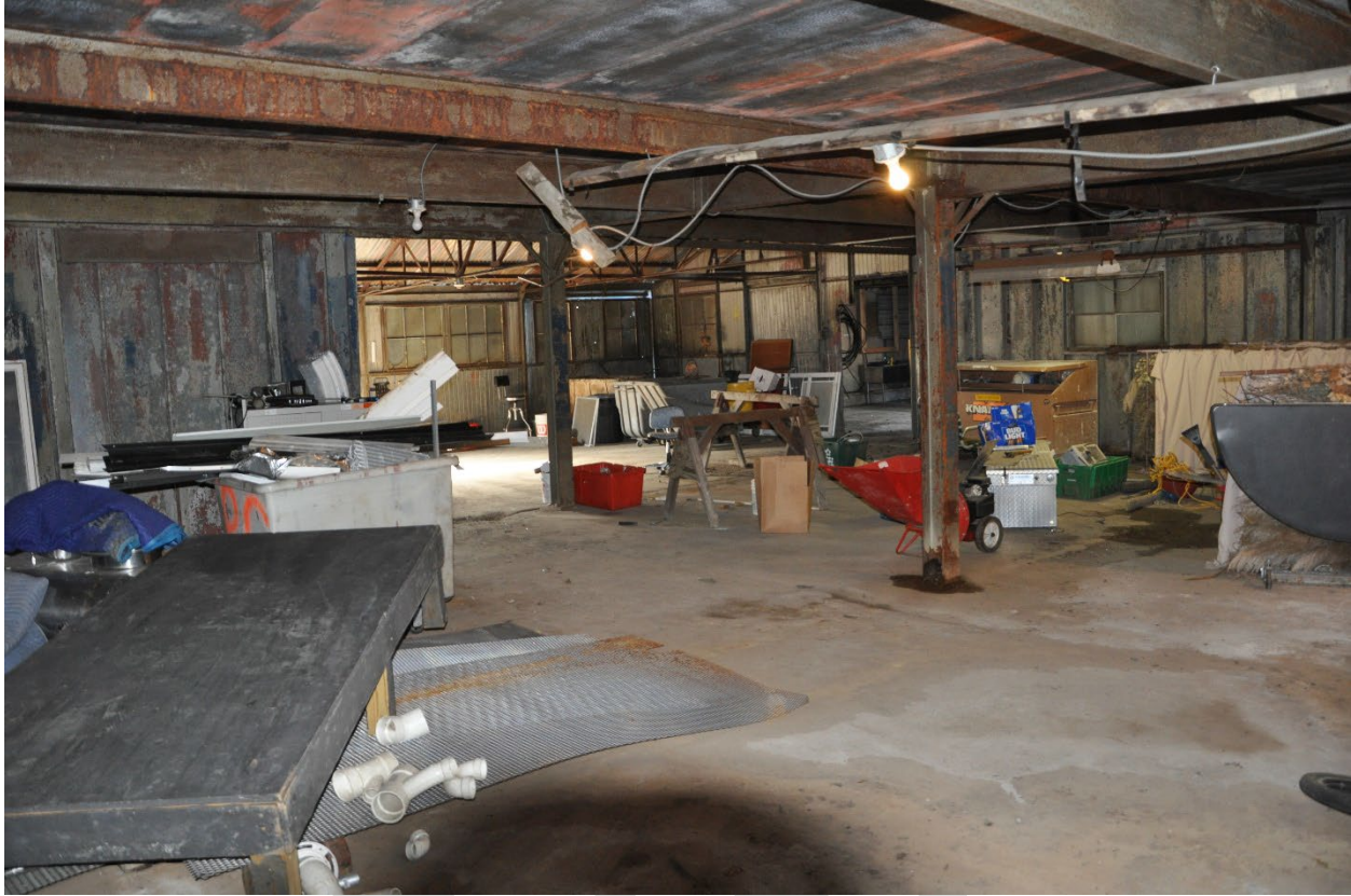
Figure 19: Interior view of the first story of the first and second additions of the Magnus Metal Company Building, looking southwest.
