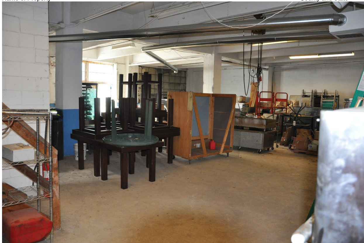
Figure 11: Interior view of the first story of the main block of the Magnus Metal Company Building, looking southwest.
