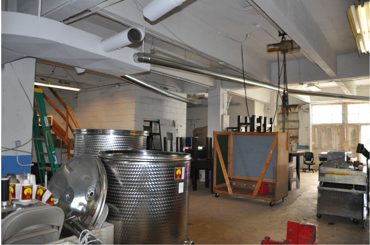
Figure 12: Interior view of the first story of the main block of the Magnus Metal Company Building, including the elevator shaft, looking southeast.
