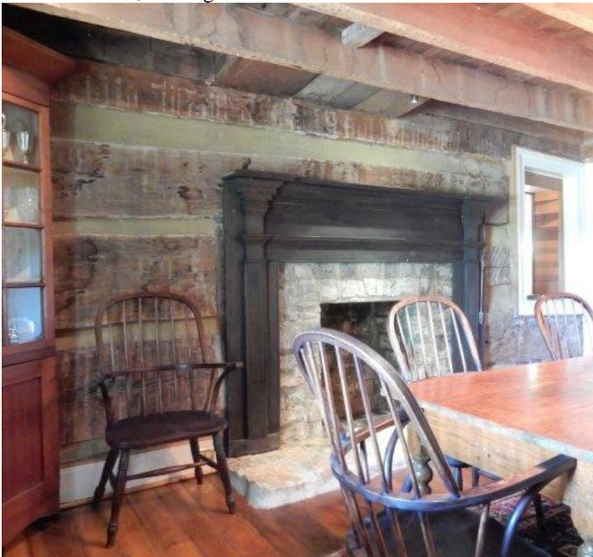
The room to the left (west) is now used as a dining room and its logs and 3" x 8" ceiling joists have been exposed. The room retains its original poplar floor and beaded baseboard, although much of the other
