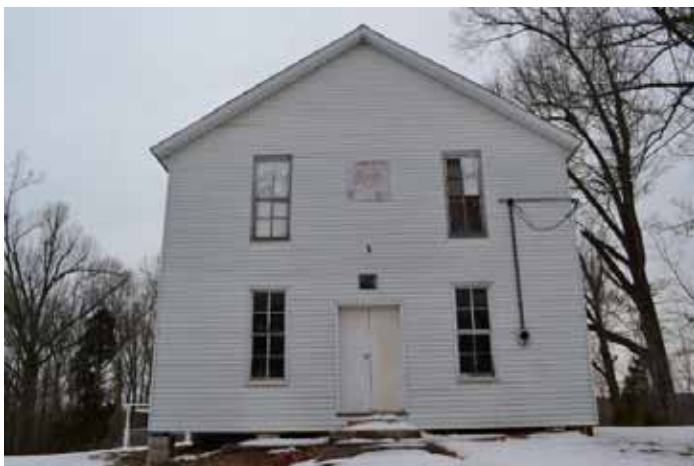
Photo 1: front (southeast) façade
