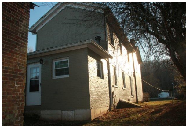
One-story 1970s addition
