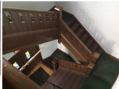
Looking down stairway
