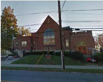
Bardstown Presbyterian Church
