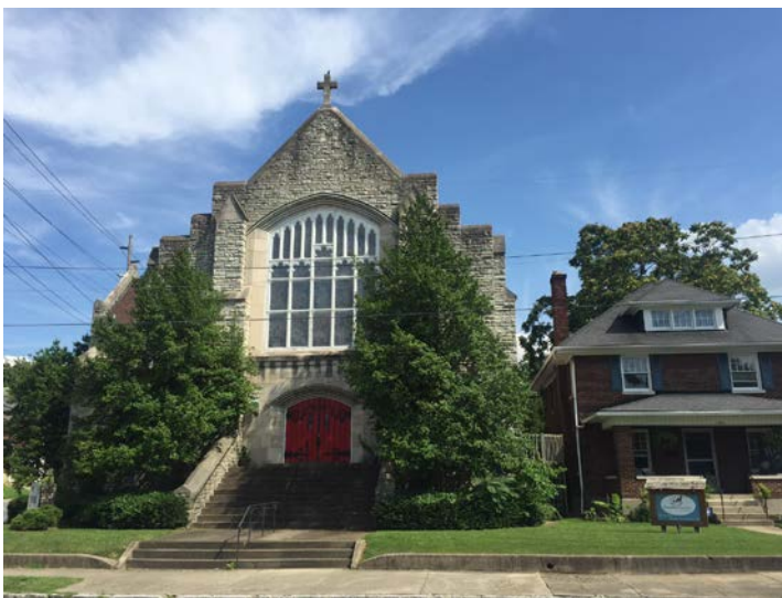
Northwest (main) façade, along Roanoke Avenue
