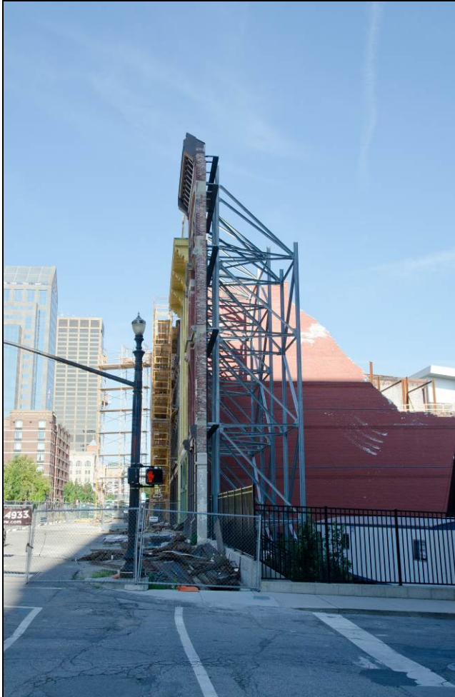
105 West Main Street, view from southeast.
