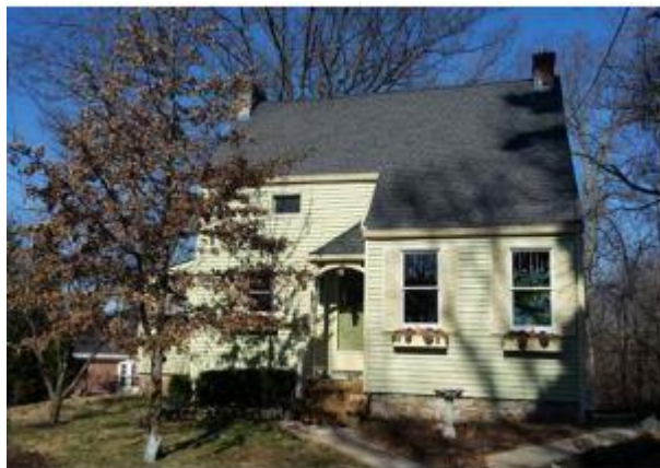
CPFT-125_01, Hubbard Main House, Façade (north elevation)
