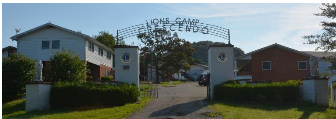
Camp entrance; Lodge on left, Admin Bldg on right
