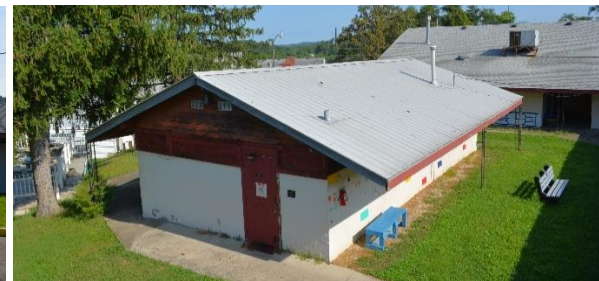
Men's restroom building (viewed from Dorm F balcony)
