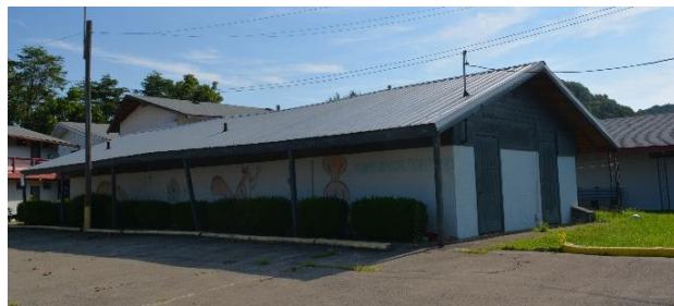
West side of women's restroom
