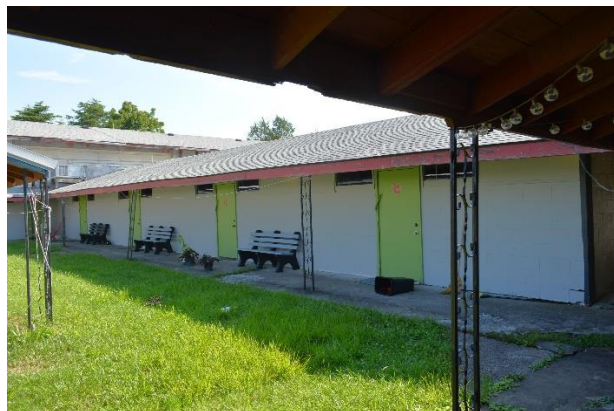
West side of dormitory D
