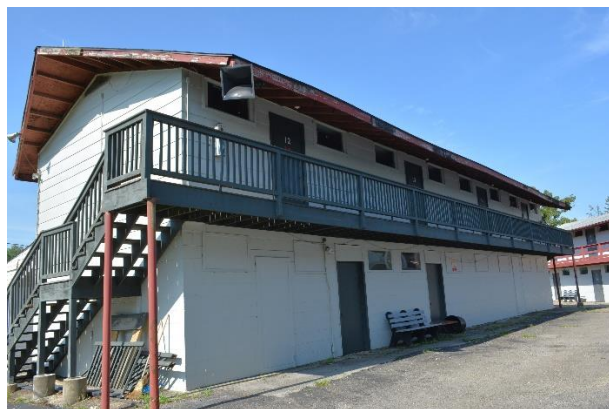
North side of dormitory C
