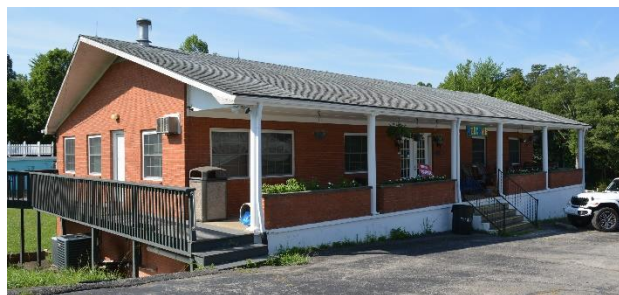
Main/north façade of Admin building
