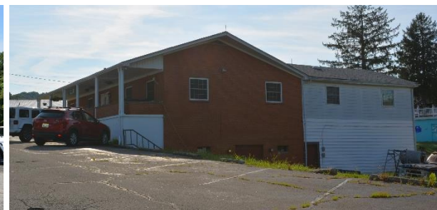
West façade – note filled-in basement below
