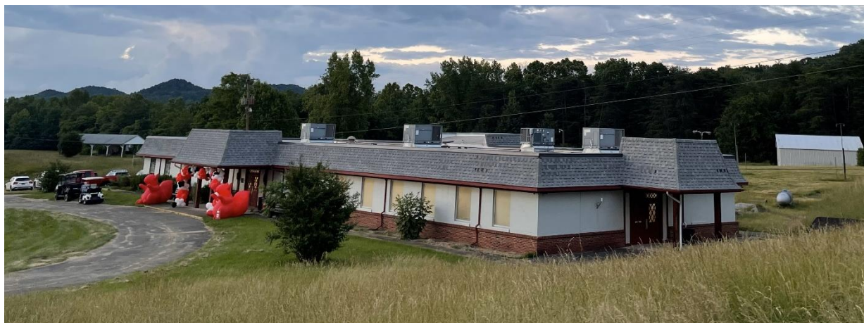
Cafeteria / mess hall, main entrance on west façade with driveway loop from Pine Tavern Road
