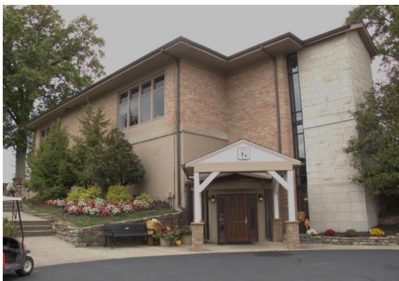
South façade Clubhouse (left of corner entry)
