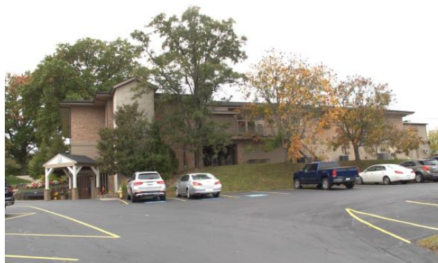
East façade of Clubhouse
