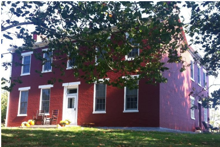
Front (southwest) façade; southeast side on right
