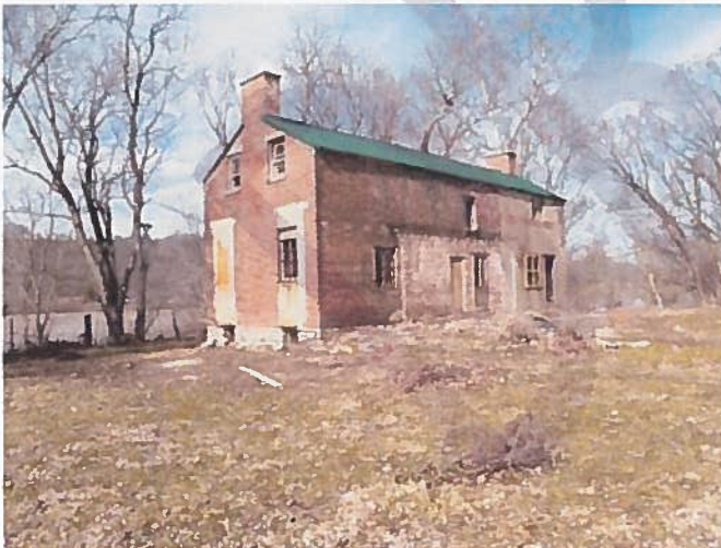
Southwest side and southeast (back) side, to North
