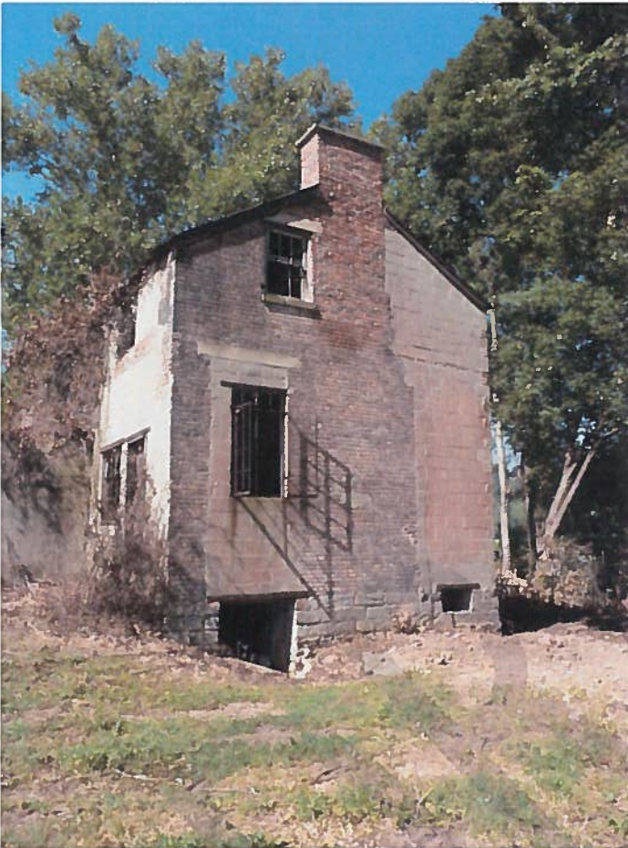
Northeast side with cellar entrance
