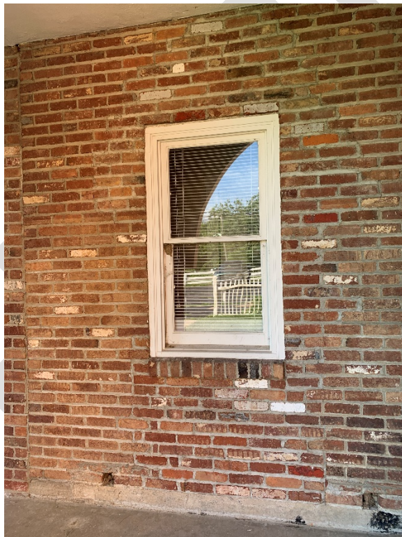
Photo 12: Façade of northwest gable-end section of 1948 addition, note brick infill and poured concrete foundation, view northwest
