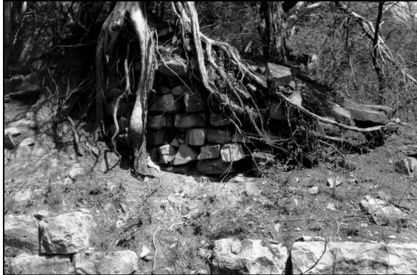
Figure 6. Photograph of the Top of the West Façade of the Shrull Lime Kiln Facing East Showing the Sandstone Interior Lining.
