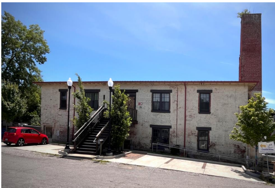
Section A of Luigart Malt House, north elevation (June 2024)
