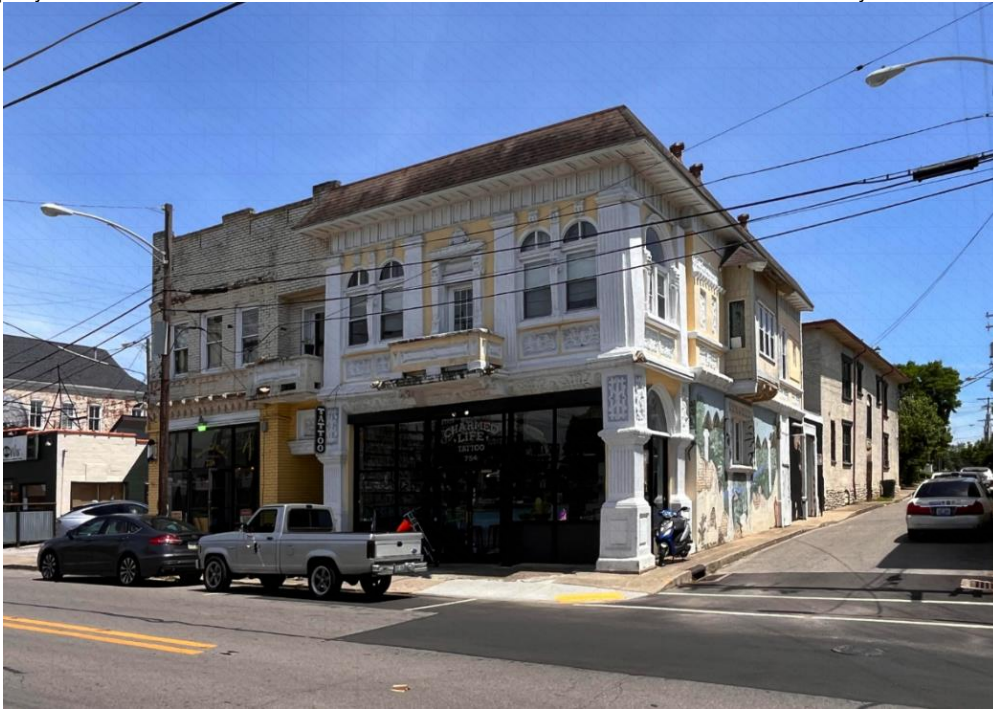
758 and 754 North Limestone, west elevation (June 2024)
