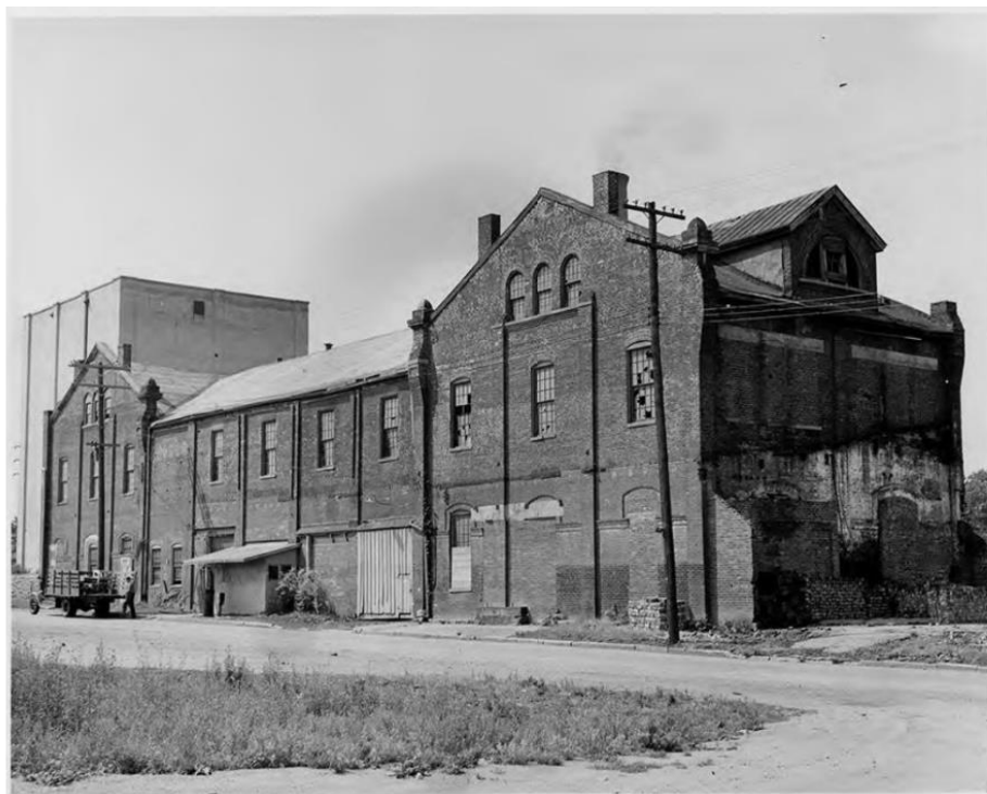
Photograph of old power plant on Loudon Ave, facing east (J. Winston Coleman collection)
