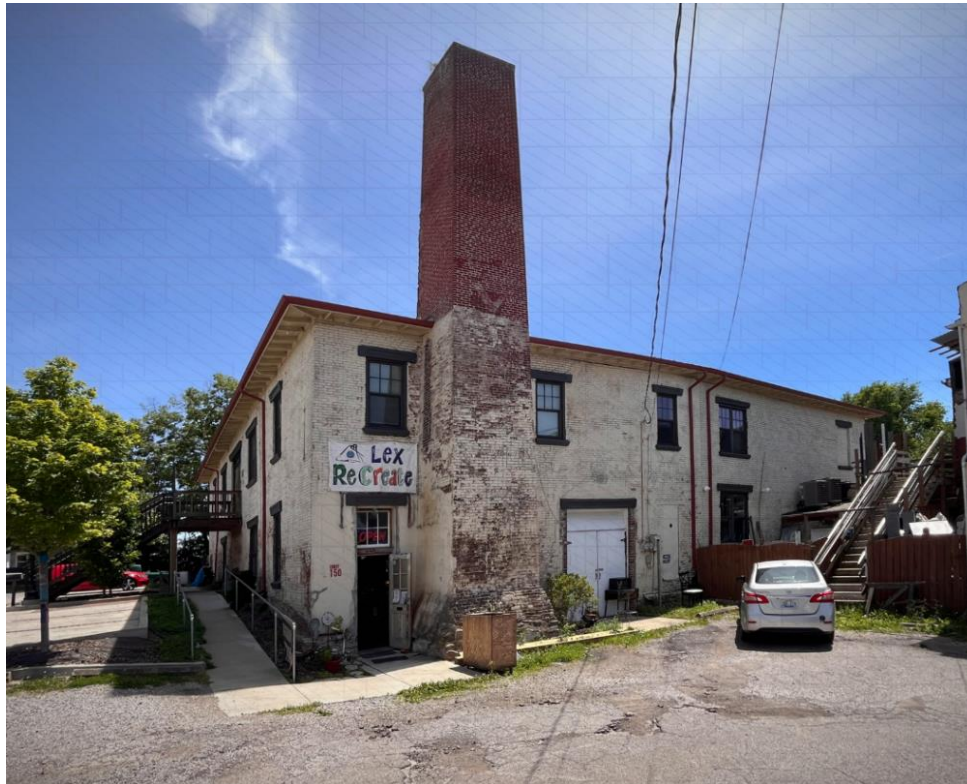
Section A of Luigart Malt House, west elevation (June 2024)
