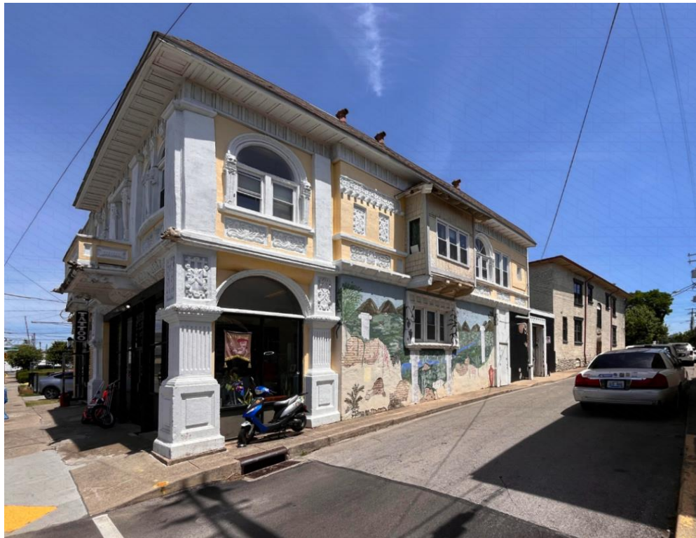
South elevations of 754 North Limestone and malt house, Section B (June 2024)
