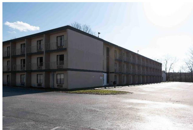
Photo 6, Wing B at left, Wing C at right
