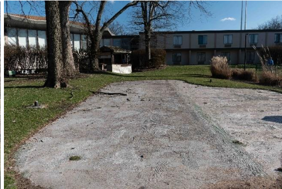
Concrete Pad for Putting Green
