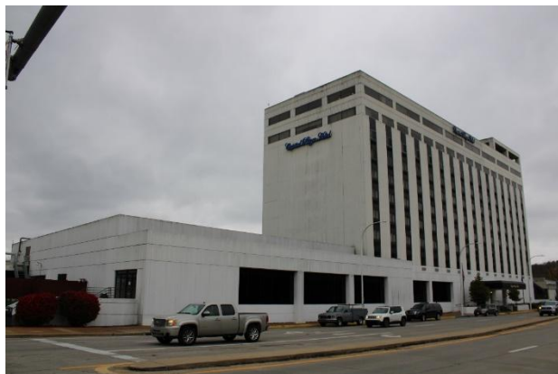
North and West Façades, camera facing south
