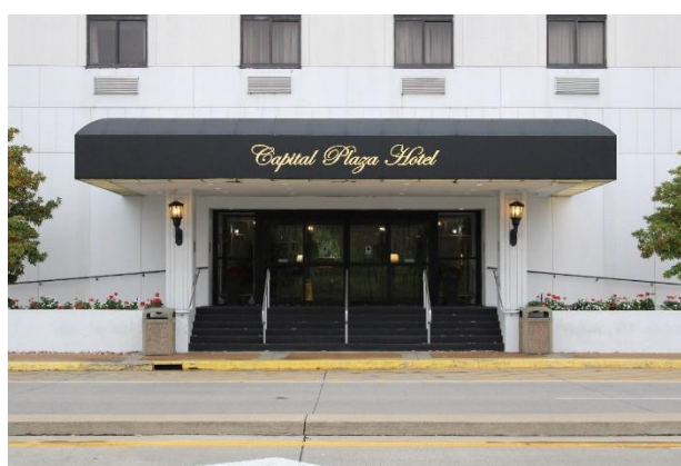
Front entrance, West Façade
