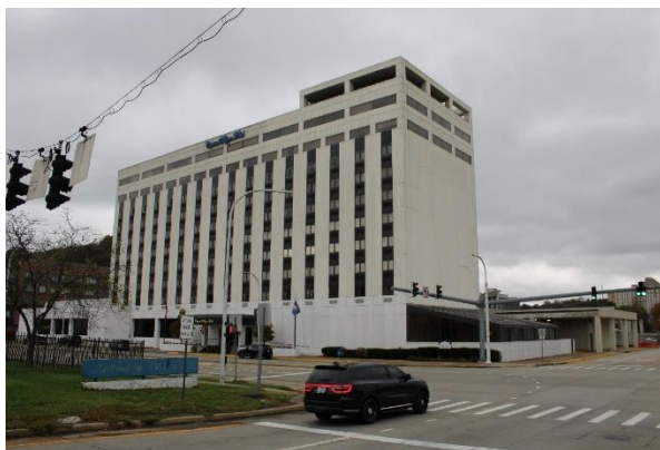
West and south façades, camera facing east
