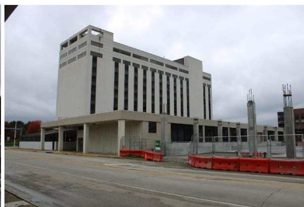
East Façade, camera facing north
