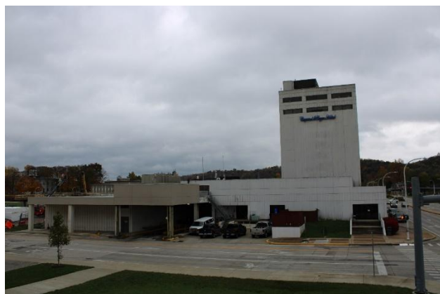
North Façade, camera facing southwest
