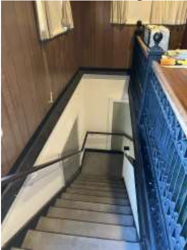
Photo #14 (KY_Campbell County) Interior, 2 nd Floor Stairway, camera looking North
