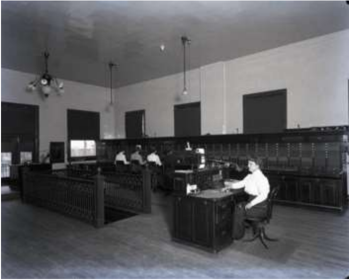
Historic Photo – Switching Room
