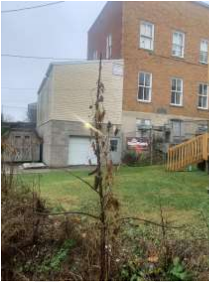
Photo #1 (KY_Campbell County) Exterior, Northeast Corner, camera facing southwest
