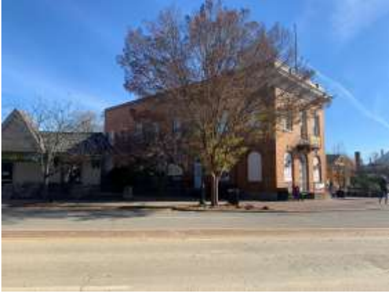
Photo #12 (KY_Campbell County) Exterior, Northwest Corner, camera facing Southeast
