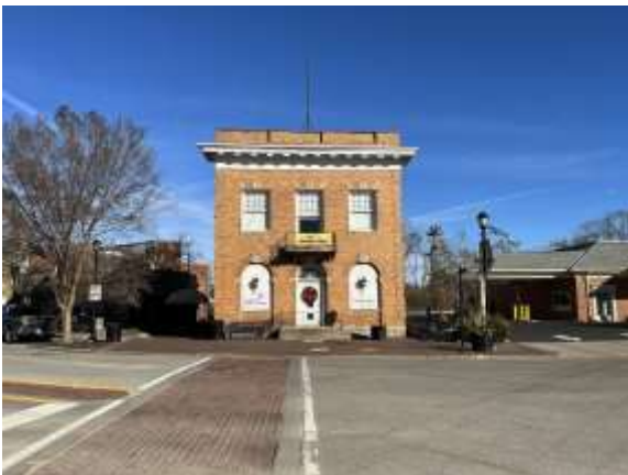
Photo #5 (KY_Campbell County) Exterior, West Façade, camera facing East
