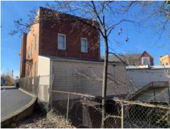
Photo #13 (KY_Campbell County) Exterior, Southeast Corner, camera facing Northwest
