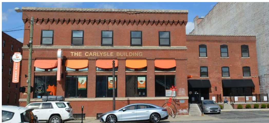
East Main Street façade, camera facing north. In the photo: western portion on left; eastern portion on right.
