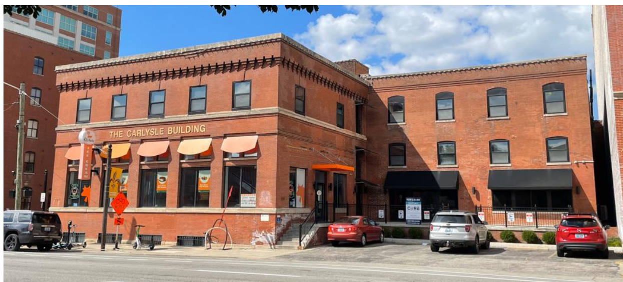
Front/south façade of Armour & Co. Branch House
