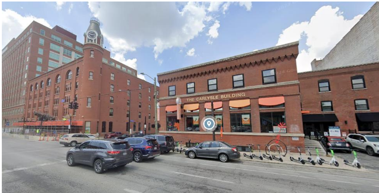
Louisville Public Warehouse (with corner clock tower) and the Armour & Co. Branch House
