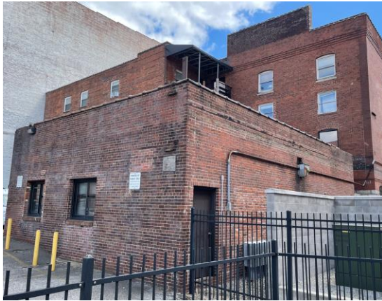
NW corner of utility building
