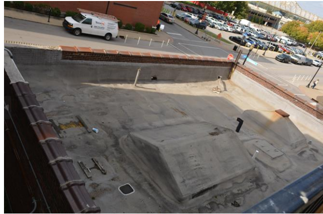
Roof of utility building
