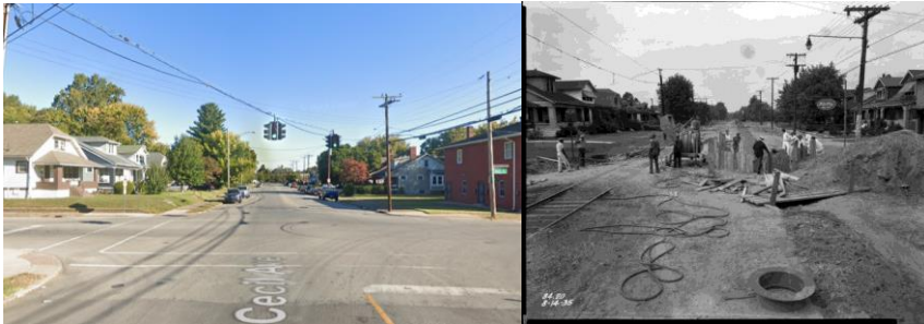
Figure 13. Sewer improvements at Cecil Avenue and Hale Avenue in 1935, and view today (University of Louisville Archives and Special Collections and Google Streetview)
