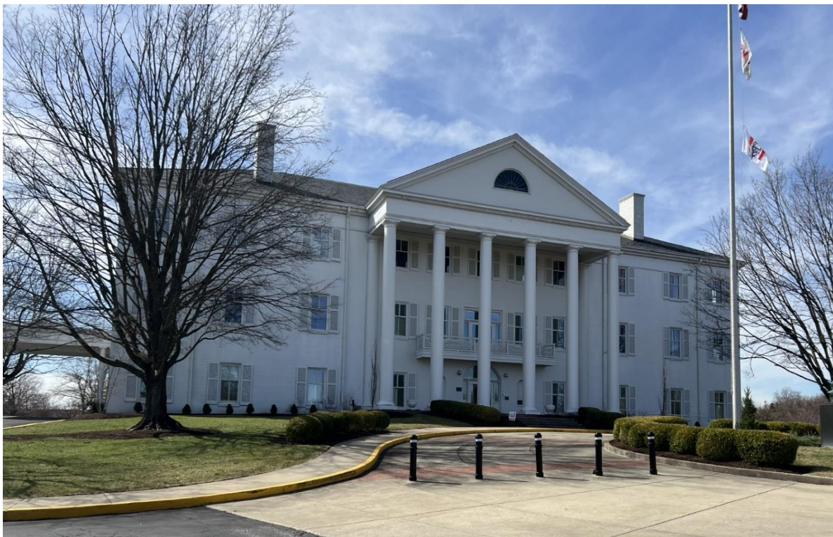
Photograph 1, KFC White House Building, North Façade, captured by Janine Webb, 2024
