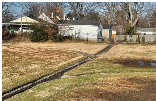
Detention basin at 4831 Redwing Way
