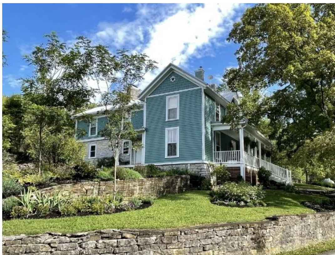
View of the south and west elevations of the main house
