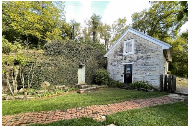
Root cellar and south end of rag house.
