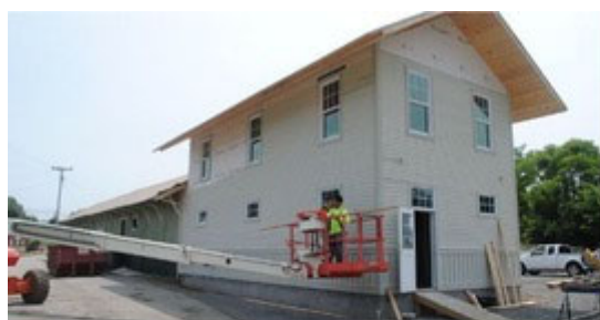
L&N RAILROAD PASSENGER STATION SCOTTSVILLE, KY
