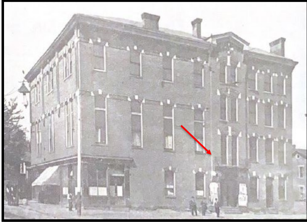
Figure 8. 635 6 th Avenue, I.O.O.F. Hall/City Building, 1898 image depicting east elevations double entry with cast iron awning frame with decorative cresting/rail (red arrow).
