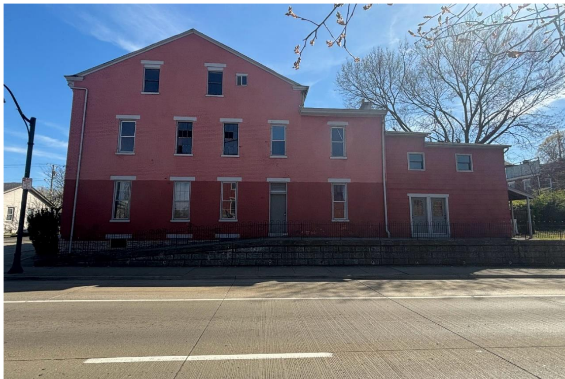
The Lubber House, Kenton County, Kentucky, north (side) facade
