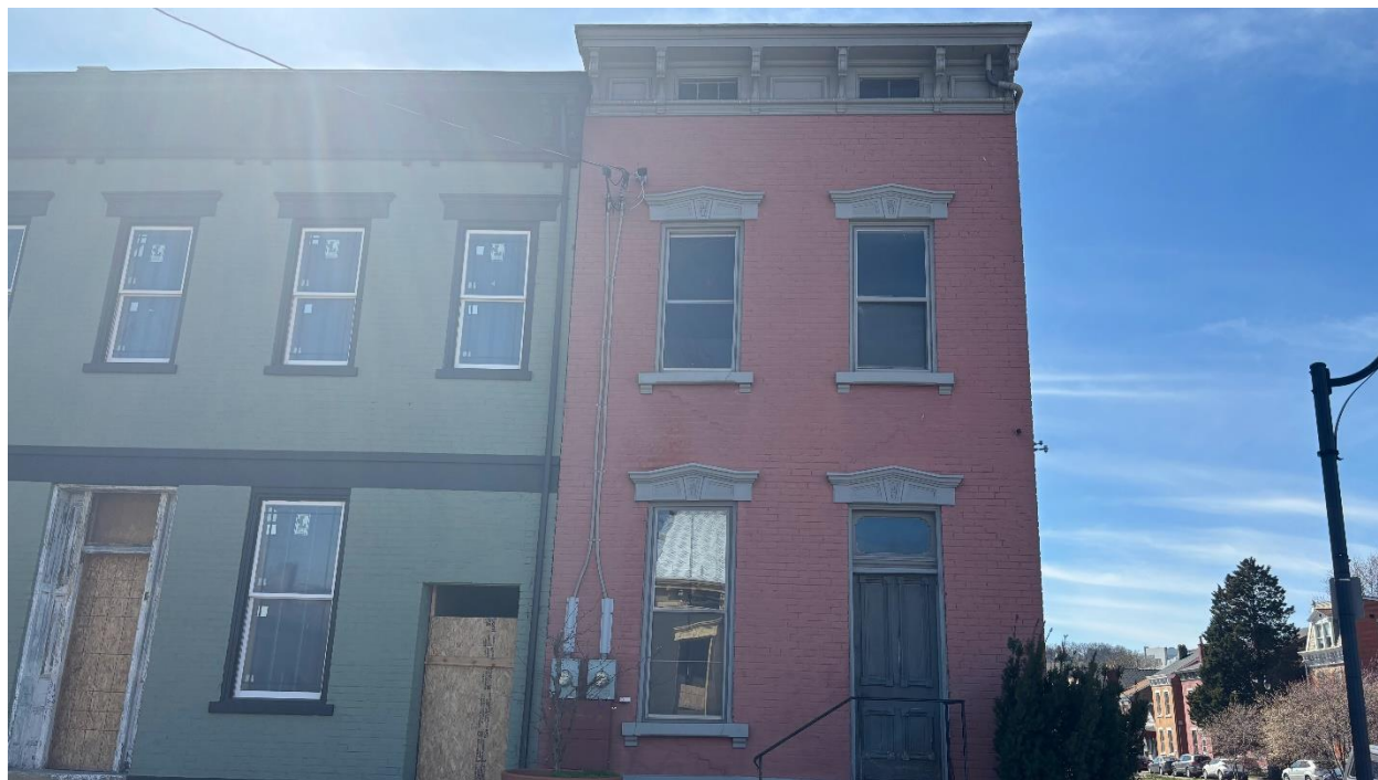
The Lubber House, Kenton County, Kentucky, east (front) facade
