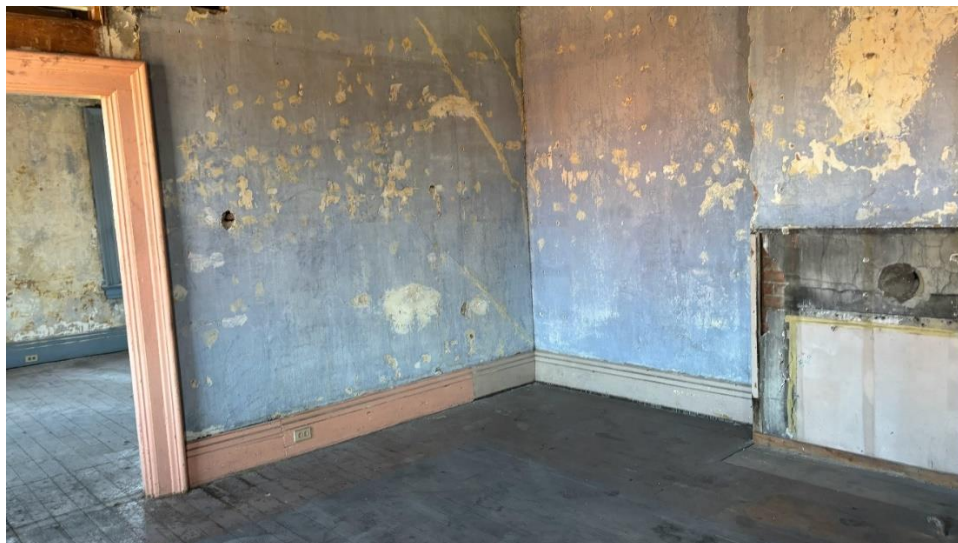
The Lubber House, Kenton County, Kentucky, second floor second room
