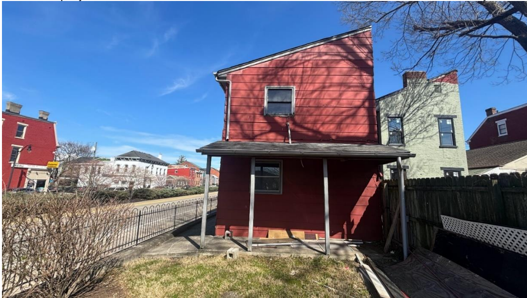
The Lubber House, Kenton County, Kentucky, west (rear) facade
