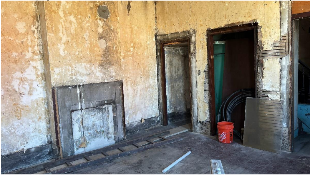
The Lubber House, Kenton County, Kentucky, first floor second room
