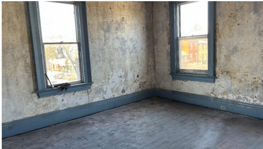
The Lubber House, Kenton County, Kentucky, second floor front room
