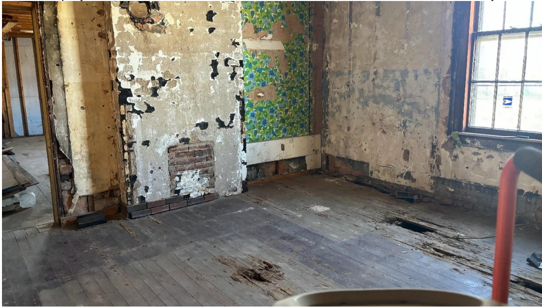
The Lubber House, Kenton County, Kentucky, first floor third room
