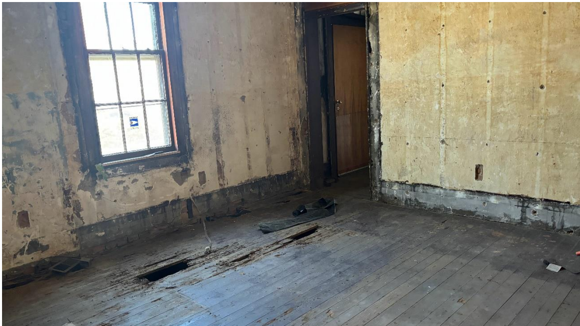
The Lubber House, Kenton County, Kentucky, first floor third room
