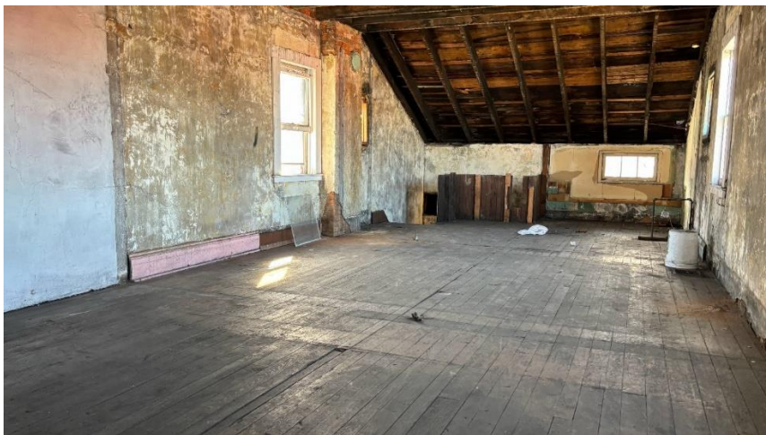
The Lubber House, Kenton County, Kentucky, third floor
