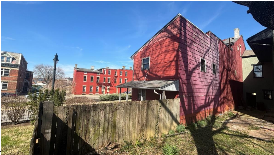
The Lubber House, Kenton County, Kentucky, south (side) facade
