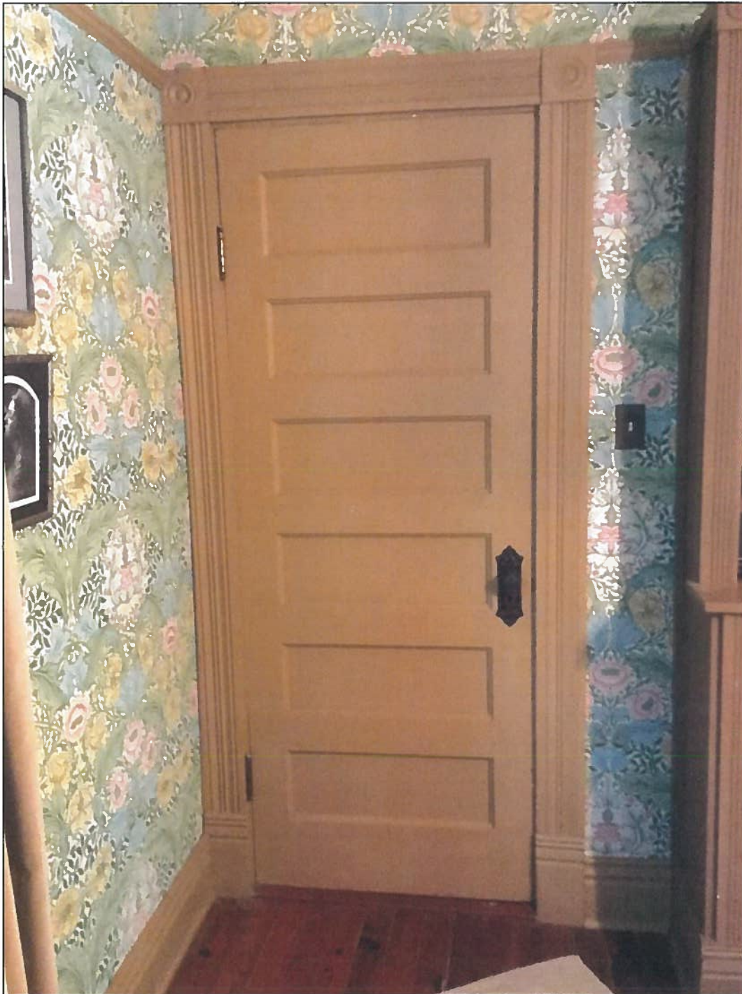
KY_Jefferson County_Harriet Griswold and Judge Samuel Bonner Kirby House_0020 Original six horizontal panel doors & hardware
