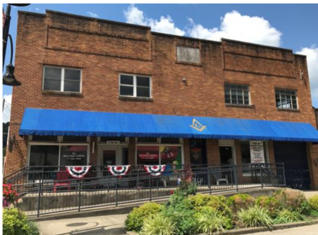
#36: Masonic Lodge Building
