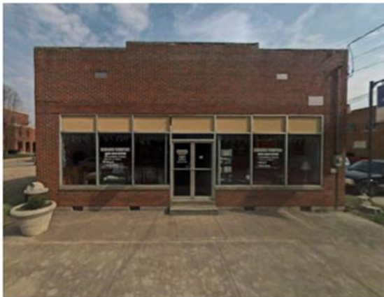
#7 Dunahoo Building prior to facade update.
