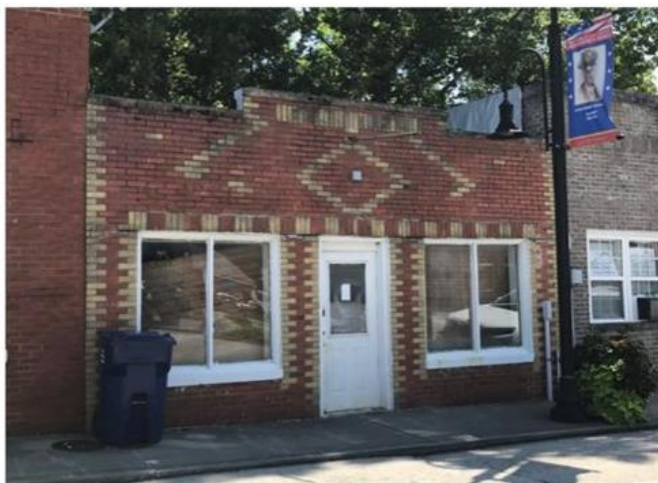
#17 Shuler Building, former Catholic Thrift Store
