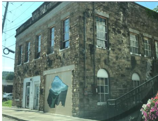
#51: Works Progress Administration Bldg.
