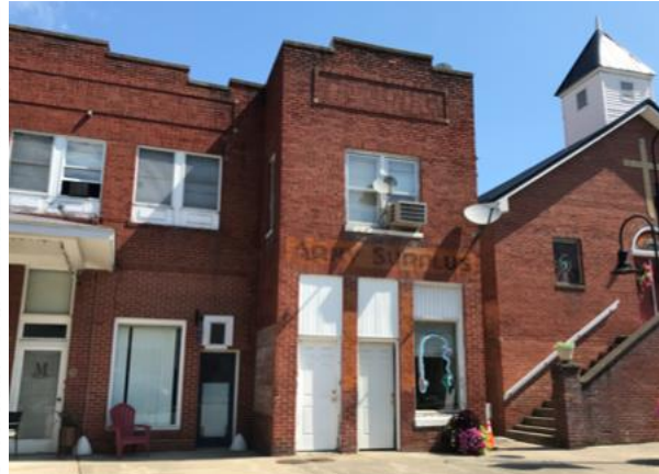
#25: Army Surplus Building
