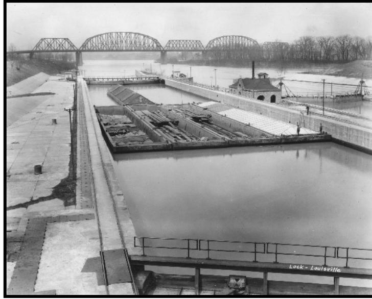
**Figure 4. 10** Lower part of locks, showing Dam 41 at Portland Canal and Lock, circa 1926.<sup>242</sup>
