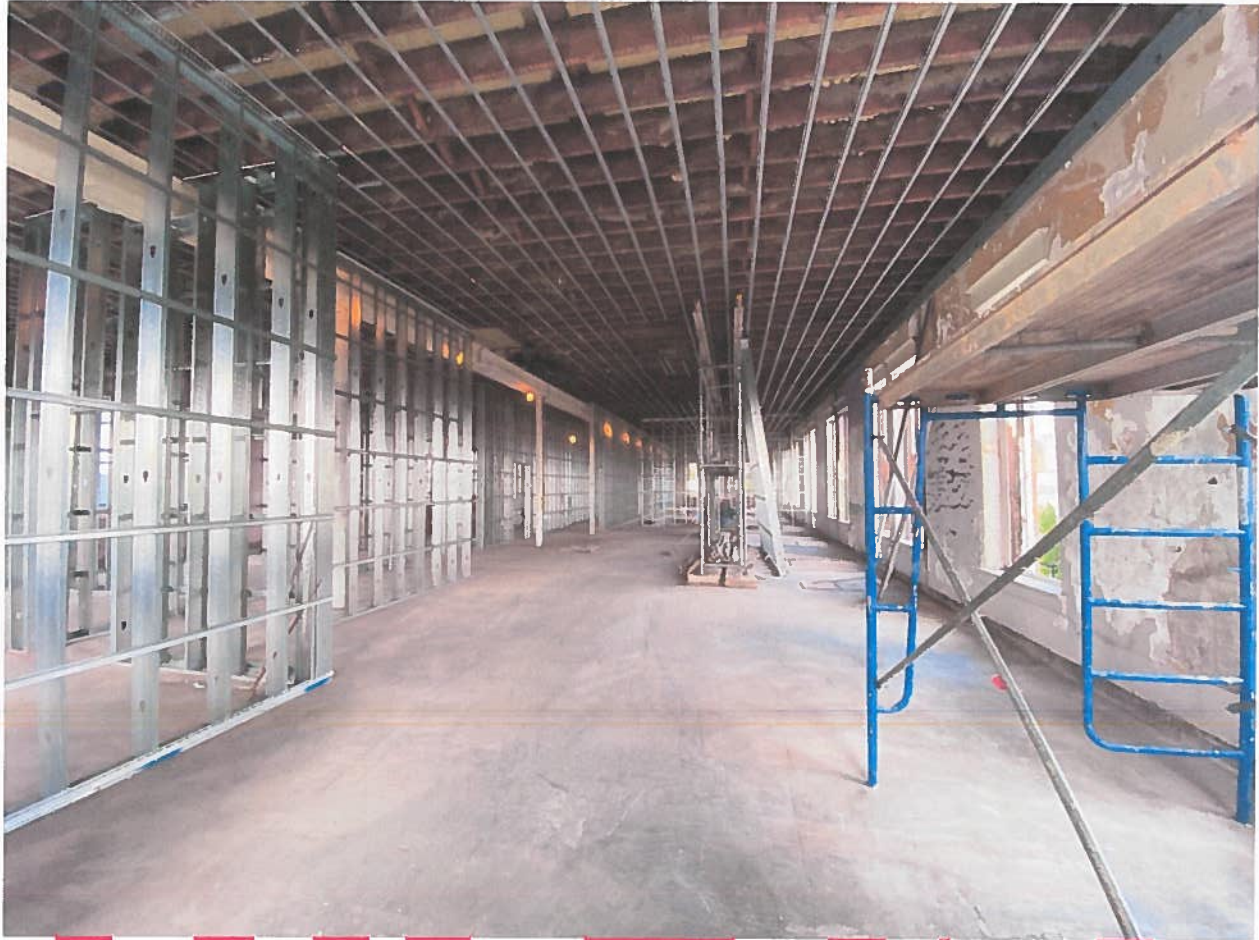
The front of the third floor, facing north along the east façade. The original heights have been restored and the non-historic partitions removed. 28 of 31.
