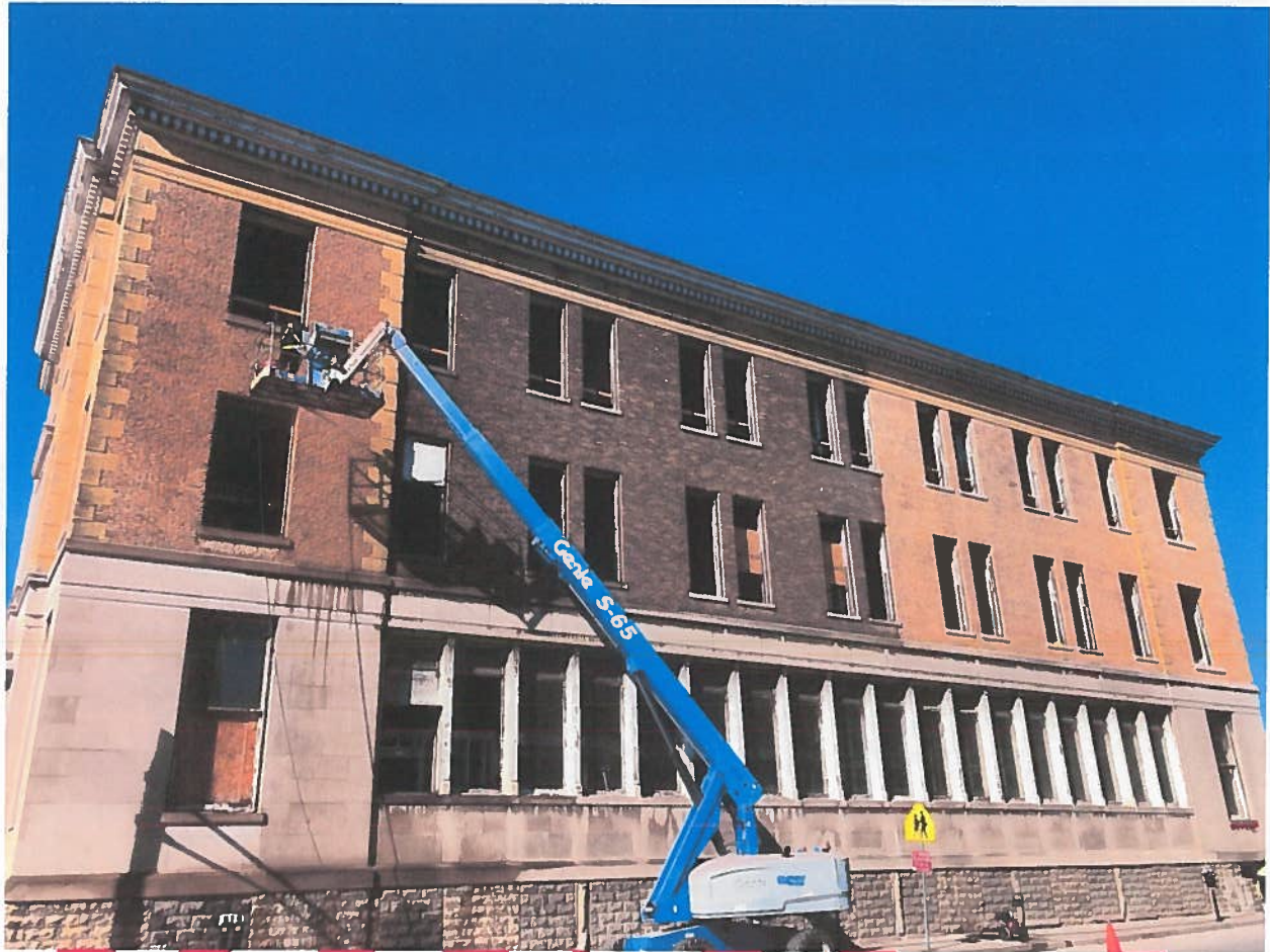
The east façade along South Brook Street in the process of being cleaned. The dark section has not yet been cleaned. The blond brick has been cleaned. 18 of 31.
