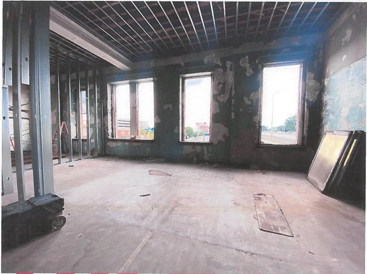
The front of the second floor, in the southwest corner, along the interstate, which is visible through the right window. Initial framing has begun with the non-historic partitions removed.
