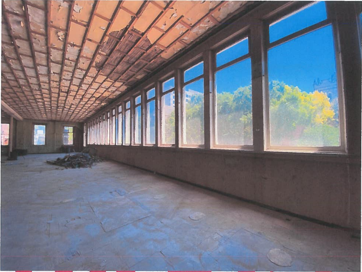
The infirmary area after demolition, facing north. The windows and the ceiling have been returned to full height.
