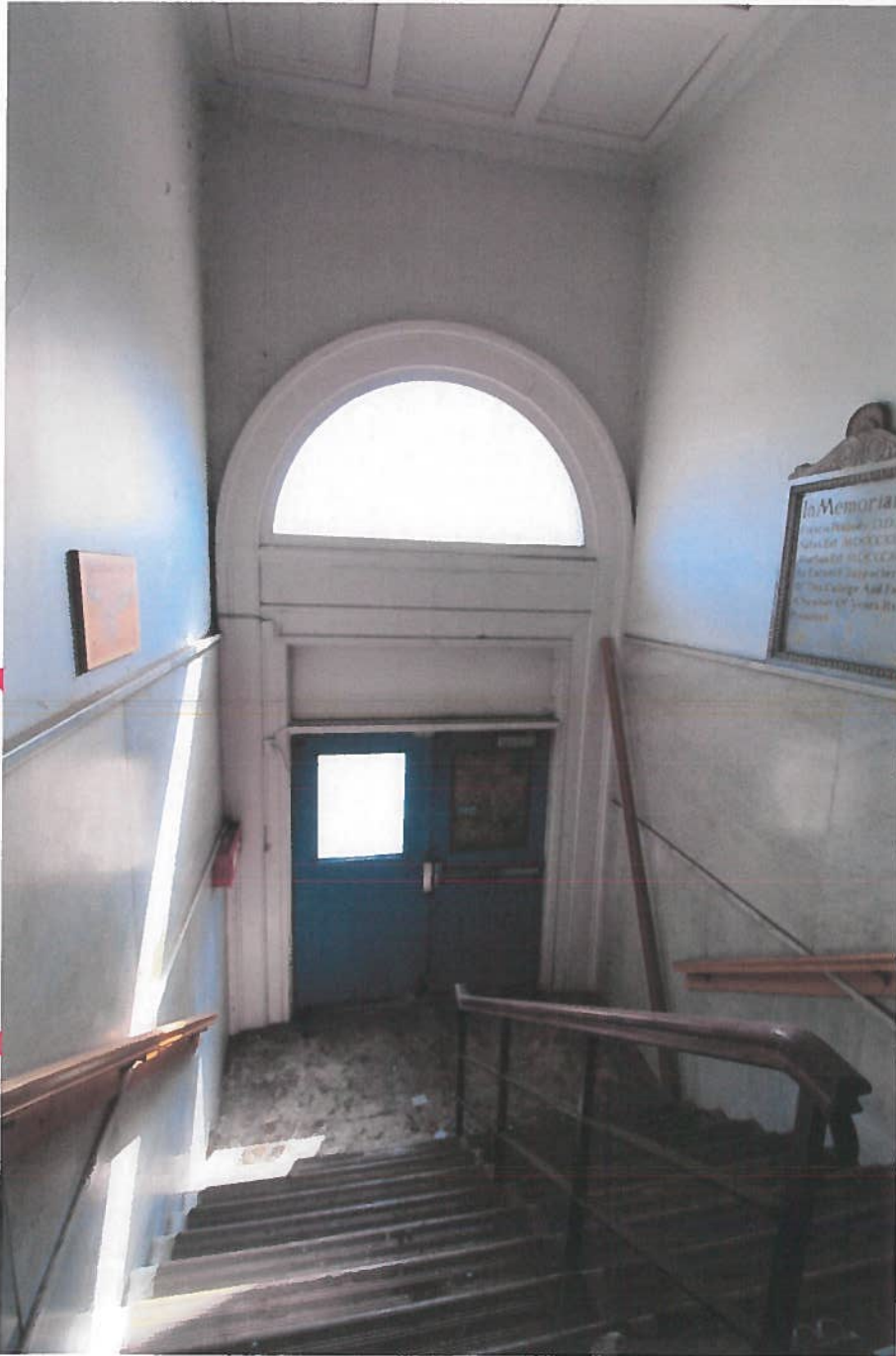
The front entrance, facing down the interior steps to the front doors. The doors are non-historic, but the arched window is original as well as all the interior materials and configuration. 6 of 31.
