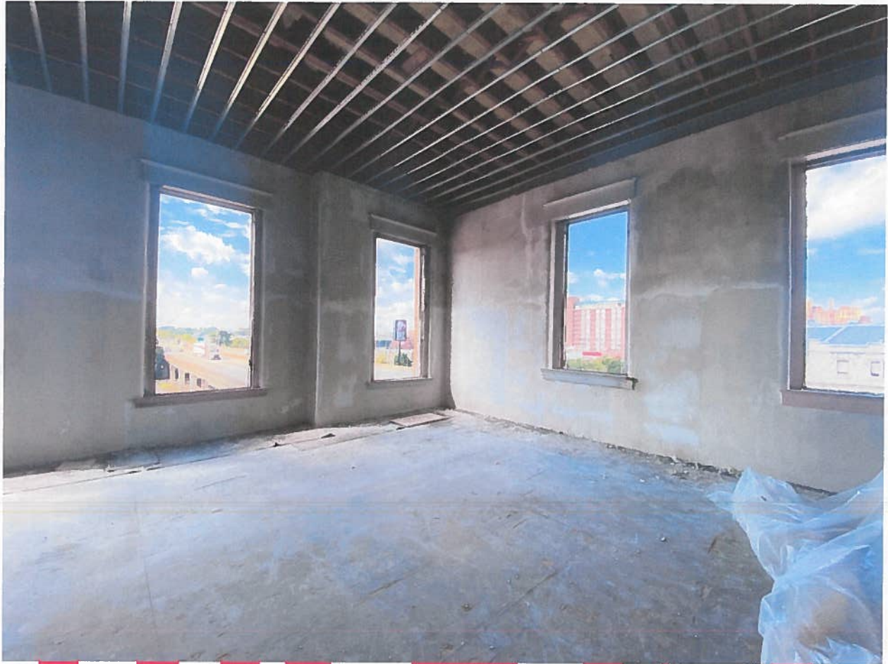
The southwest corner of the third floor, facing southwest. The plaster walls were all restored after shattering behind the furred out drywall. 29 of 31.
