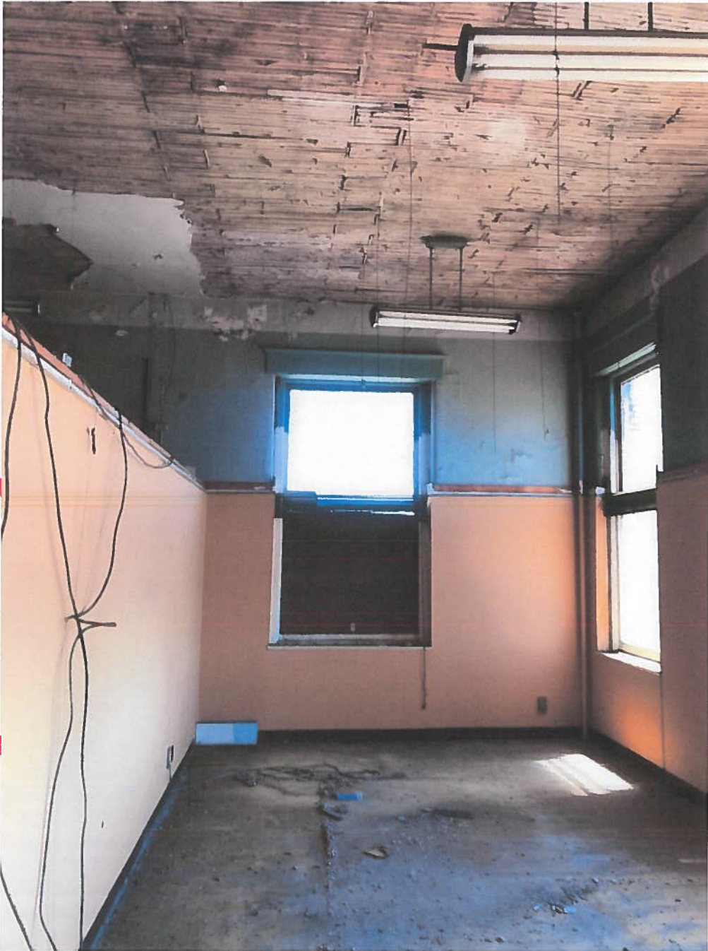
The southeast corner of the second floor, where the ceiling was removed to determine the extent of historic materials beneath. The original plaster ceiling was mostly removed when the ceiling height was lower significantly. The walls beneath the non-historic ceilings were furred out to run electrical, plumbing, and HVAC system components.
