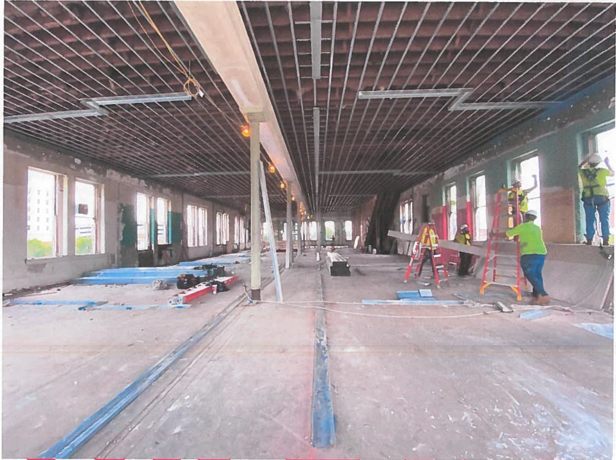
The second floor, facing south toward the front of the building. The non-historic partition walls were removed and the initial framing is beginning.
