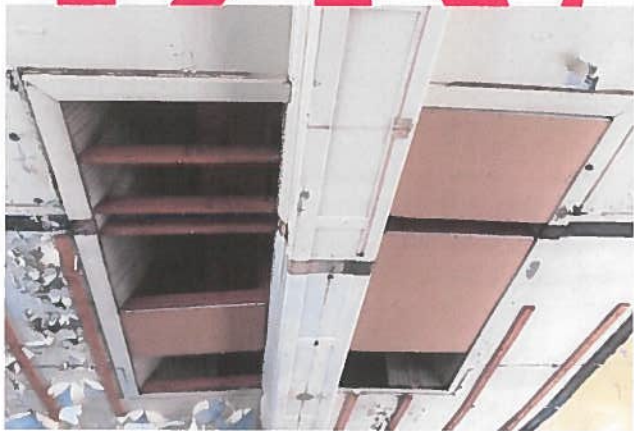
Skylight at the front of the third floor, which was located over the main structural beam of the building. The skylight provided light to an instruction lab below.
