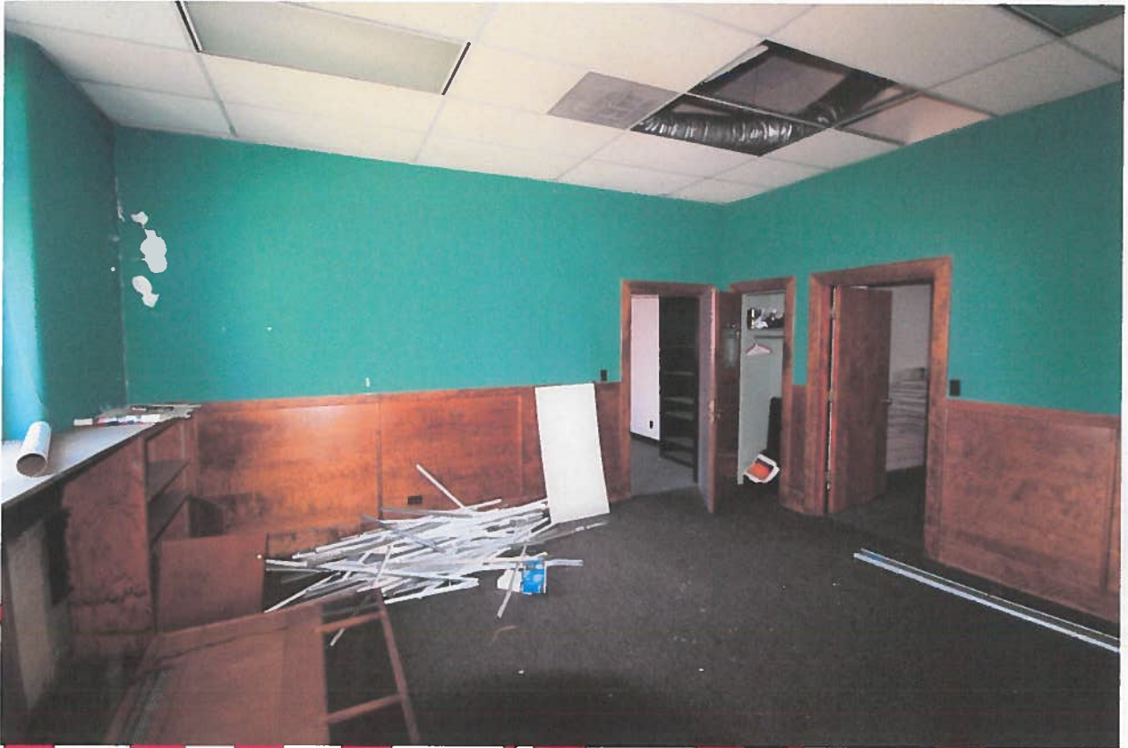
A corner office at the rear of the second floor, with windows that overlook Brook Street. The paneling and the ceiling are non-historic and were likely installed when the modern heaters were installed. 10 of 31.
