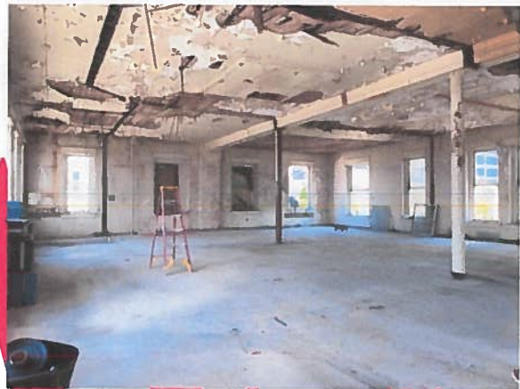
Existing columns and beam at the rear of the third floor.
