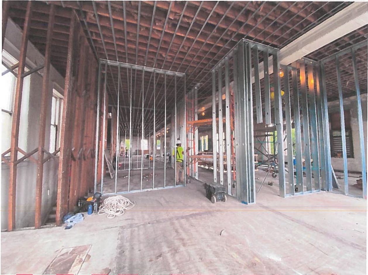
The front of the second floor, facing north toward the rear of the building. The initial unit framework has begun. The floors and ceilings have not been completed.
