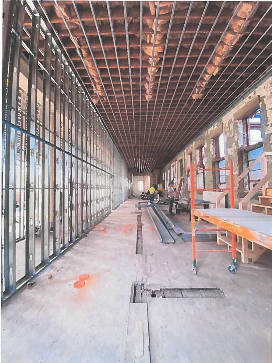
The first floor, facing south toward the front of the building. The initial framing has begun for the first floor corridor. The ceilings and floors have not been completed yet. 19 of 31.
