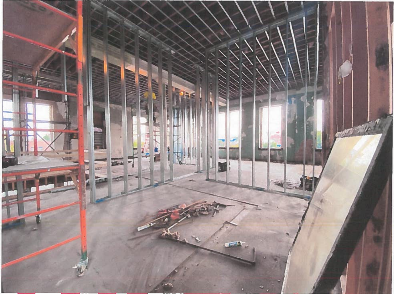
The middle of the second floor, facing southeast toward the front of the building. The initial framing has begun, which is restoring the full height of the spaces.
