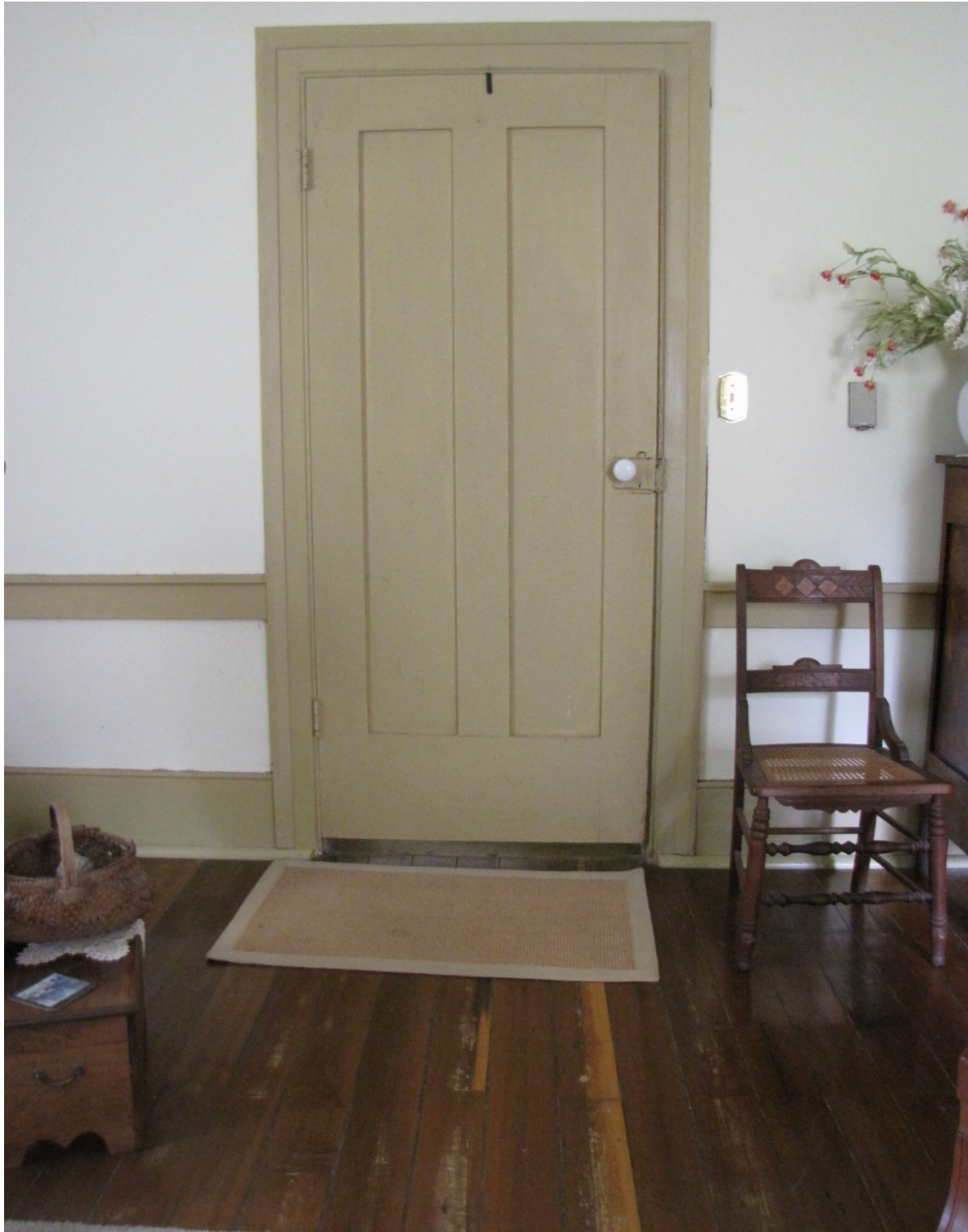
Interior door from downstairs south bay to entry hall; also showing the baseboard and chair rail of the south bay room, and the restored original poplar floors.
