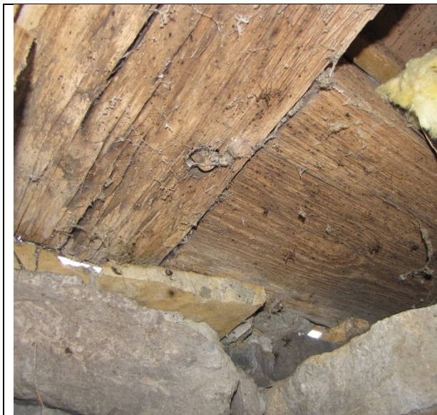
Sill timbers at corner, as seen from crawlspace in northwest corner of house.
