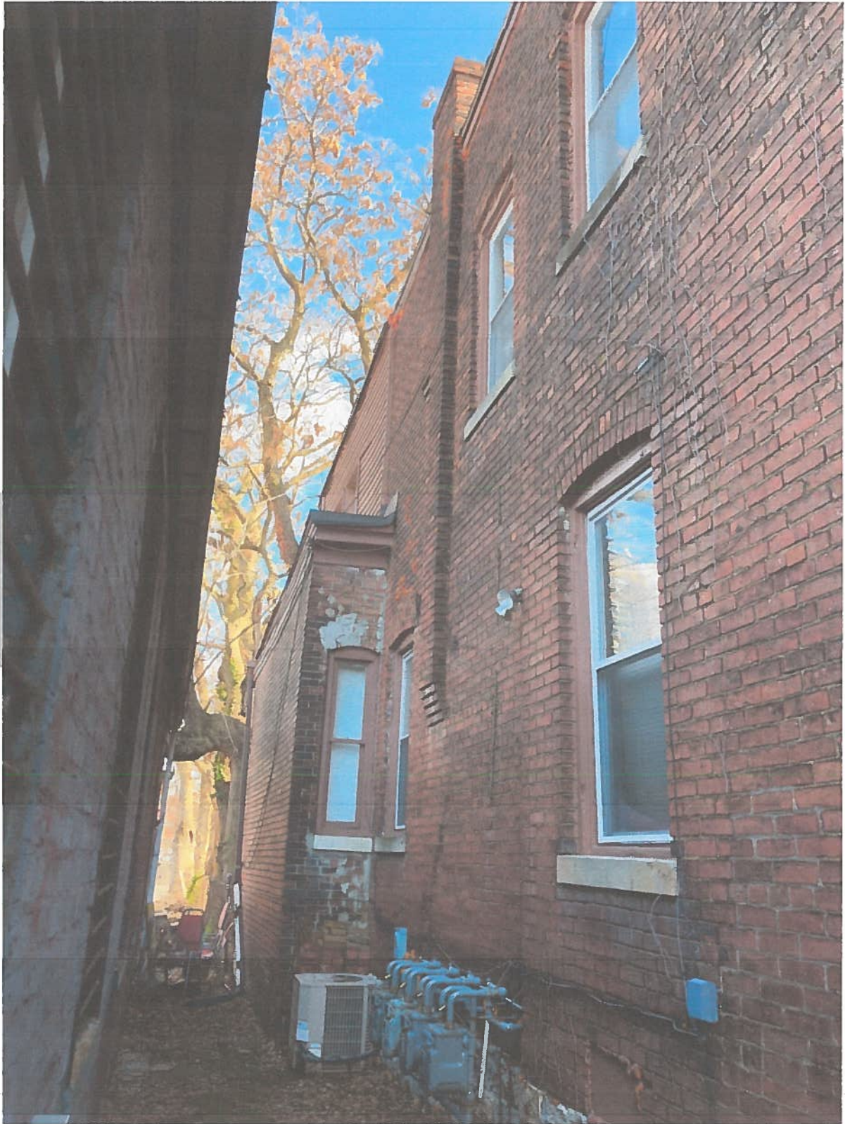
Photo 5: North Facing Side of Nugent House, Looking East
