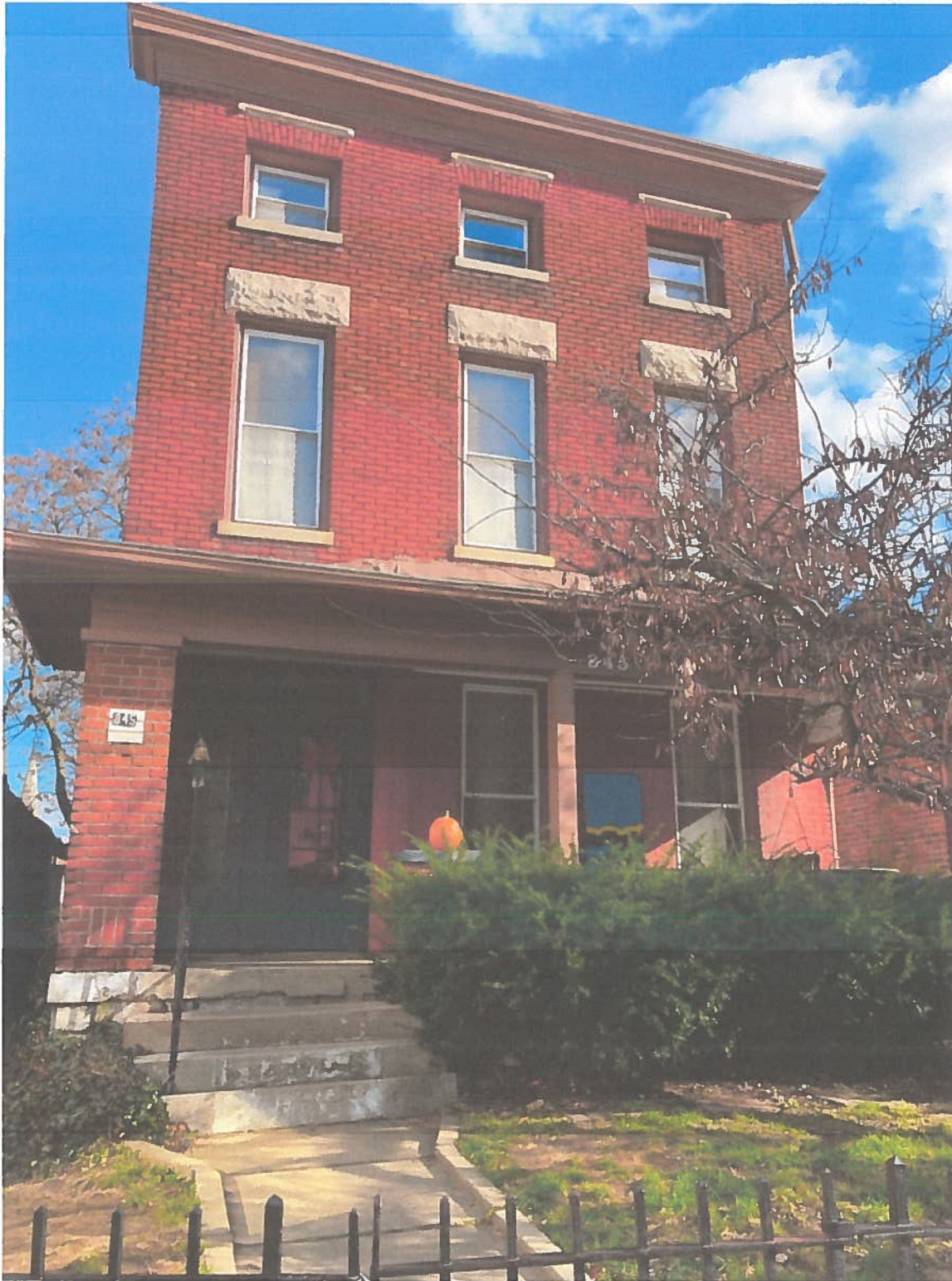
Photo 2: Nugent House Facade Facing S. 6 th Street, Looking East
