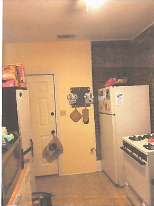
Kitchen, View of Door to Exit Stairs
