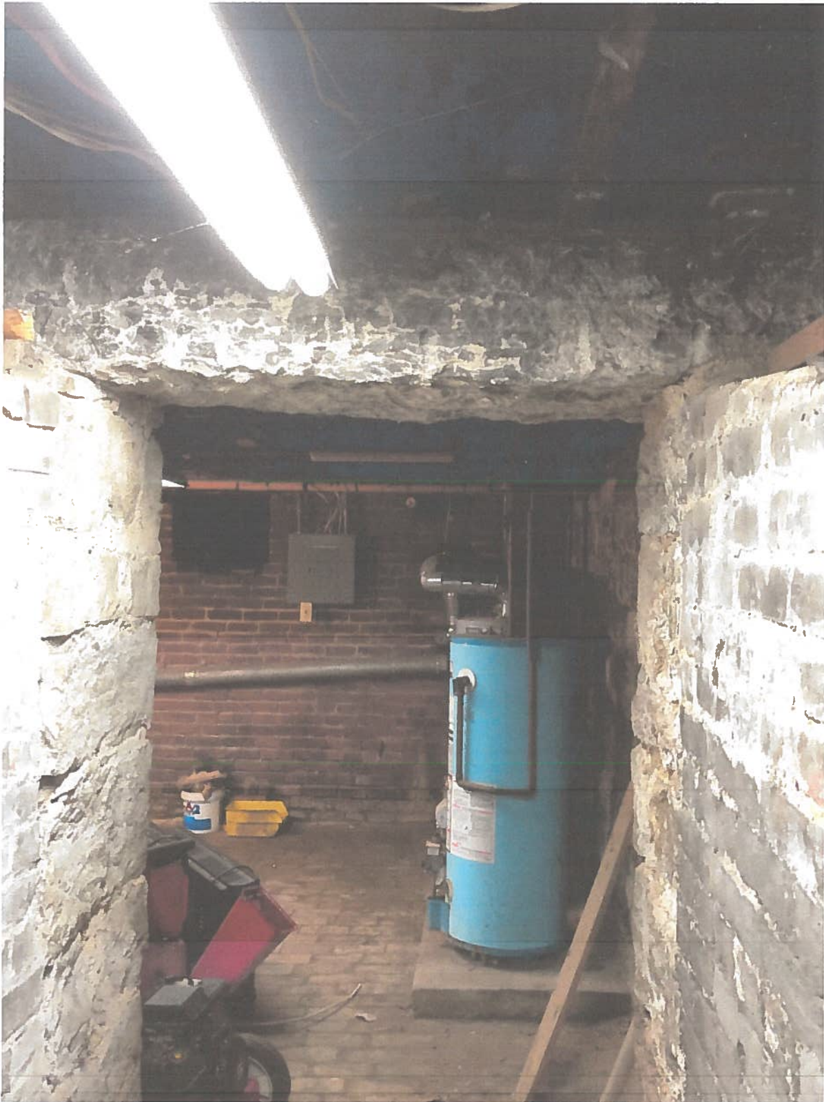
Photo 12: Basement Entrance, Looking West
