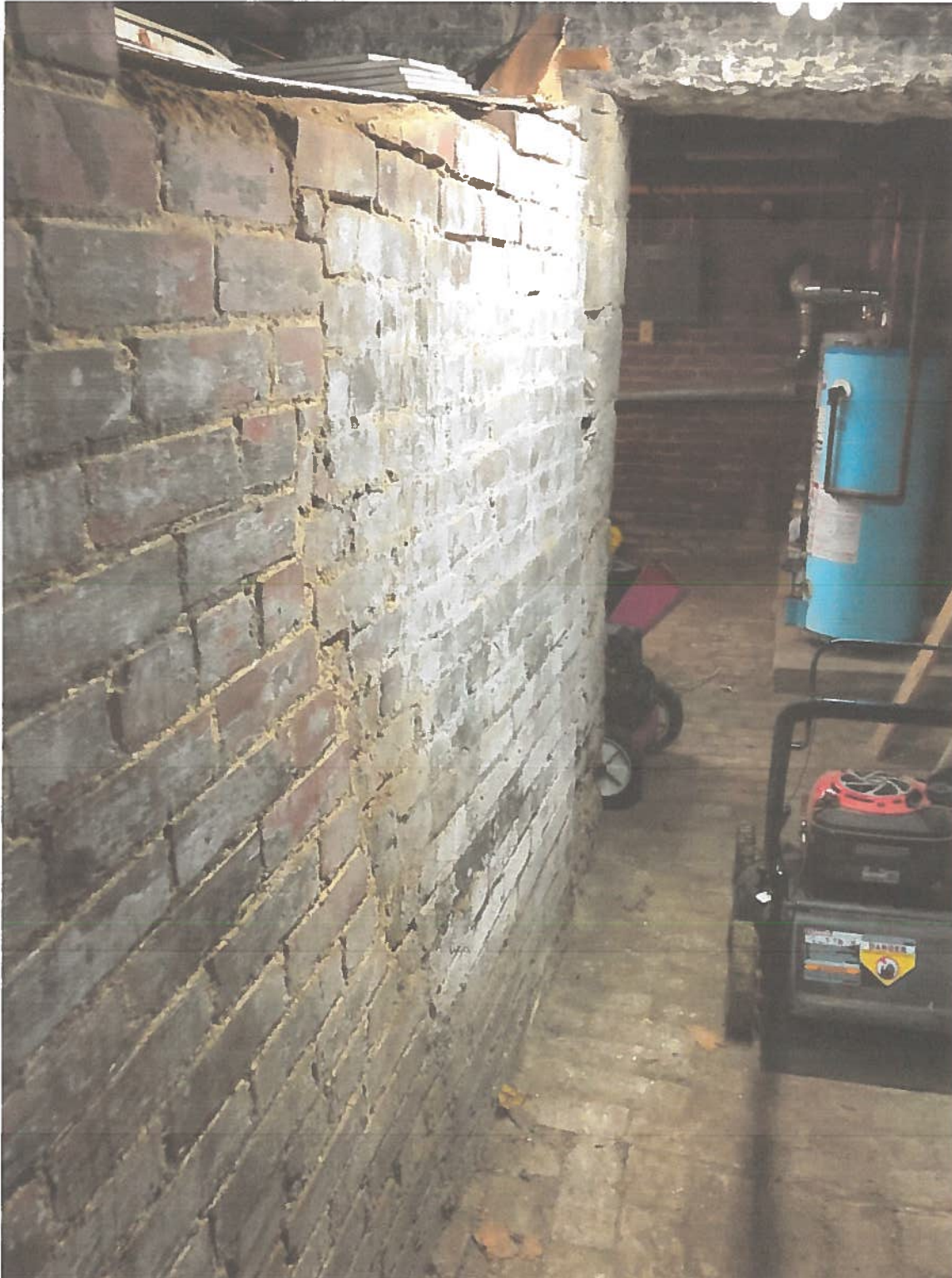
Photo 11: Basement Entrance, Looking West
