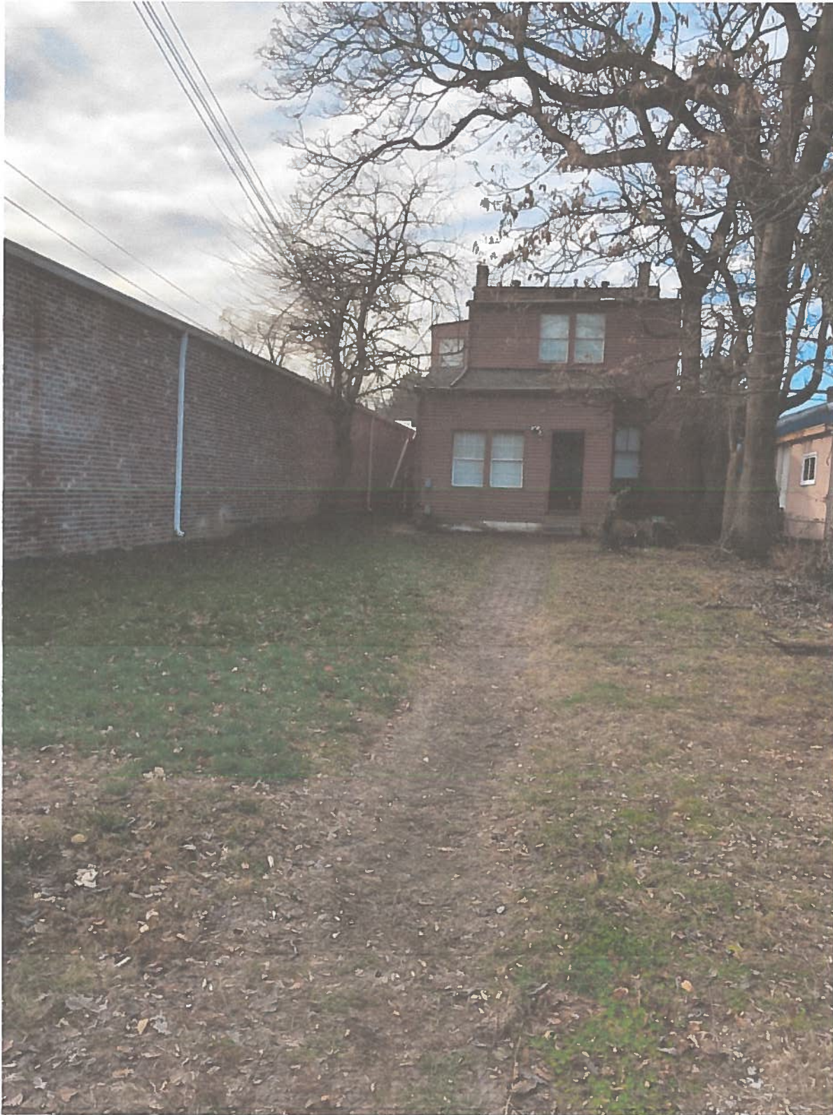
Photo 8: Rear of Nugent House, Looking West
