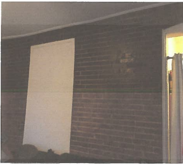
Original Exterior Brick Wall in Studio
