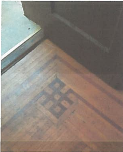
Detailed Inlay on First Floor
