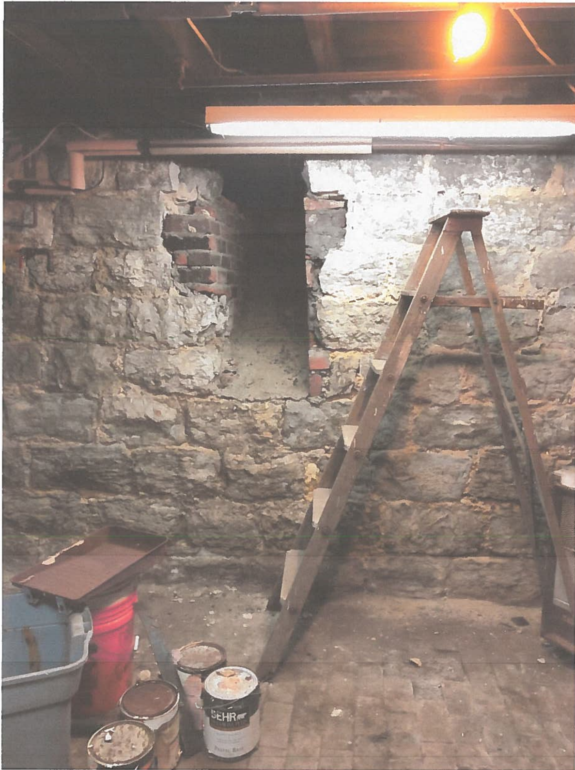
Photo 13: Basement, Looking South, View of Original Coal Shoot
