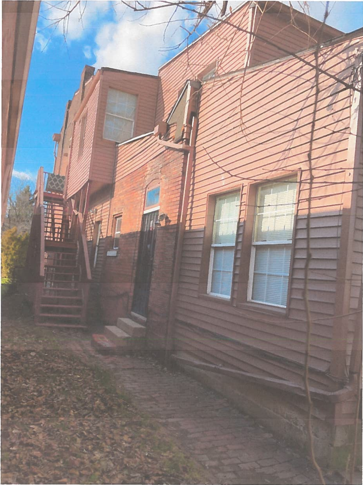
Photo 10: South Facing Side of Nugent House, Looking West
