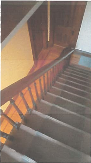
View from Third Floor, Looking Down to Second Floor
