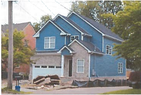
An example of infill construction. This house was constructed in 2019. 134 Goodrich Avenue (FAL-634, NRHP #394)
