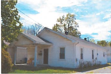
An example of one of four properties classified as early 20 th century vernacular. 198 Rosemont Garden(FAL-335, NRHP #99)
