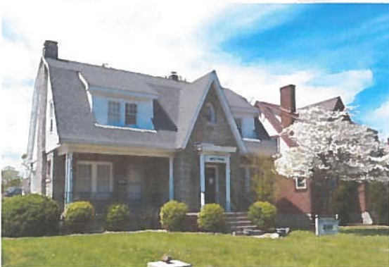
An example of a rooming house. 1739 Nicholasville Road (FAL-238, NRHP # 2)
