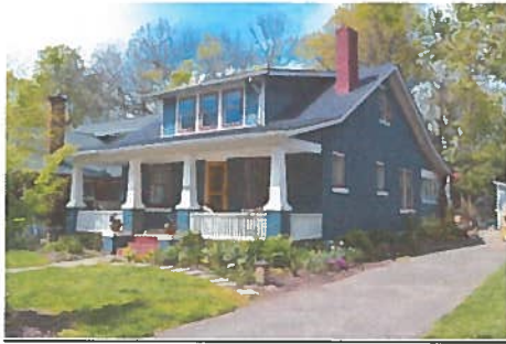
An example of a bungalow in the Craftsman style. 157 Suburban Court (FAL-264, NRHP #29)
