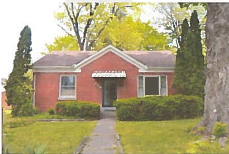
An example of a mid-20 th century vernacular resource. 159 Wabash Drive (FAL-469, NRHP # 233)
