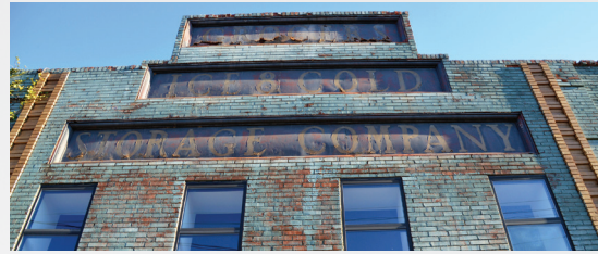
1906 Grocers Ice and Cold Storage Company building
