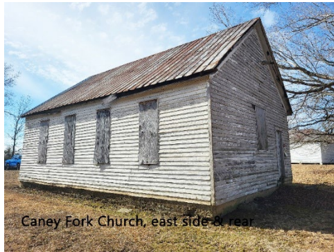
Southeast and Northeast (back) sides
