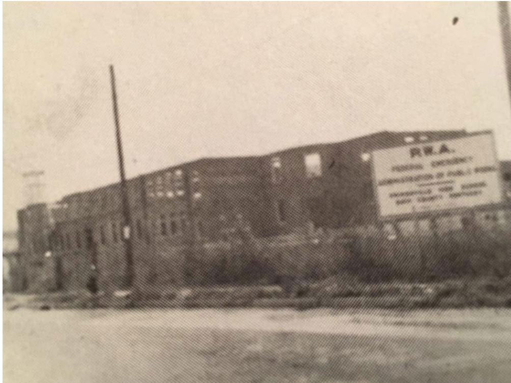
Bath County High School under construction, ca. 1939. Note PWA sign to the right.
