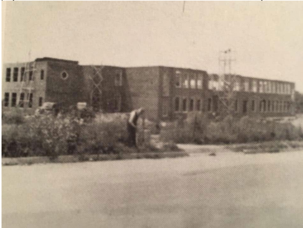
Bath County High School under construction, ca. 1939.
