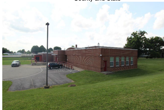
South end of east facade
