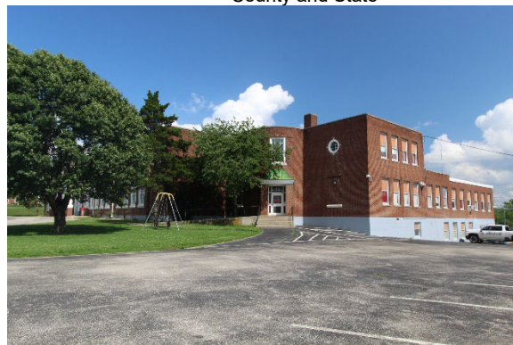
North end of west facade
