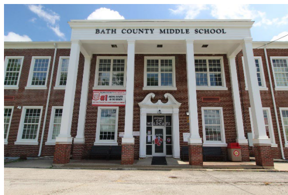
Detail of entryway and portico
