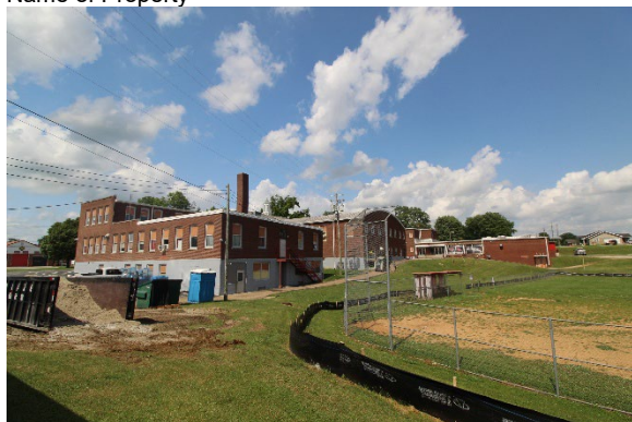
South end of west facade
