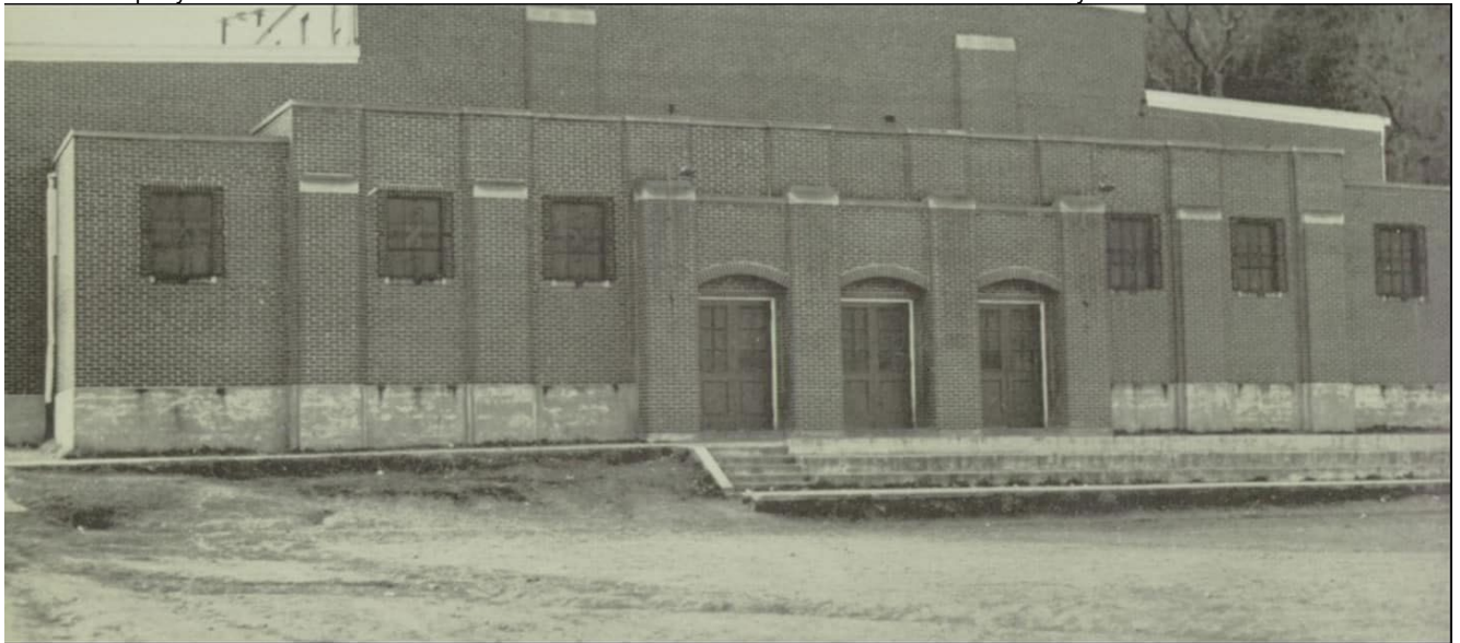
View of the PWA Gymnasium, ca. 1950. Note that the entryway sits much lower than the rest of the building to accommodate it being built into the bank. The outer doors led to steps to the gym while the center door led to a ticket booth.
