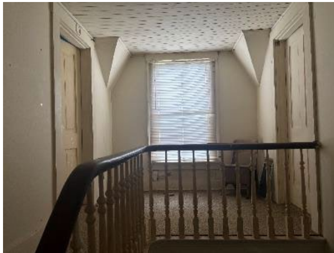
Second floor landing with original handrail and balustrade, Beadboard ceiling, wood doors and wood trim
