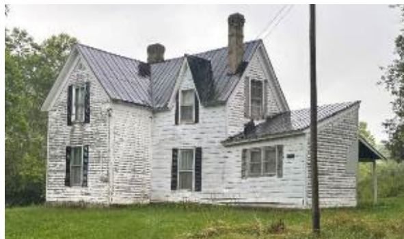
North and West Elevations
