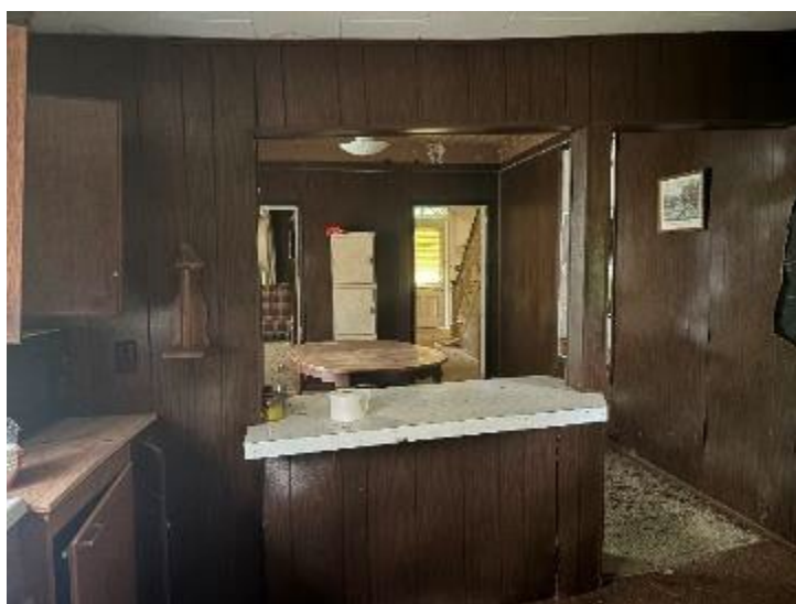
Kitchen, looking east. Located in rear addition
