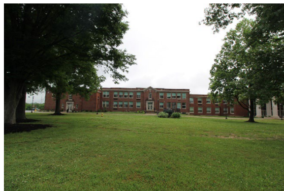
West Façade-1939 Building
