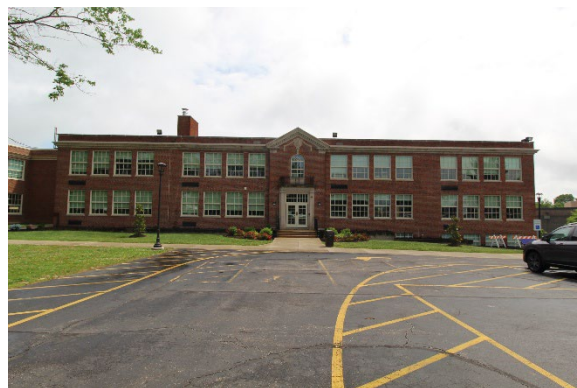
West Façade-1948 Building
