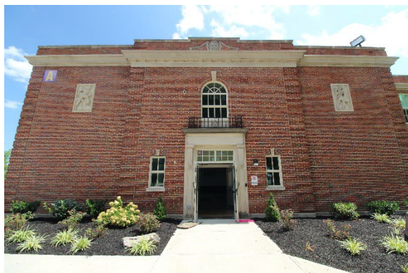
West Façade-PWA Gym
