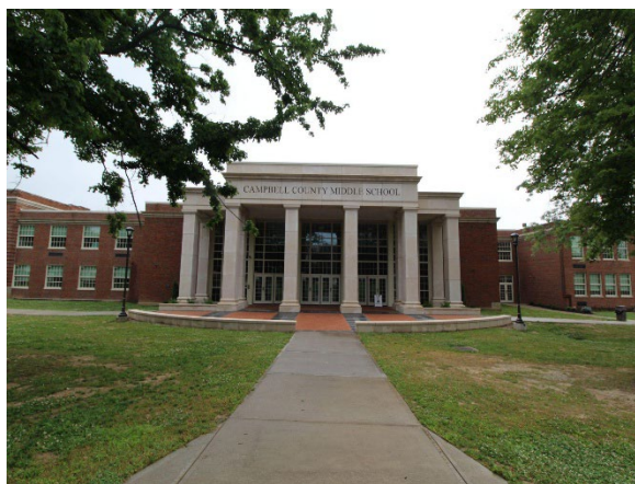
West Façade-Central Entryway
