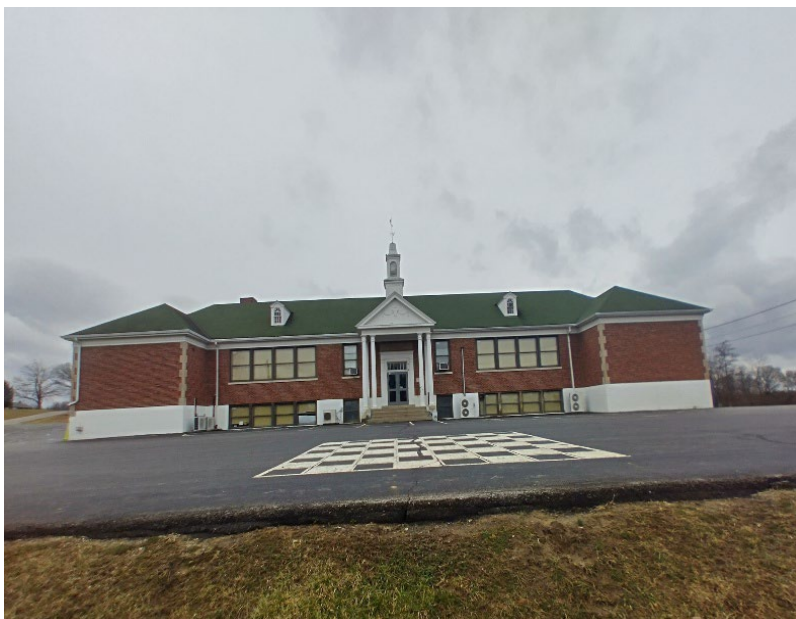
Figure 5. Historic Façade, oriented east.
