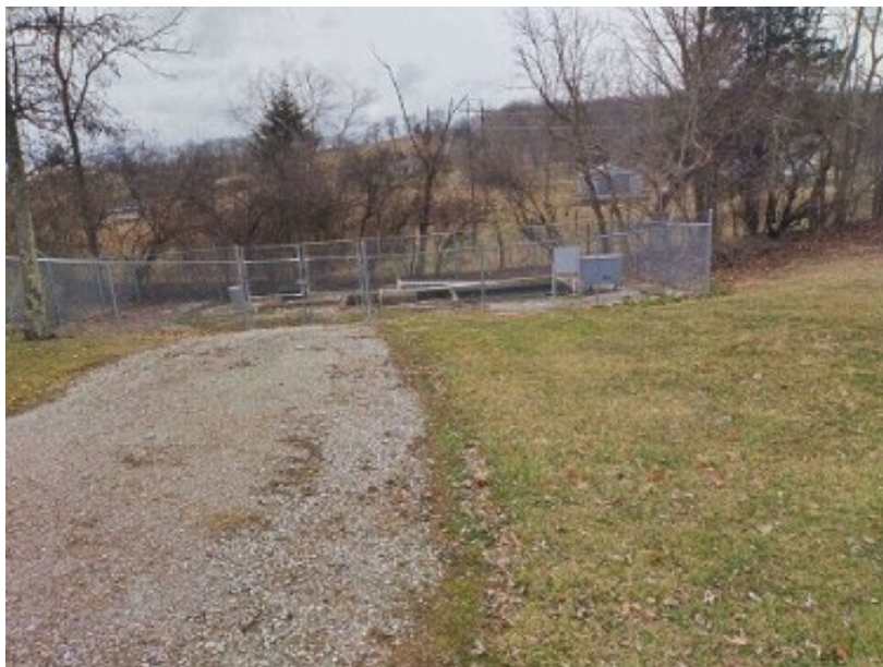
Resource D, Water Treatment Plant
