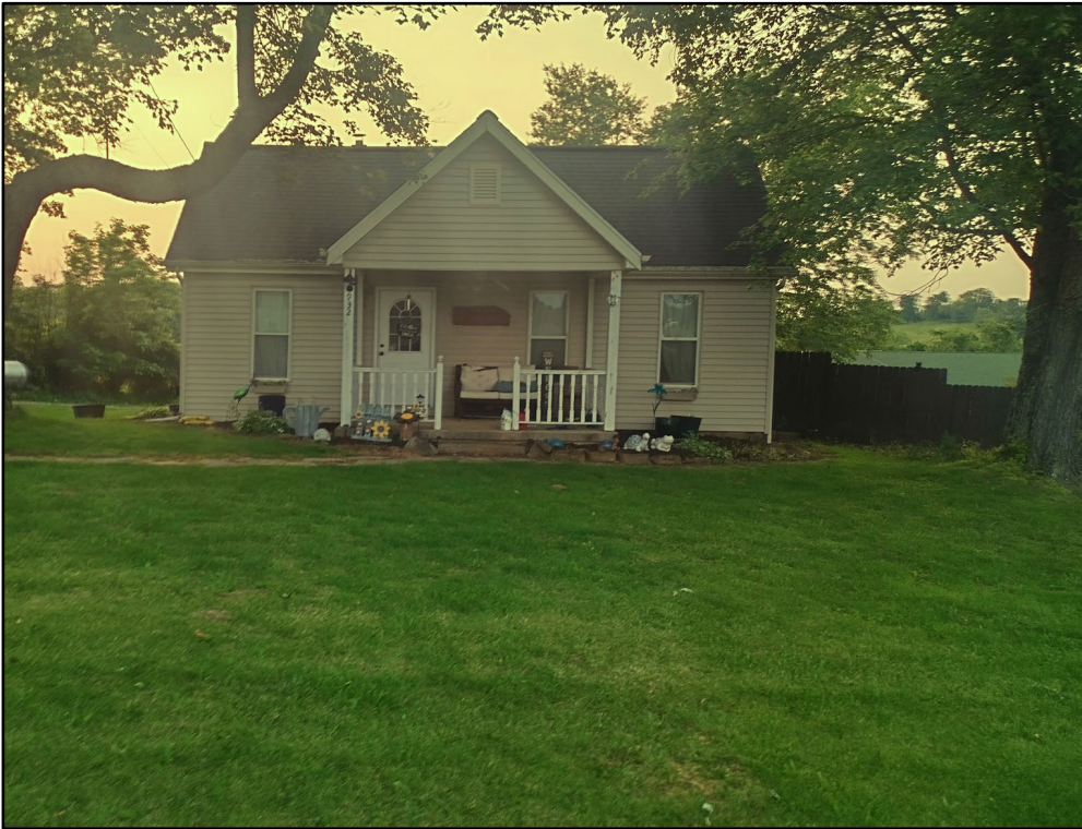
Figure 6. The Principal's/Janitor's House (CP 556). 2025
